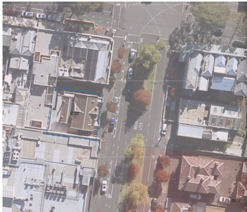
Figure 2: Aerial view of the La Mama Carlton Courthouse (delineated with the dashed blue line). The former Carlton Police Station (shaded) is visible diagonally opposite in Drummond Street. The two buildings are evidence of the enforcement of law and order in Carlton in earlier years. Source of image: Vicplan
