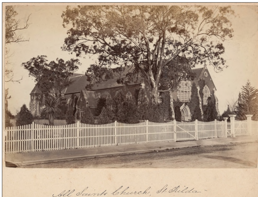
Figure 2 Undated image of All Saints Church, with timber picket fence evident. Image Source: SLV.
