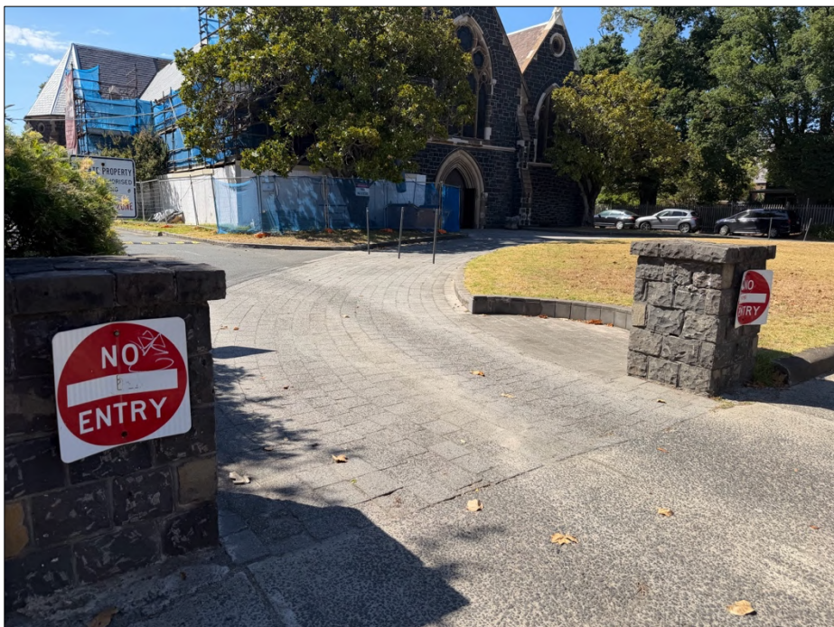
Figure 4 Bluestone piers to the north driveway entrance.
