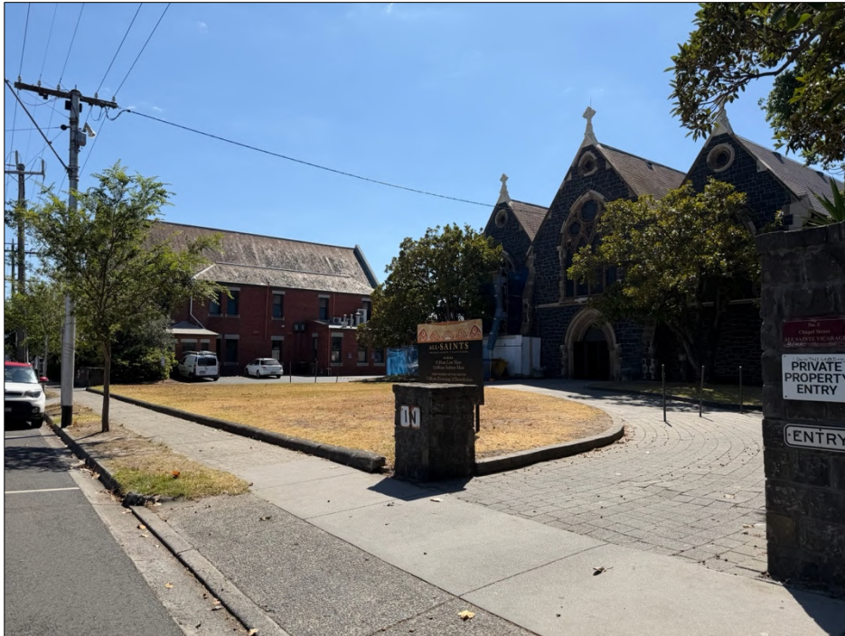
Figure 5 View of All Saints Church, including the bluestone piers at the southern end of the boundary.
