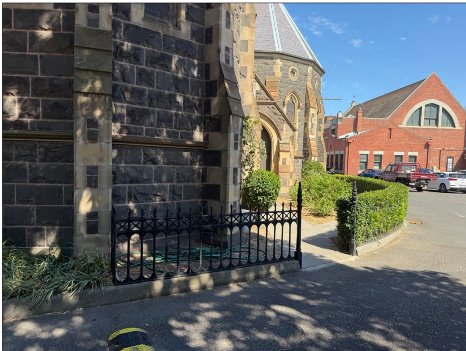
Figure 8 Metal picket fence at the rear of the church.
