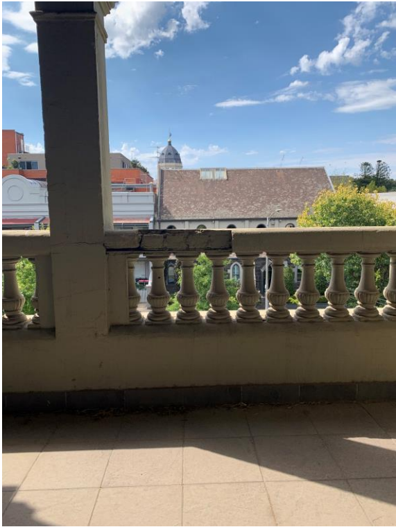
Figure 2 Modern tiling to the second floor balcony
