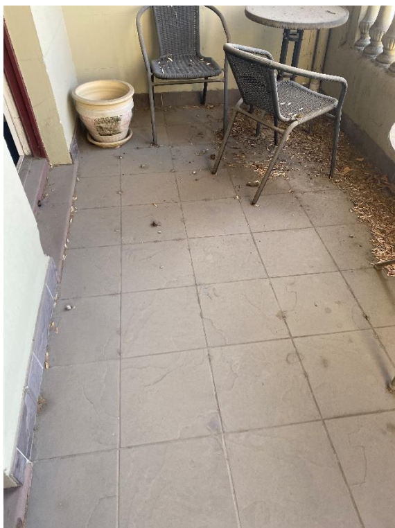
Figure 1 Modern tiling to the first floor balcony Source: Stoll Architecture
