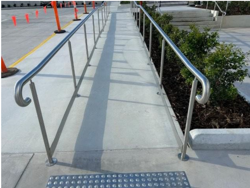
STAINLESS STEEL HANDRAILS WITH KERB RAILS
