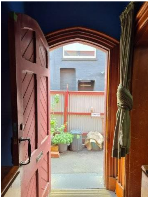
EXISTING TIMBER DOOR & ARCHITRAVE
