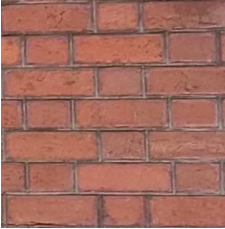
EXISTING FACE BRICKWORK: RED MORTAR FINISH: RED
