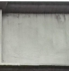
EXISTING FACE STONE WALL & TRIMS
