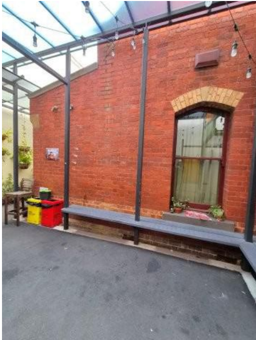
EXISTING BRICKWORK FINISH PATTERN
