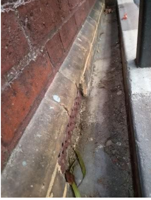
PHOTO 11 - CONCRETE VENTILATION CHANNEL
