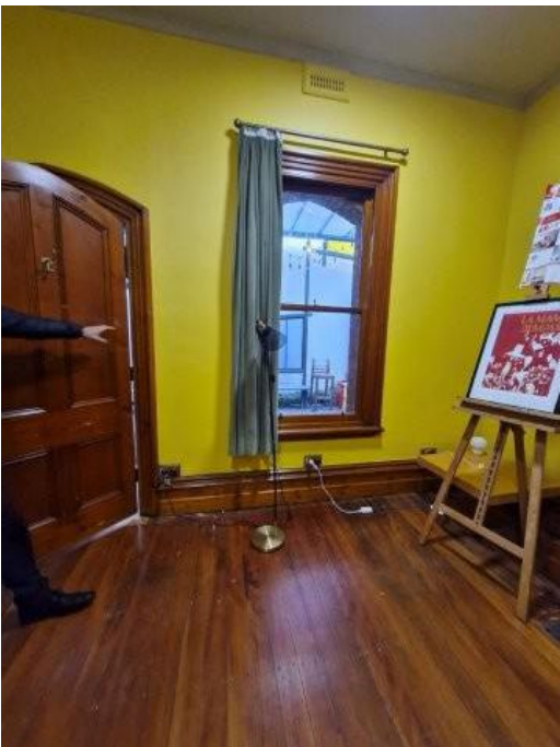
TIMBER ARCHITRAVE & SKIRTING IN DRESSING ROOM
