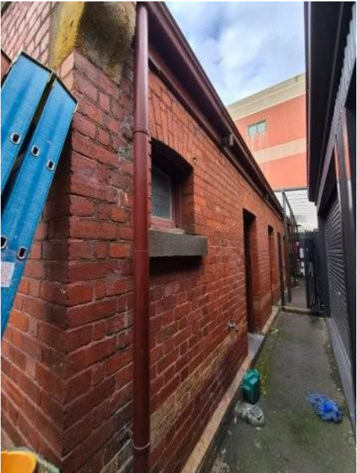
PHOTO 07 - ENTRY TO WC
