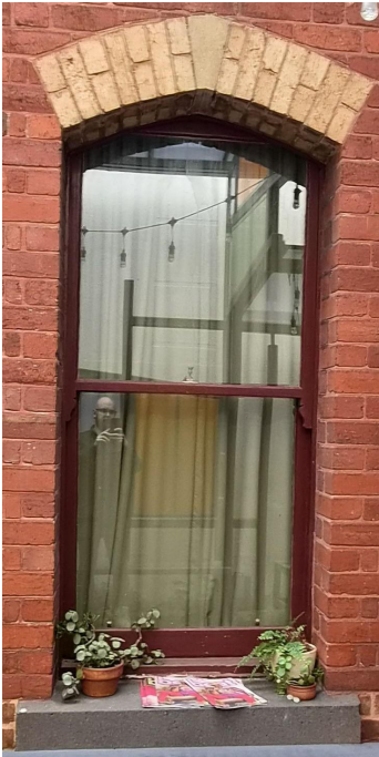
TIMBER FRAMED WINDOWS ,CONCRETE SILL & ARCHED BRICKWORK
