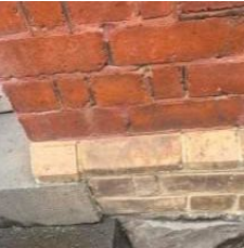
EXISTING PLINTH BRICKWORK: LIMESTONE MORTAR FINISH: LIMESTONE
