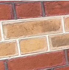
EXISTING FACE BRICKWORK: LIMESTONE MORTAR FINISH: LIMESTONE
