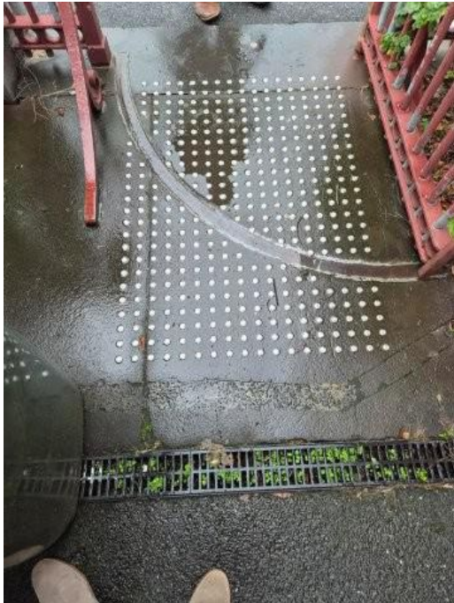
EXISTING STEEL ARC EMBEDDED INTO STONE PAVING
