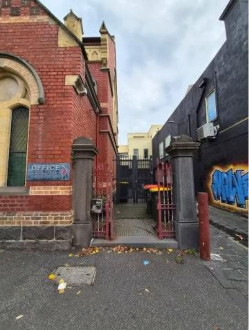
PHOTO 02 - PICKET FENCE & SECURITY GATE
