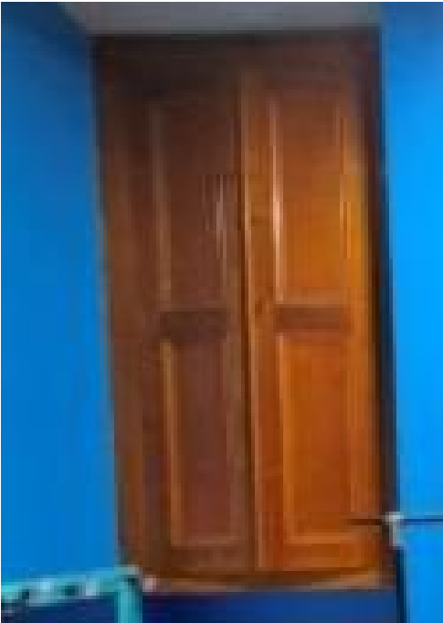
EXISTING CABINET IN FOYER
