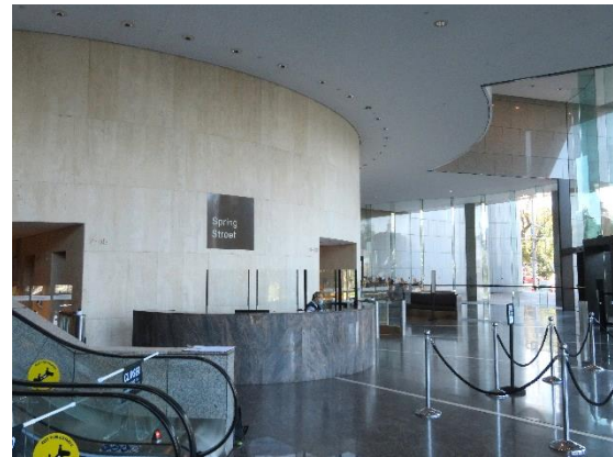
Figure 9 Security control point and expressed, travertine-clad core
