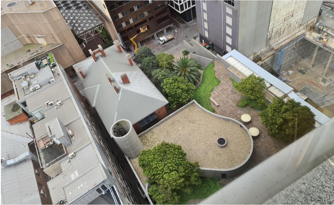
Figure 64 View of northern plazas and Milton House from Tower Level 15
