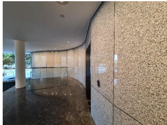
Figure 17 Curved baffle wall at the west end (rear) of the Ground level foyer
