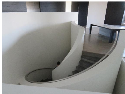
Figure 29 Curved internal staircase at Level 28
