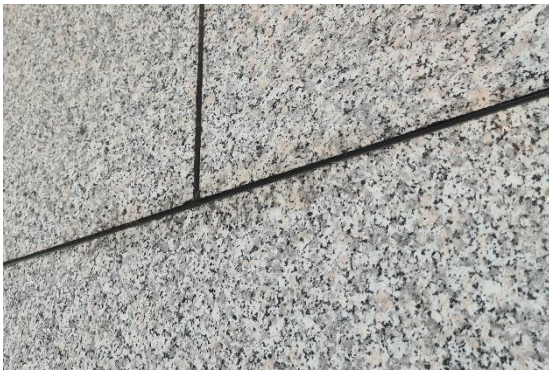
Figure 41 Grey granite wall cladding
