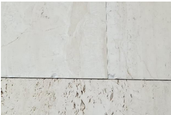
Figure 43 Unfilled travertine wall panels
