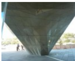
Building pier in main external plaza
