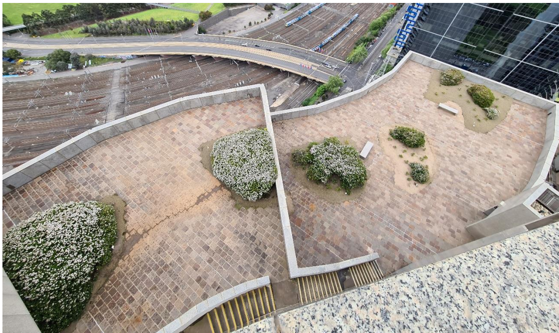
Figure 34 Roof plazas at Levels 27-28, as viewed from the roof of the service core
