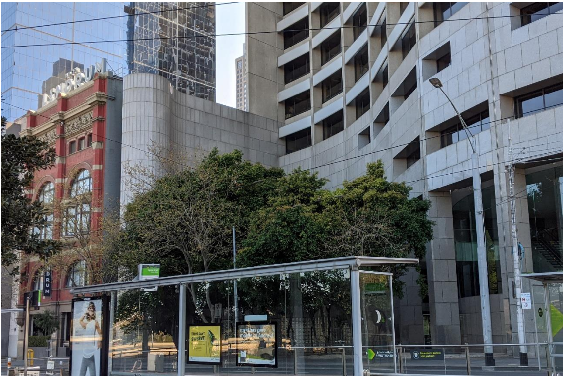
Figure 53 Flinders Street setback, showing the west screen wall as executed to match the height of the Hotel Lindrum, and the group of trees within the plaza which were established to meet planning and engineering requirements for wind protection in this corner
