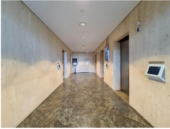
Figure 20 Ground level lift lobby
