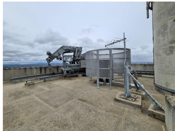
Figure 38 Jib crane and other equipment on service core roof
