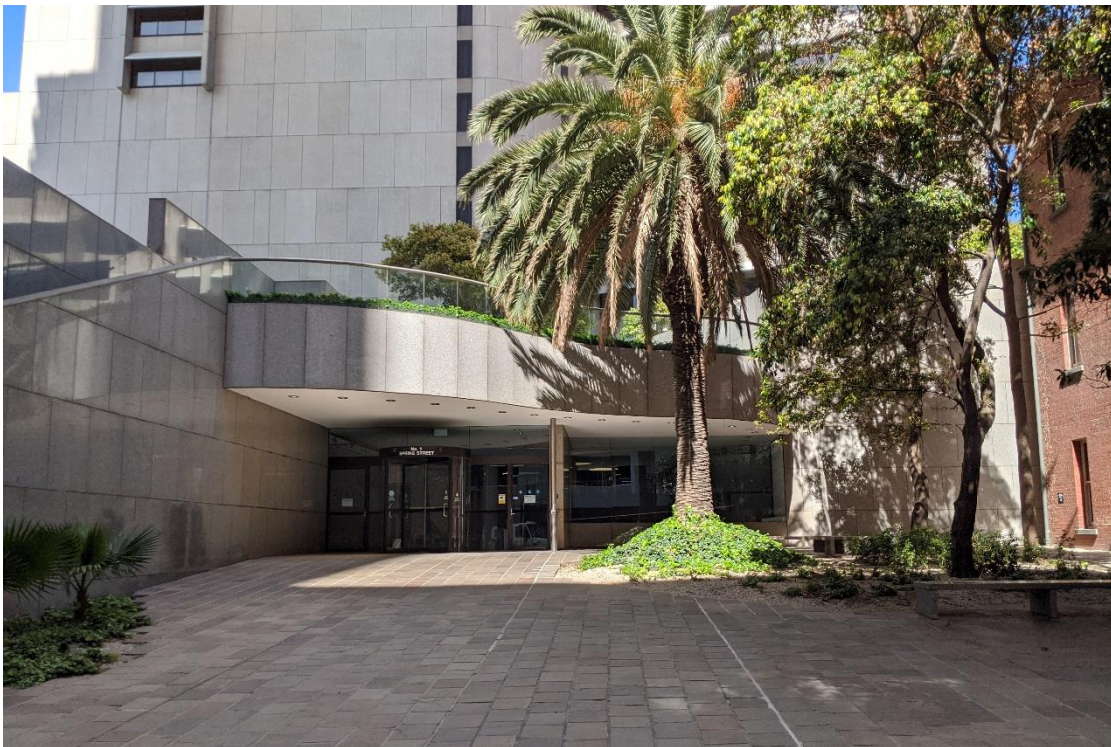
Figure 65 View south from Flinders Lane across the northern plaza to the level 2 concourse entry, with the level 3 roof garden balustrade and the tower's service elevation in background
