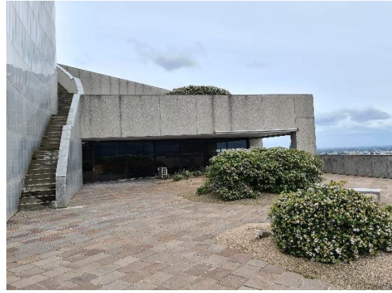
Figure 36 View of terraced roof levels from Level 27
