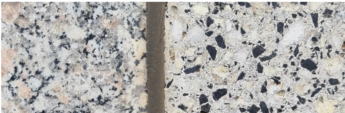
Figure 45 Comparison of natural grey granite cladding (left) and reconstructed granite precast (right)
