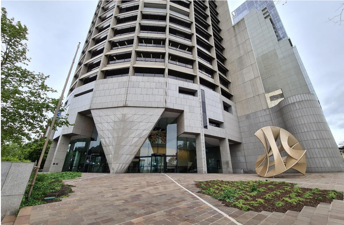
Figure 52 Spring Street plaza, showing the stepped arrangement of the north end wall
