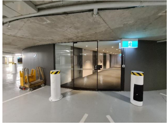
Figure 21 P4 car park lift lobby
