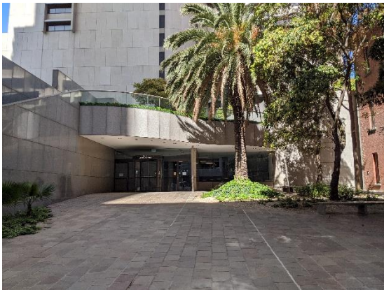
Figure 14 North plaza and entry from Flinders Lane
