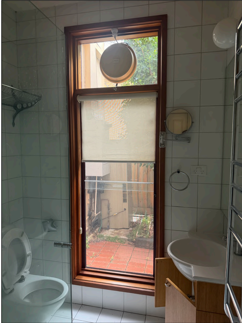
Figure 4 Altered window at ground level within the rear wing.
