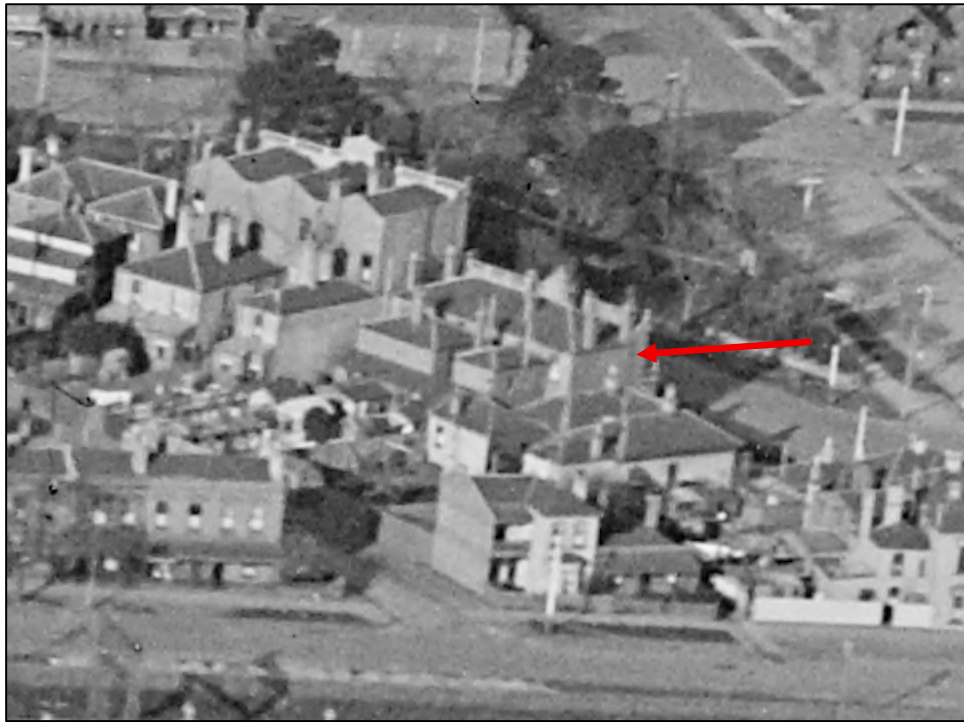
Figure 1 Extract of oblique aerial image from 1940s, with a red arrow highlighting the subject site. It appears at least two chimneys were associated with the rear wing.
