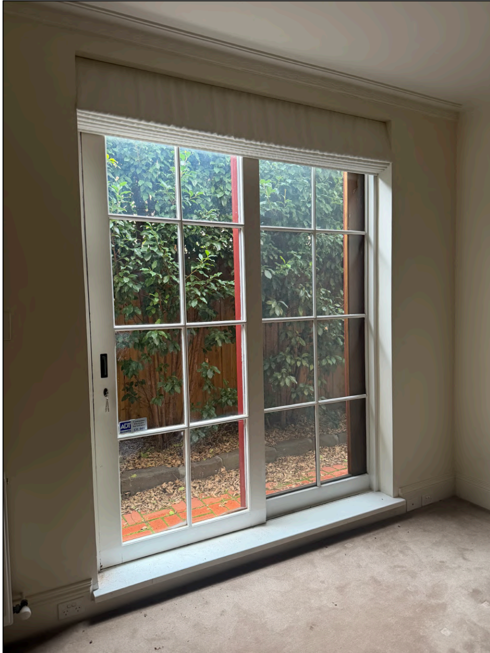
Figure 5 Modern double sliding door providing access from the original rear wing to the side courtyard.
