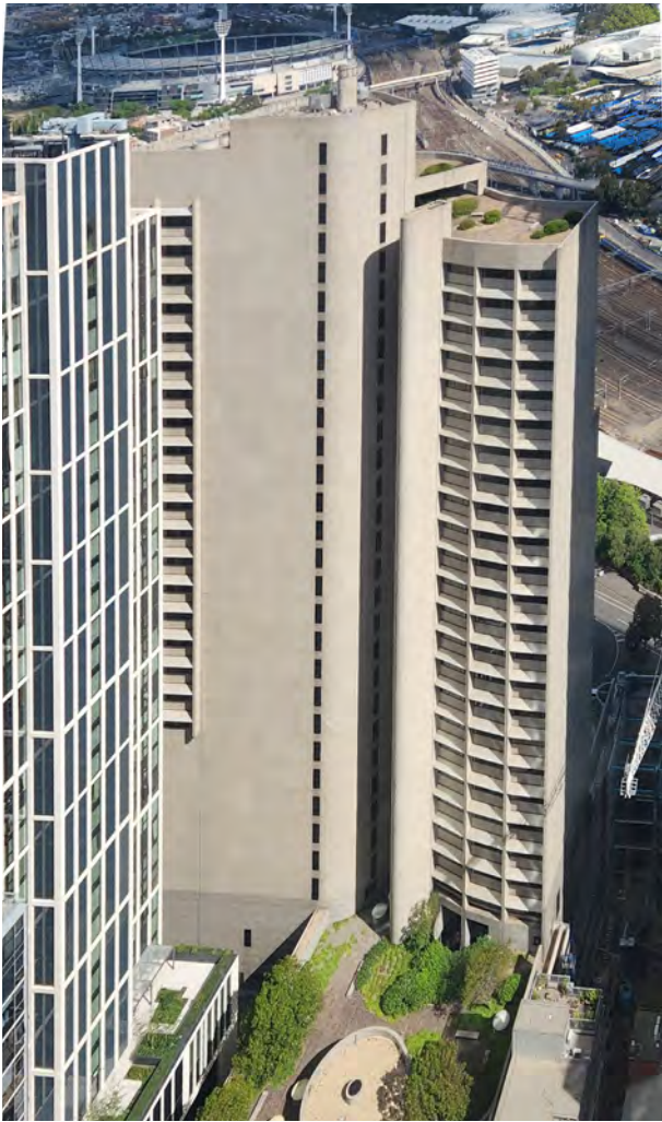
Existing Throssell Lane Facade
