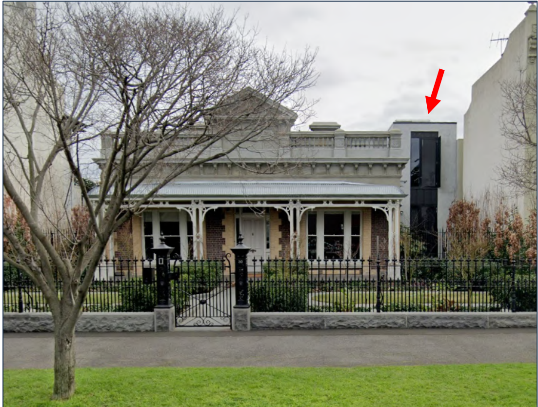
Figure 23 The single-storey Victorian residence at 30 St Vincent Place North has received a double-storey contemporary style rear addition that is partially visible from the sides and above the retained single-storey Victorian residence on the site (see red arrow).
