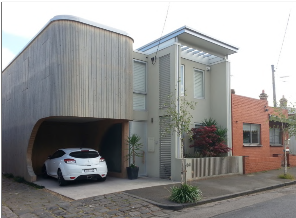
Figure 19 Modern infill at 64 Draper Street.
