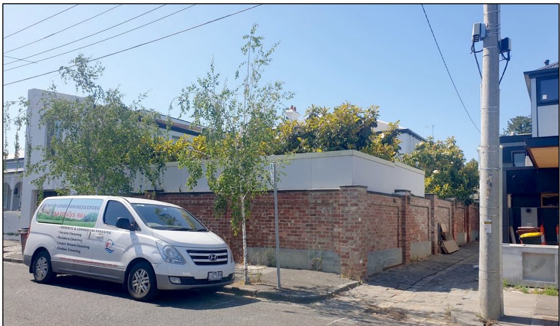
Figure 10 View of the northern Draper Street frontage of the site from the south-west, showing the existing modern red brick fence with cement sheet above. This extends along the adjacent laneway to the west (right). The former stable is partially visible at far left.
