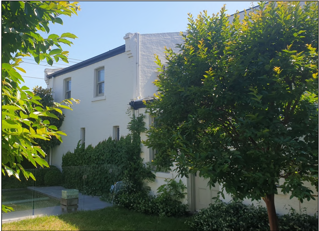
Figure 11 View of the west elevation of the former stable from within the site.
