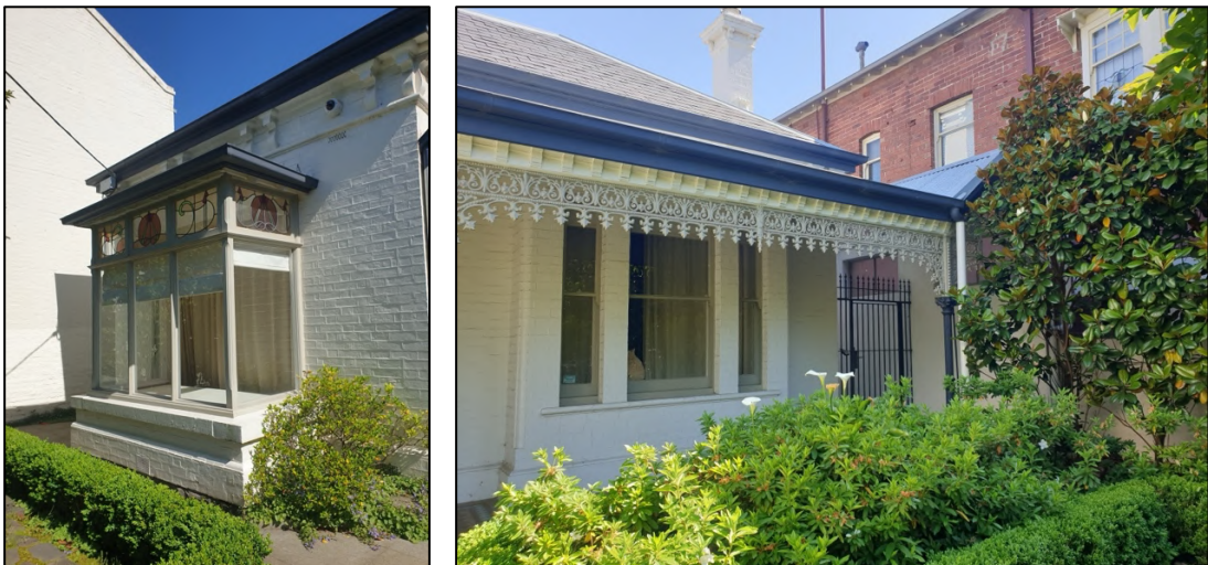
Figure 7 (left) The bay window on the west side of the facade appears to date from the early decades of the twentieth century and includes leaded glass. (right) The triple-window on the west side of the facade and the verandah.
