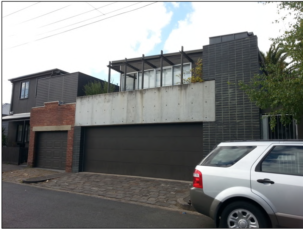
Figure 18 The rear of 78 St Vincent Place as viewed from Draper Street.
