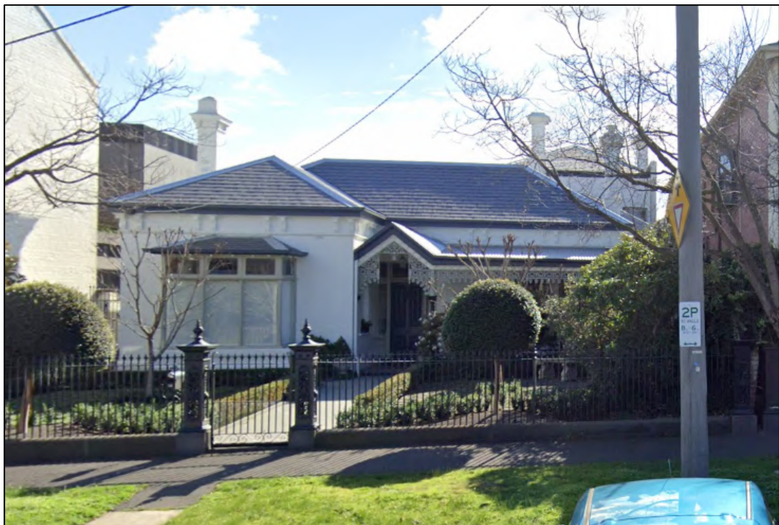
Figure 5 Recent Google Street view image of the residence from St Vincent Place North during winter. (For much of the year the house is partially obscured by deciduous trees). The double-storey rear wing is partially visible at right. A double-storey rear wing to the adjacent property to the west is also visible in the background at far left. Source: Google Maps.
