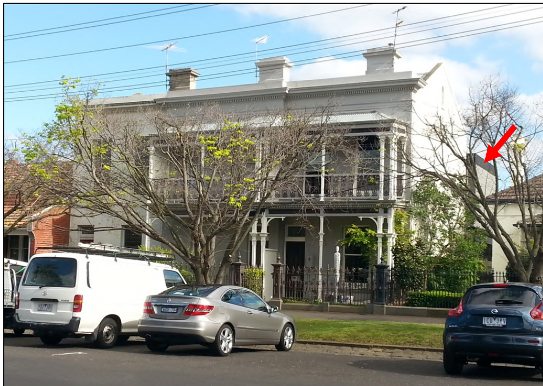
Figure 13 62-66 St Vincent Place North, adjacent the subject site to the west. This view dates from before the slate roof was installed on the house on the subject site. The location of the partially visible rear wing is shown by the red arrow.
