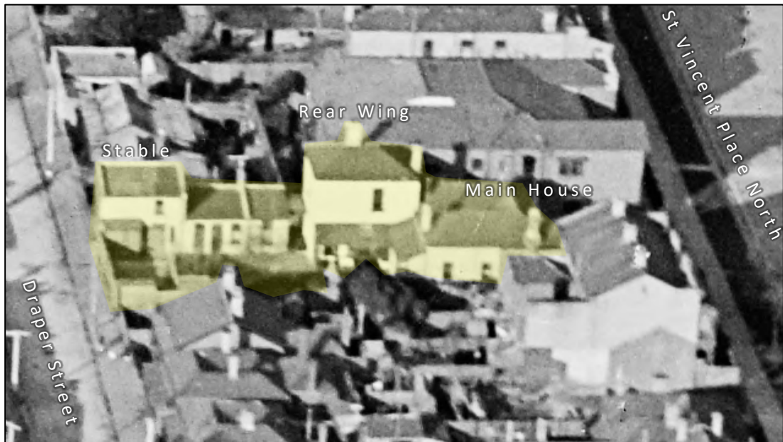
Figure 2 C.1925-1940 aerial view of 60 St Vincent Place North from the west, shaded yellow, with key elements on the site annotated. Source: http://handle.slv.vic.gov.au/10381/20433
