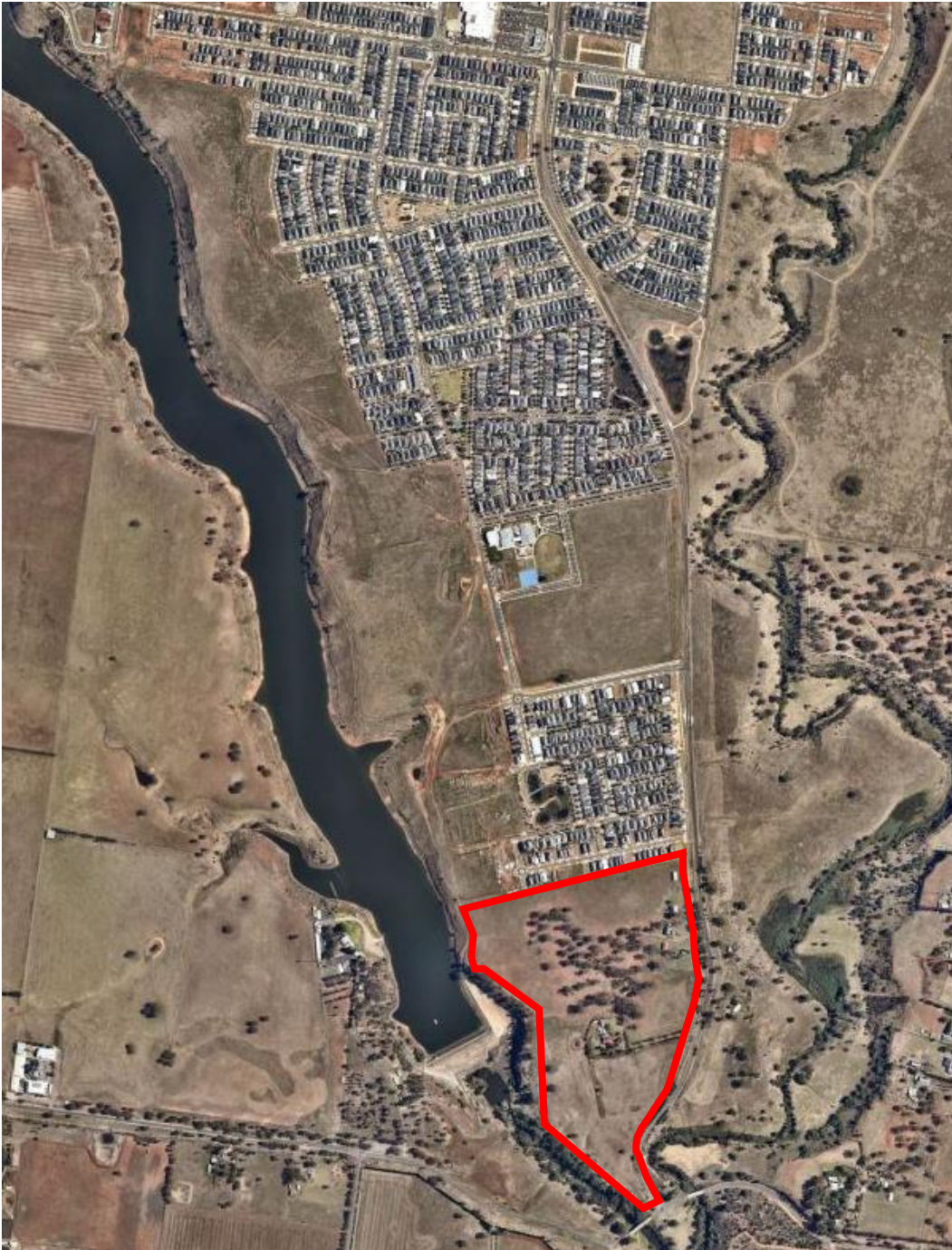
Figure 26 Recent aerial image of the Exford Waters subdivision to the north of the Exford Homestead site (approximately indicated) Source: Nearmap, image date January 2025
