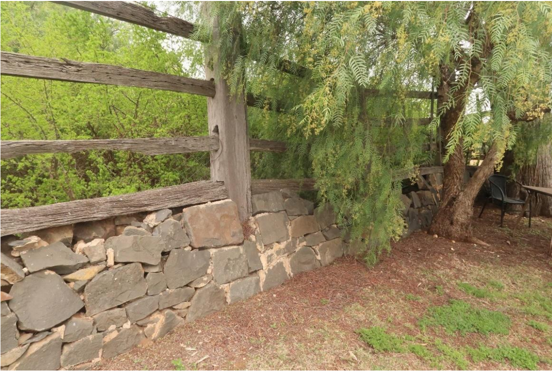
Figure 11 Bluestone wall with integrated timber post and rail fence (F3) to the north-west of the homestead (homestead precinct)
