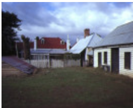
exford homestead exford street melton south rear view homestead apr1980
