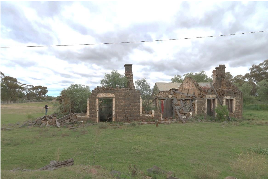
Figure 24 View to the ruin of the blacksmith's forge and residence (B12) (farm buildings precinct)
