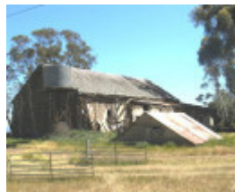
Exford barn & underground tank
