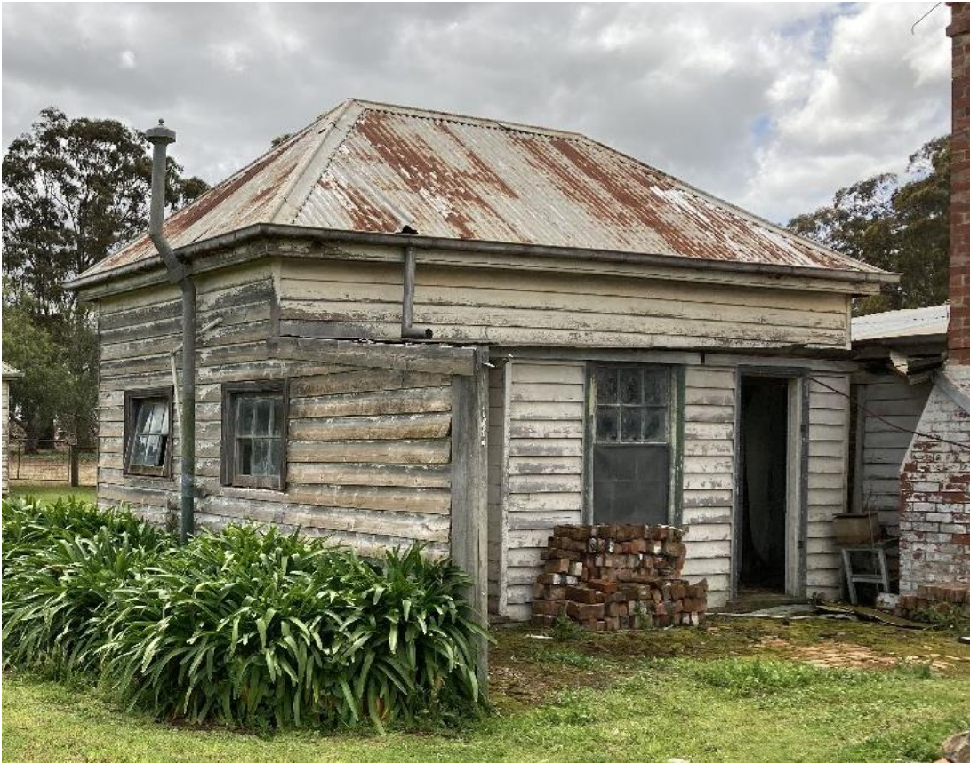
Figure 15 1930s servants' quarters adjoining the kitchen (B3) (homestead precinct)
