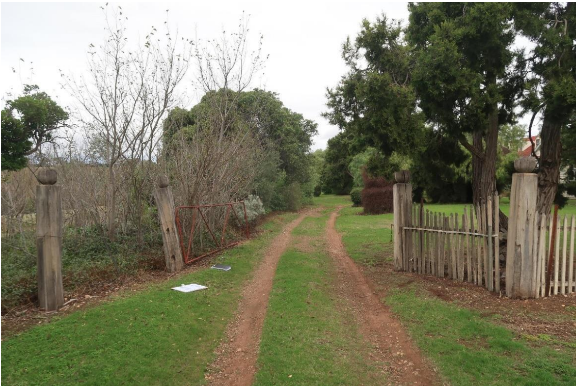
Figure 10 View along the driveway entry from Exford Road towards the entry gateposts (F2) (homestead precinct)
