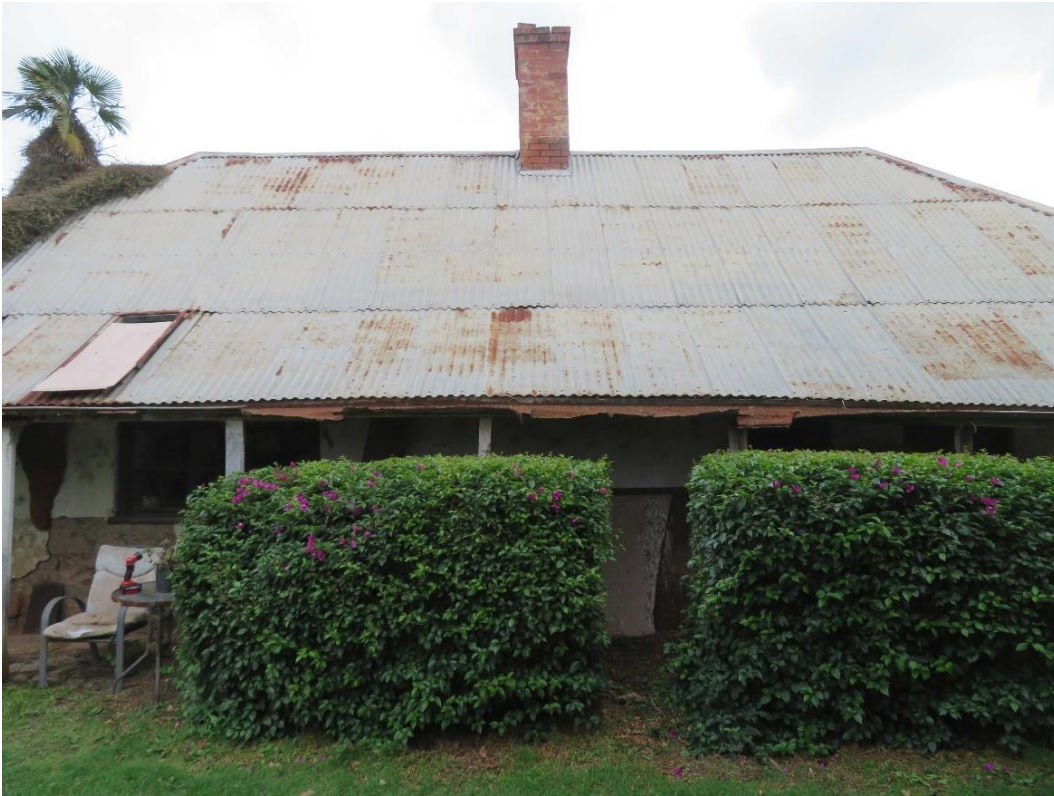
Figure 13 East elevation of the kitchen (B2) (homestead precinct)
