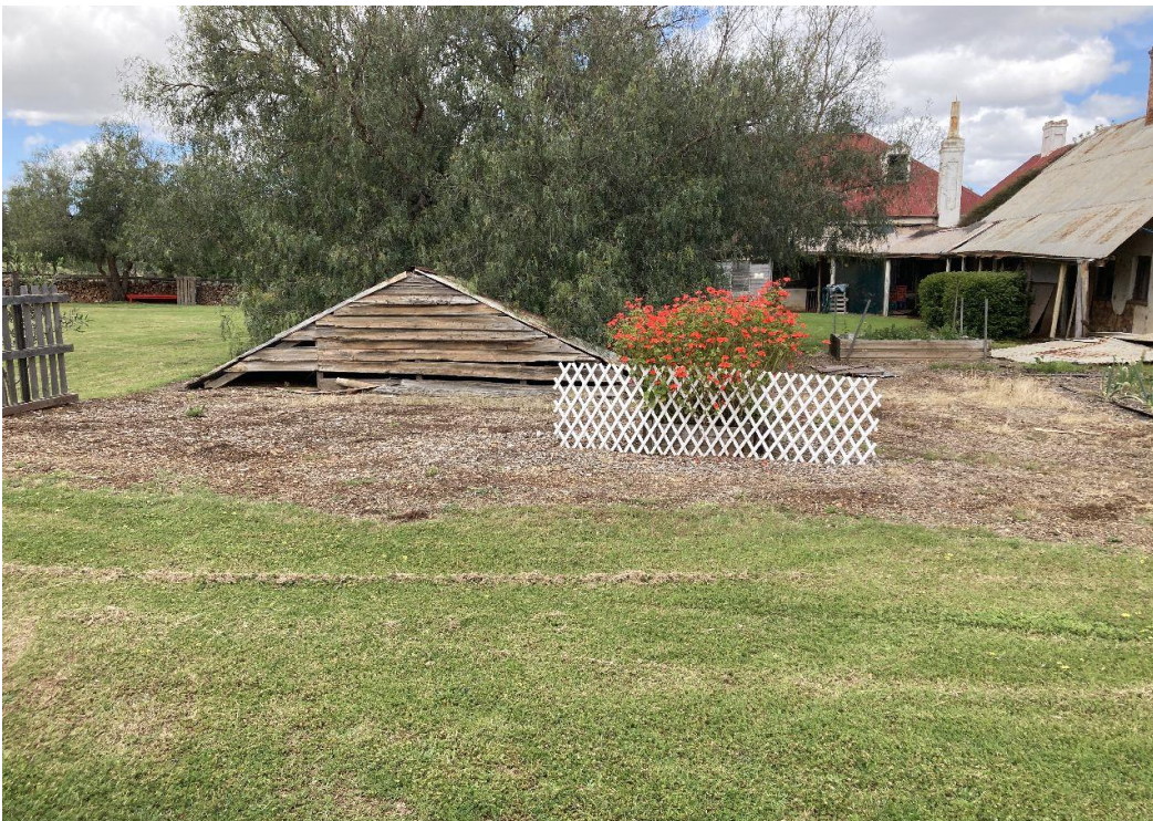
Figure 18 Covered top of the underground tank (B6) (homestead precinct)
