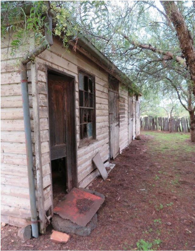
Figure 17 North elevation of the timber stable (B5) (homestead precinct)
