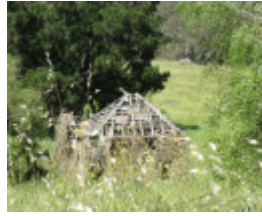
Exford gardener's cottage
