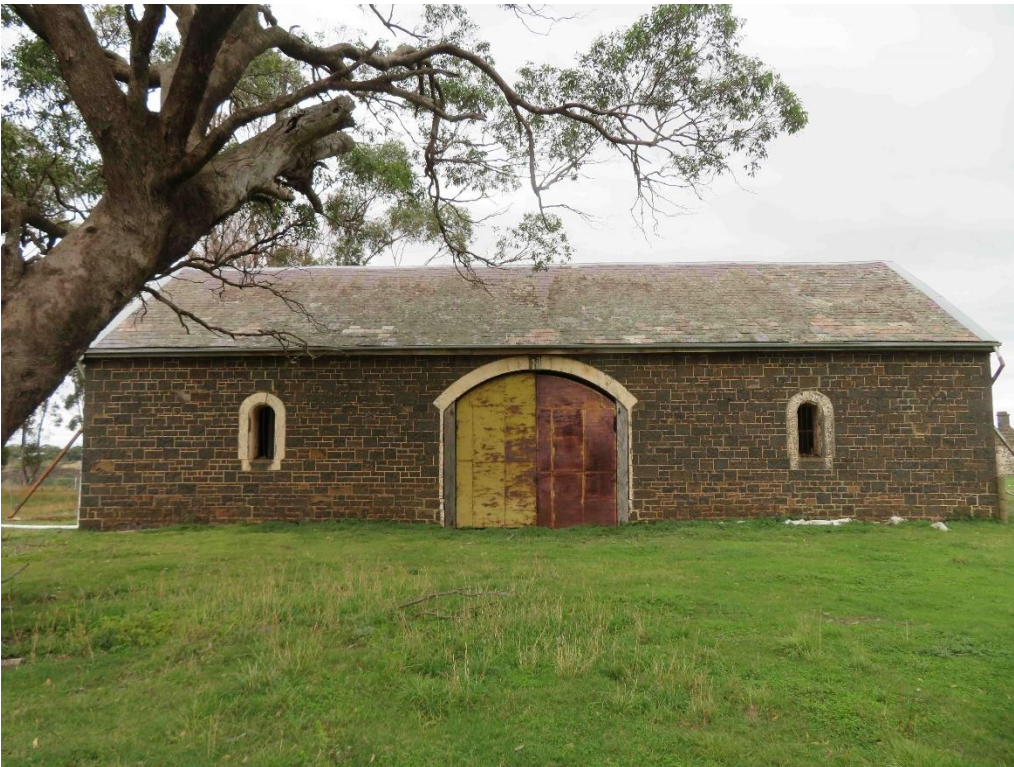
Figure 22 West elevation of the barn/coach house (B10) (farm buildings precinct)
