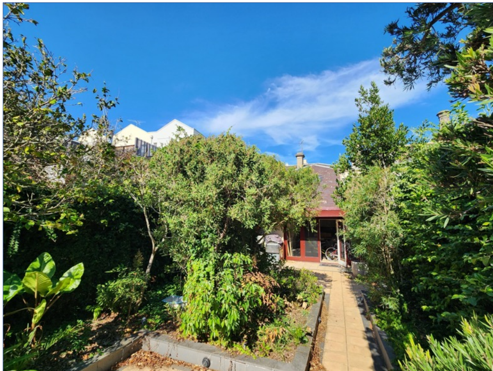
Figure 9 Rear of the house as seen from near the garage.
