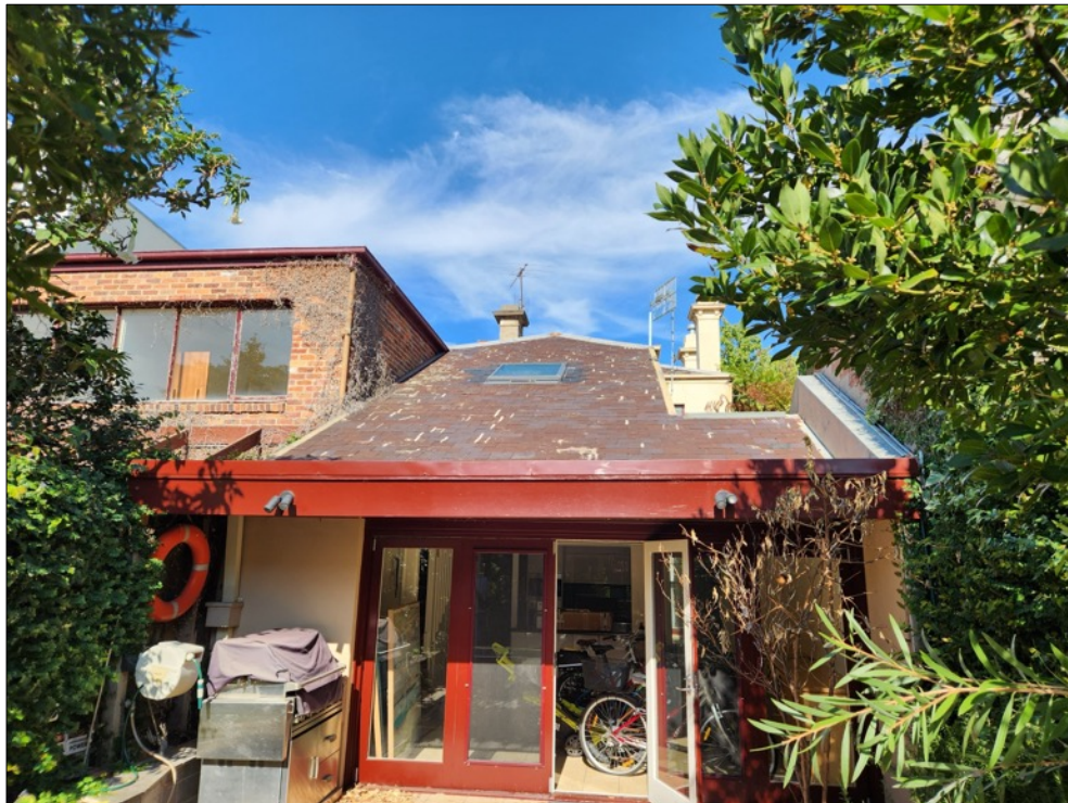
Figure 6 The rear wing, which has been altered. Note the double storey wing to the adjoining residence at no. 47 is also a non-original element.
