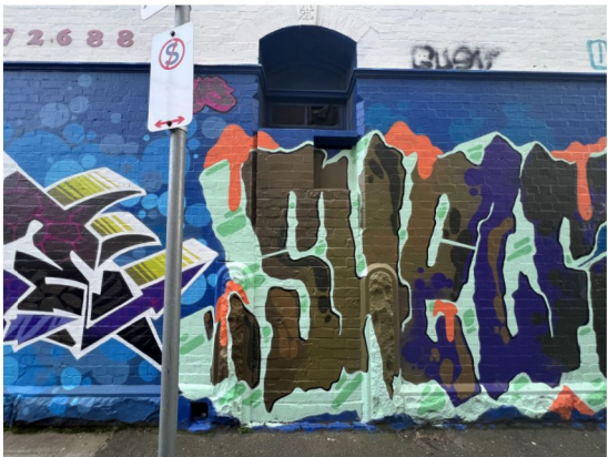
Fig: Existing infilled doorway to be restored to a door.
