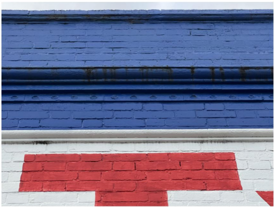
Fig: Existing render moulding to be depainted and restored to a face finish.
