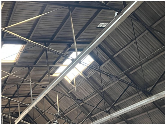
Fig: Existing internal lining boards and trusses to be repaired and repainted.
