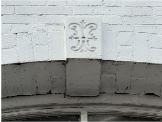
Fig: Existing window head keystone detail to be depainted and restored to a face finish.
