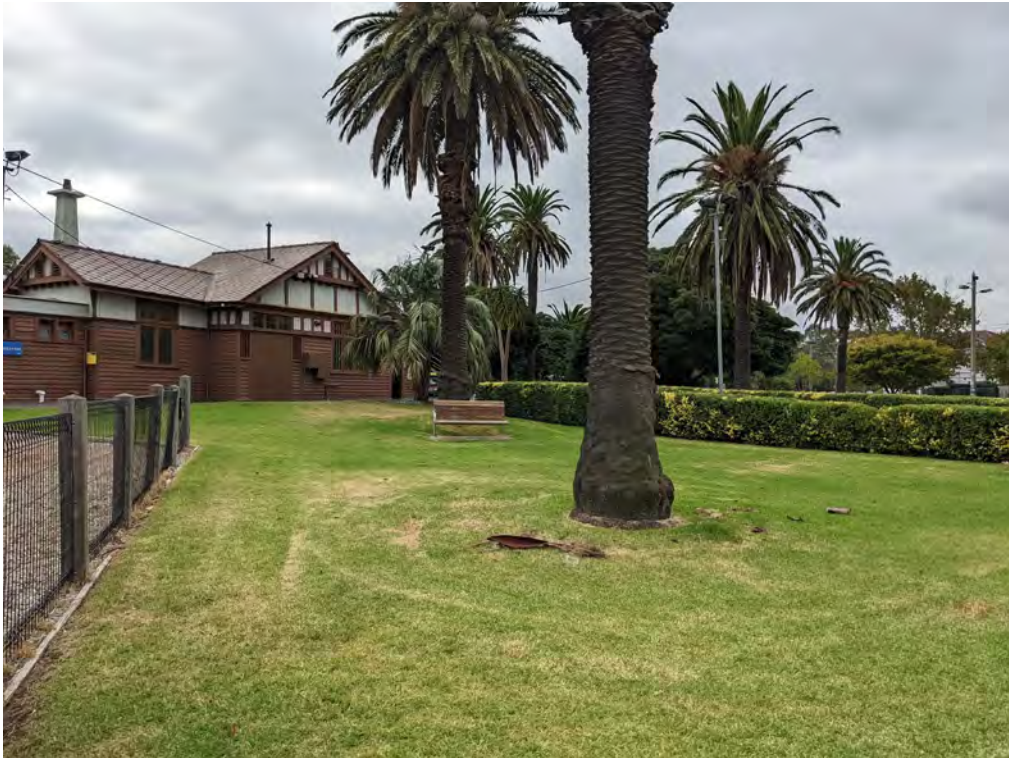
Plate 3: View of the site looking west towards the train station. Note good quality grass coverage.
