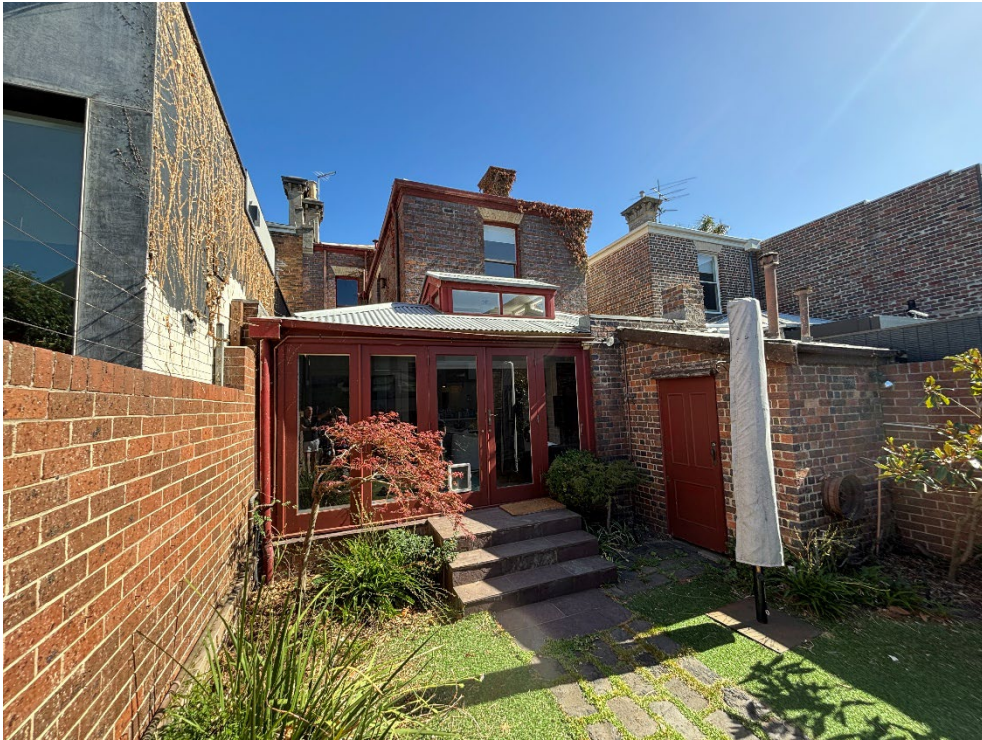
Figure 6 – The photo above is taken from the backyard, looking north towards the existing residence. Pictured here is the existing living room and shed.
