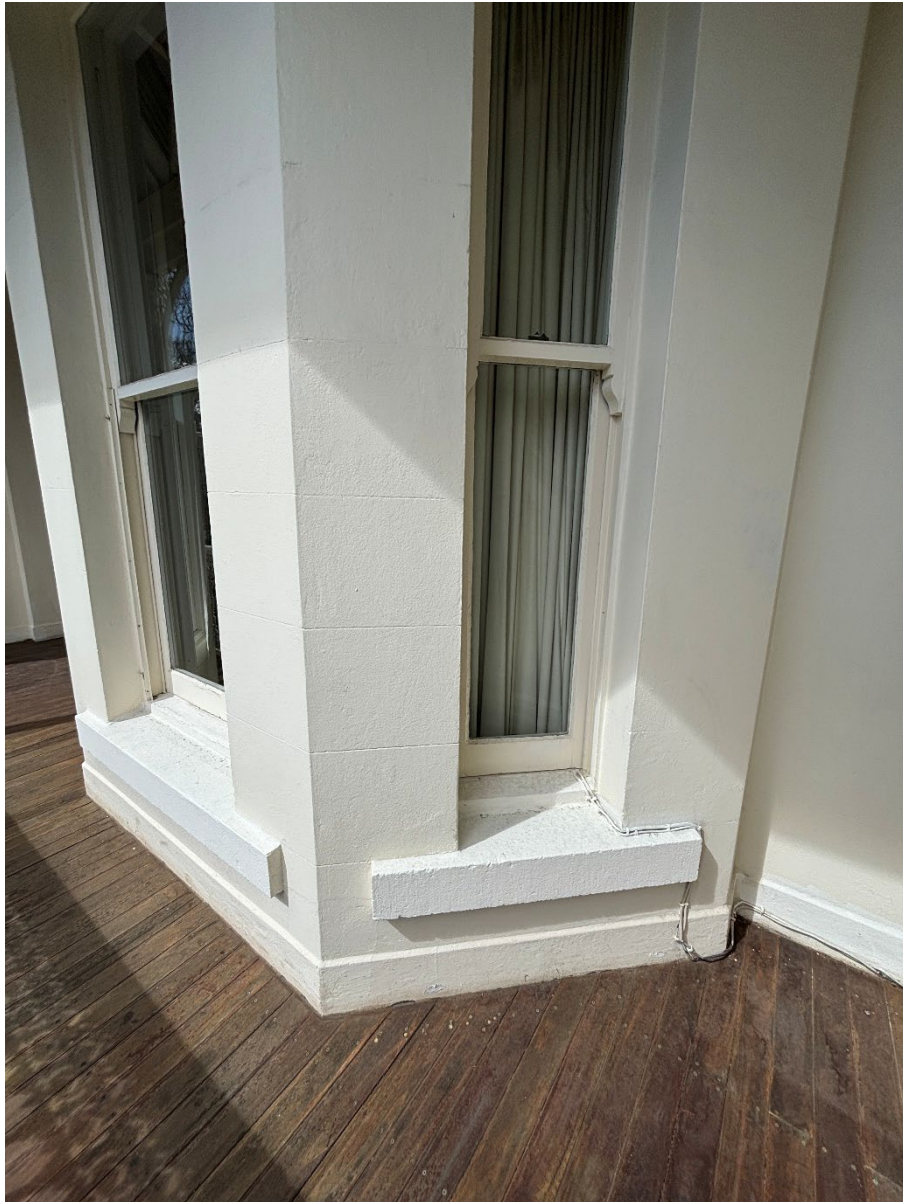
Figure 3 – The photo above shows the existing façade, generally in good condition.
