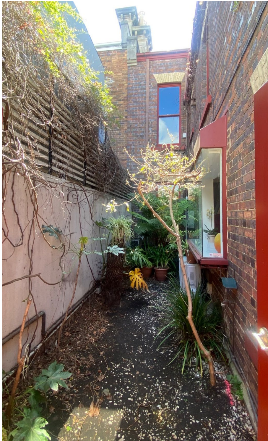
Figure 9 – Existing lightcourt pictured above.
