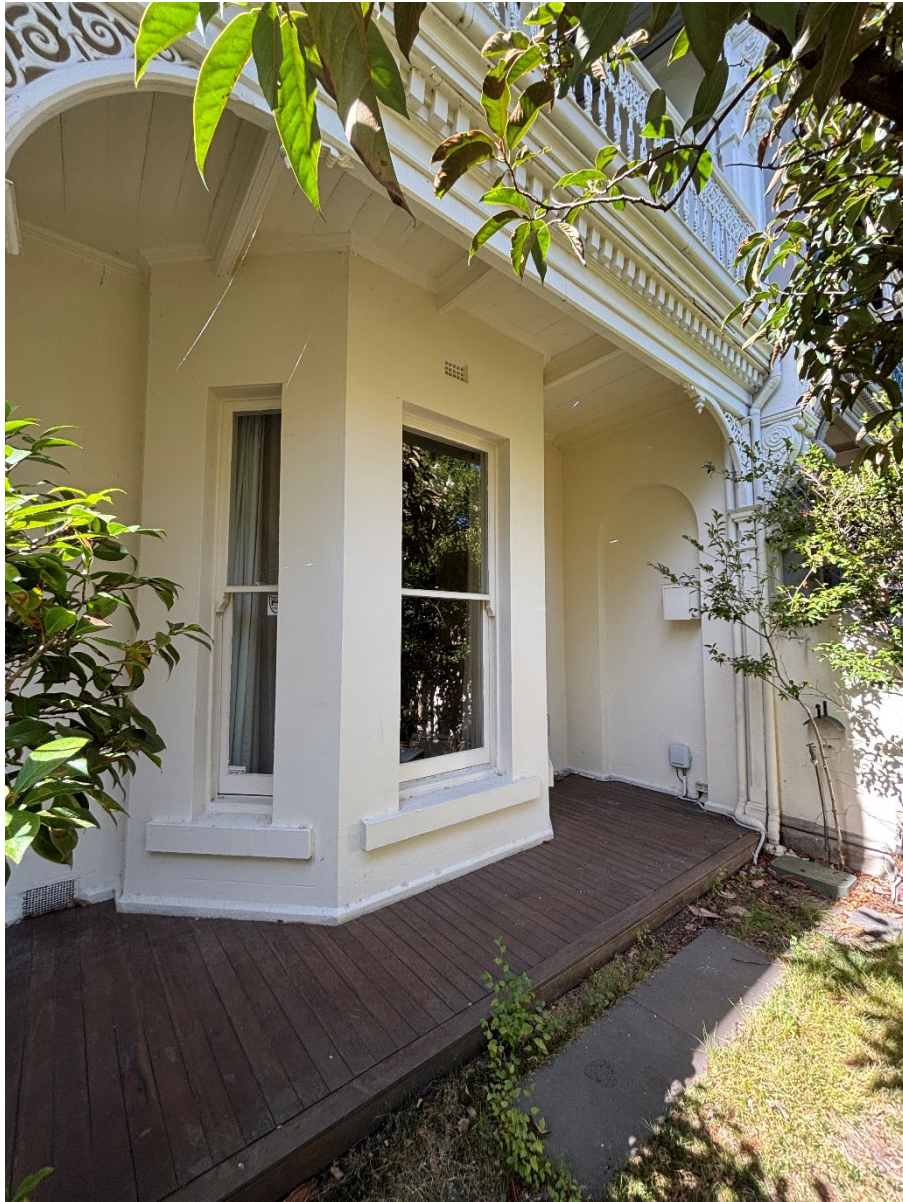
Figure 4 – The photo above shows the existing verandah timber decking. It is proposed to remove the existing timber edging and reinstate it with basalt edging to match No. 11.
