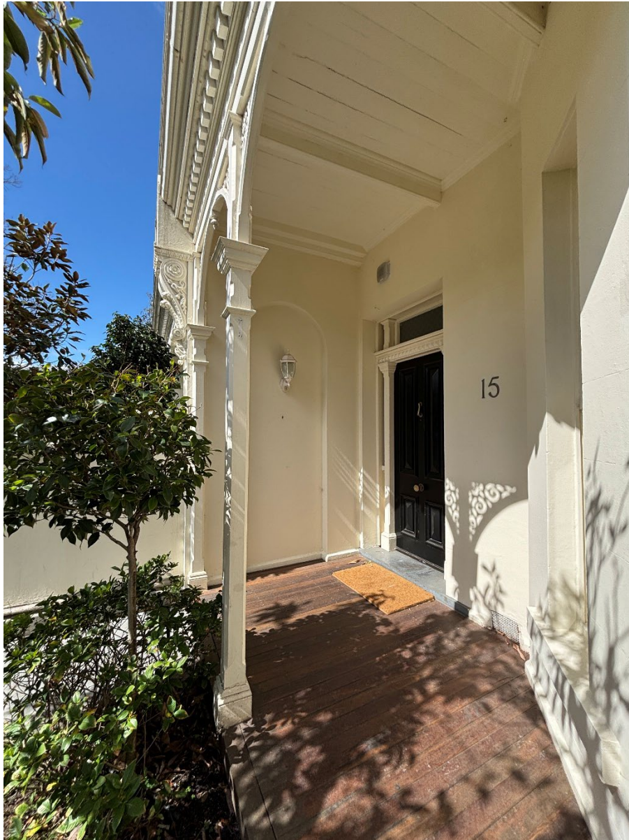
Figure 2 – The photo above shows the existing façade, generally in good condition.
