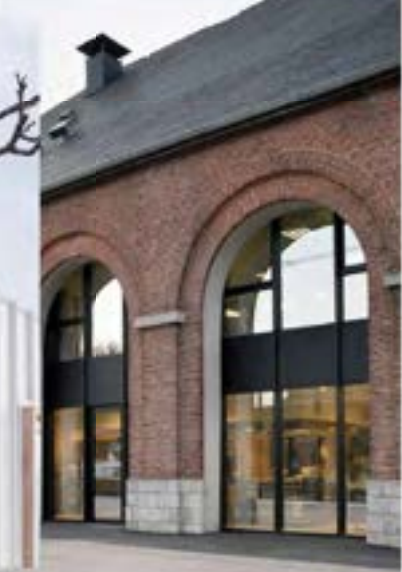
ARCH WINDOW WITH ALUMINIUM FRAME, POWDERCOATED FINISH, MOUNUMENT
