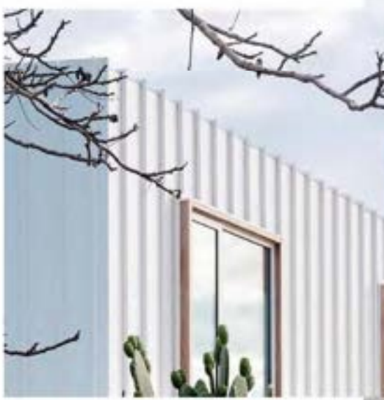
MC01 METAL CLADDING, COLORBOND FINISH, SURFMIST
