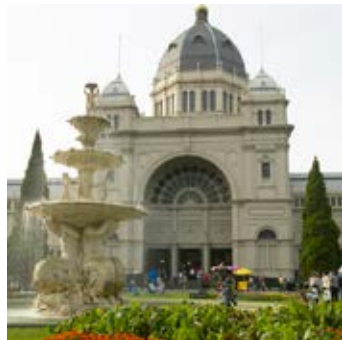
Opportunity to reprioritise a universally-accessible entrance via the Southern facade.
