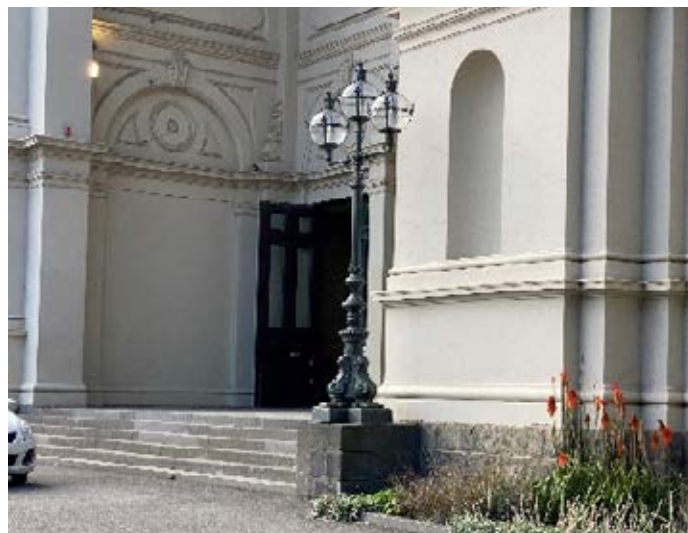
The reinstated cast iron gasoliers at the western entrance to the Royal Exhibition Building. Matching cast iron gasoliers should be reinstated on the south and eastern entrances. Source: Conservation Studio.
