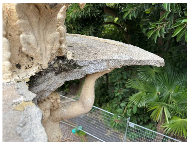
figure 8 – smaller dish section (2026) note the infill cement
