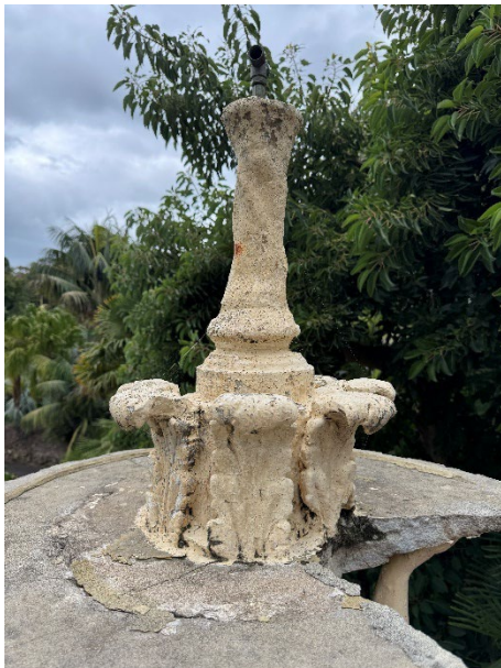
figure 6 – smaller dish of fountain (2026) note the circle line of infill cement
