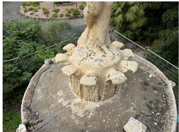
figure 7 – larger dish of the fountain (2026) note the similar circle of infill cement
