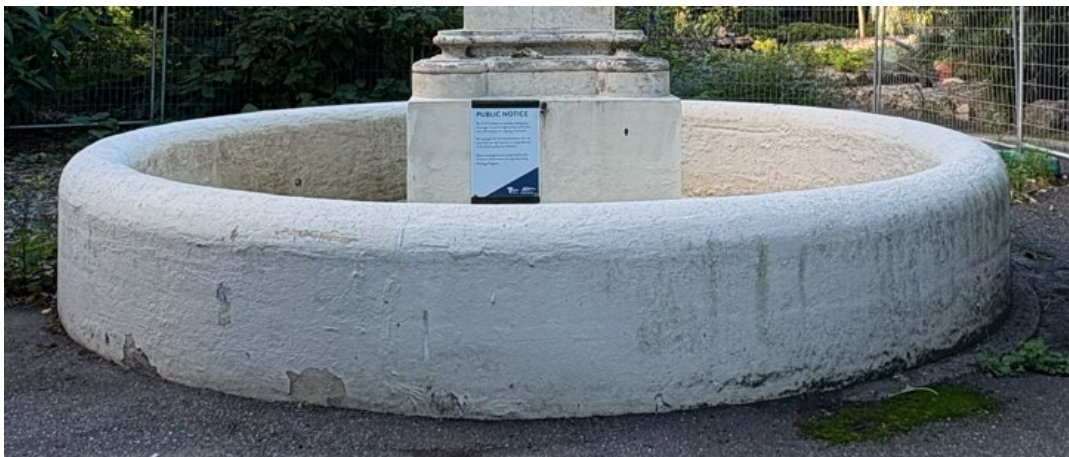
figure 12 – lower rendered brickwork section of pedestal and pond wall (2026)
