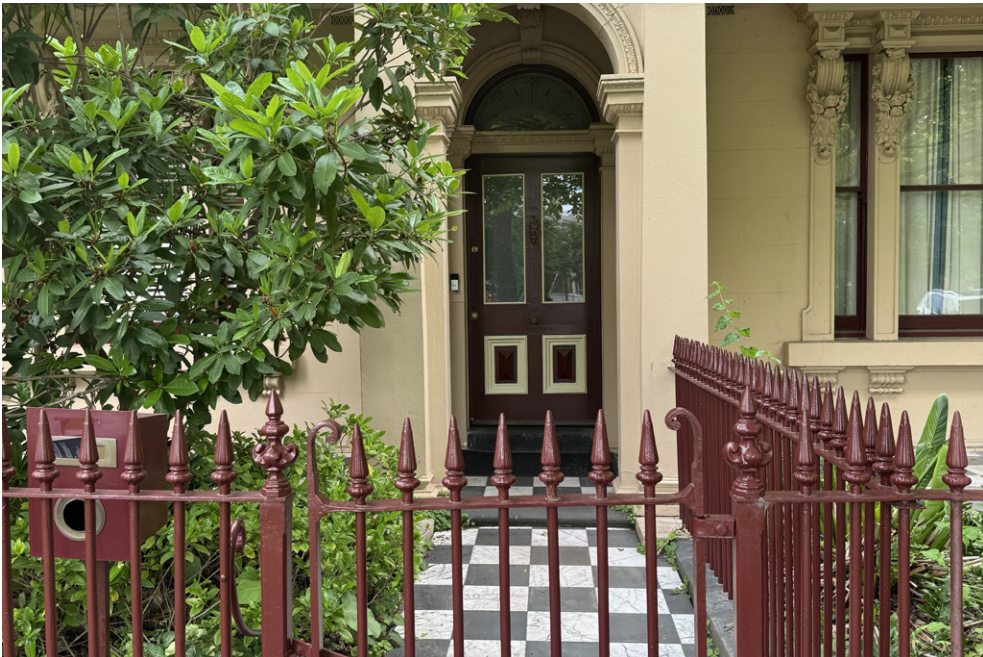
48 Howe Crescent - Entry
