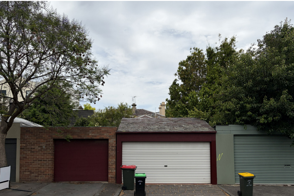
48 Howe Crescent - Martin Street (White Garage)
