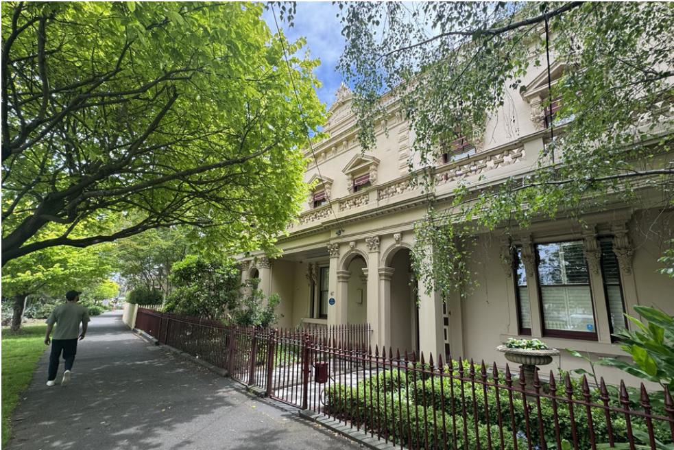
East Approach, from 46 Howe Crescent
