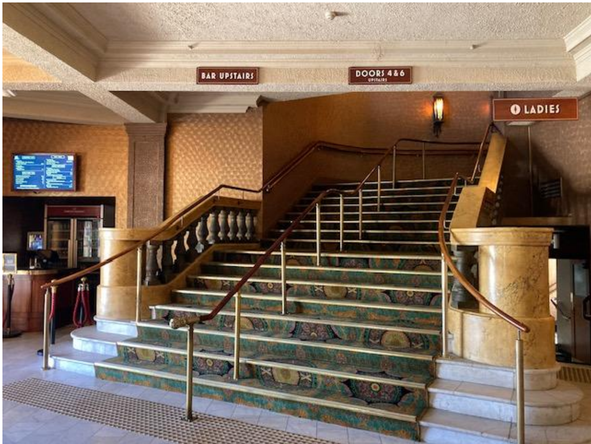
Figure 1, Palais Theatre Main Stair west side, existing conditions.
