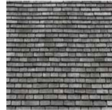
RF-01 Slate Roofing (Existing)
