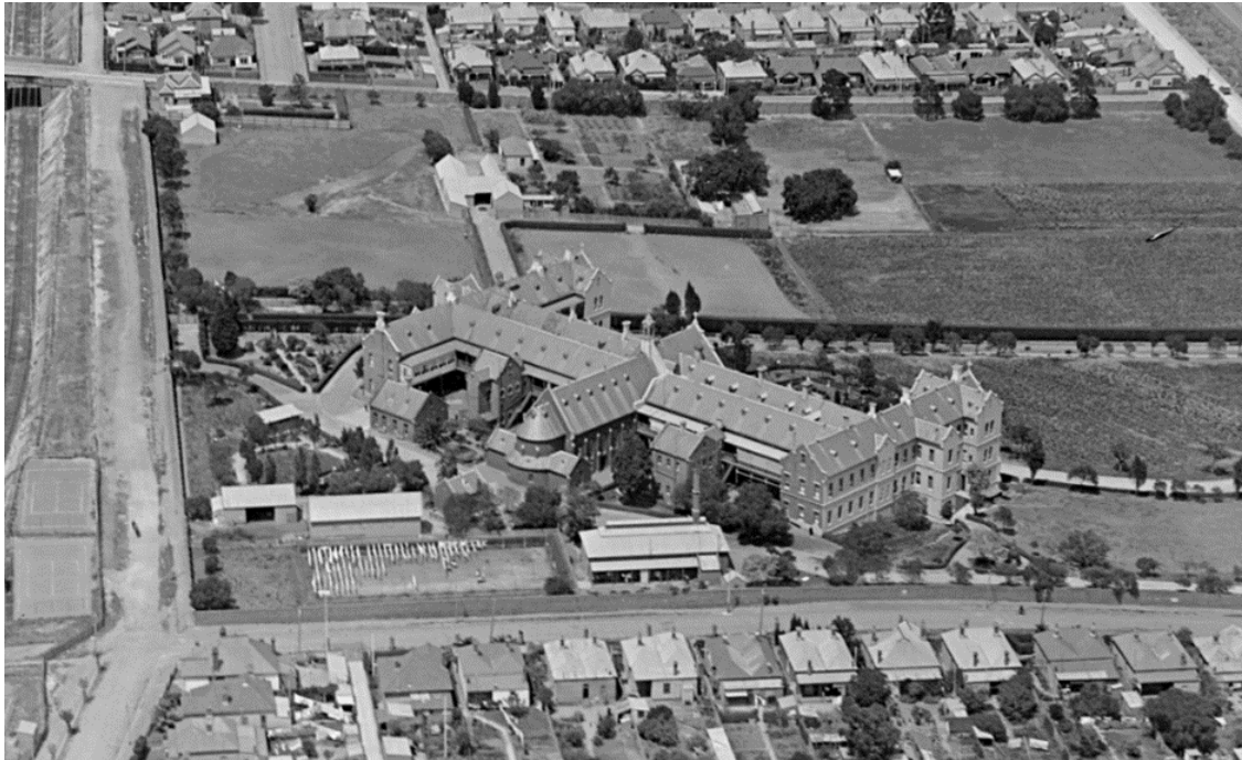
Figure 15. Looking north to Little Sisters of the Poor convent, extract from 'Northcote' by Pratt c.1928. Source: State Library of Victoria, H91.160/390.
