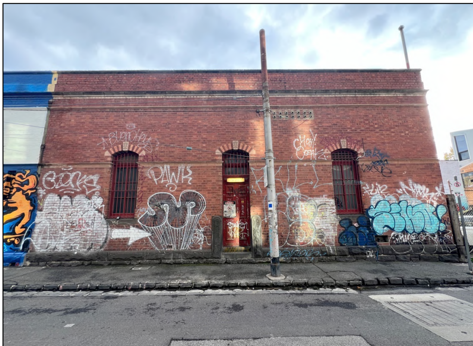
Figure 12 The adjacent northern bay of the complex at 1 Black Street (outside the subject site) has not been overpainted and shows the original bi-chromatic brickwork.
