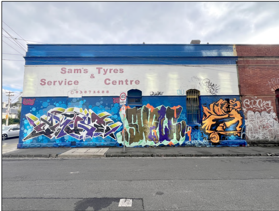
Figure 11 The overpainted east elevation of the building to Black Street originally contained three openings, the southern of which (centre left) has been infilled.
