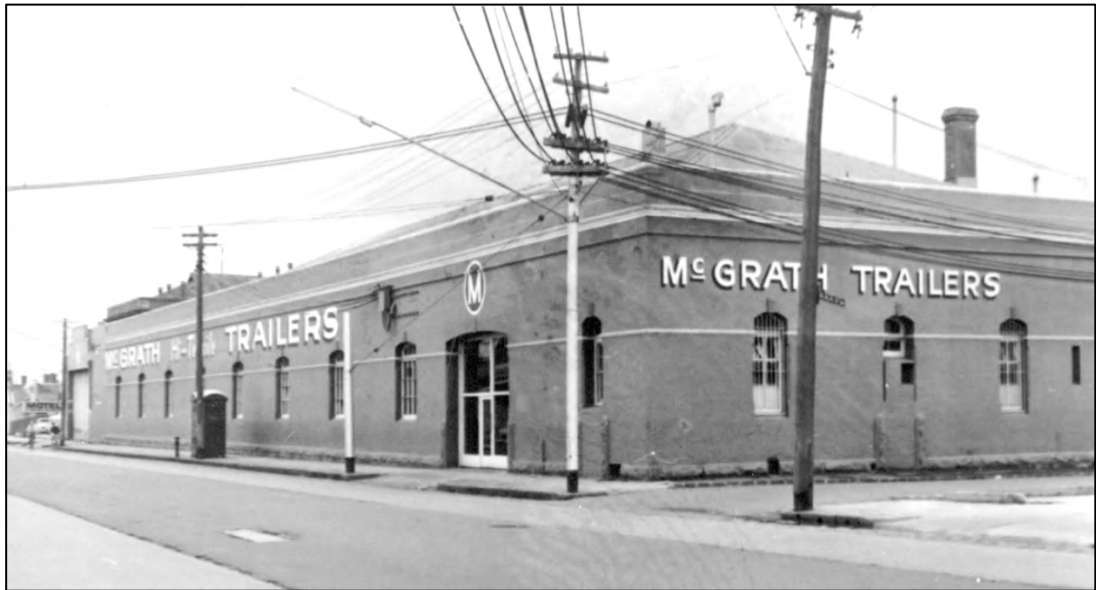
Figure 4 c. 1966-71 view from the south-east showing the originally full face brick external treatment, with a greater degree of intactness to the original fenestration. The original large chimney had been removed by this time. Source: University of Melbourne (courtesy of Leigh Harding).
