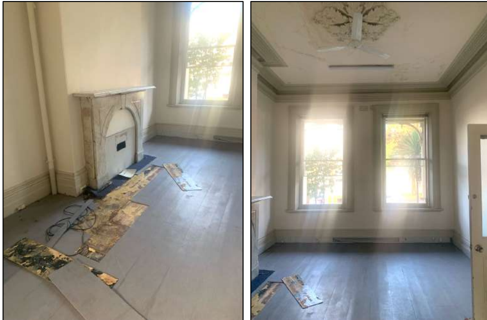
Figure 11 (left) Original marble fireplace in the front room at ground level. (right) Original cornices and ceiling rose in the front room at ground level.
