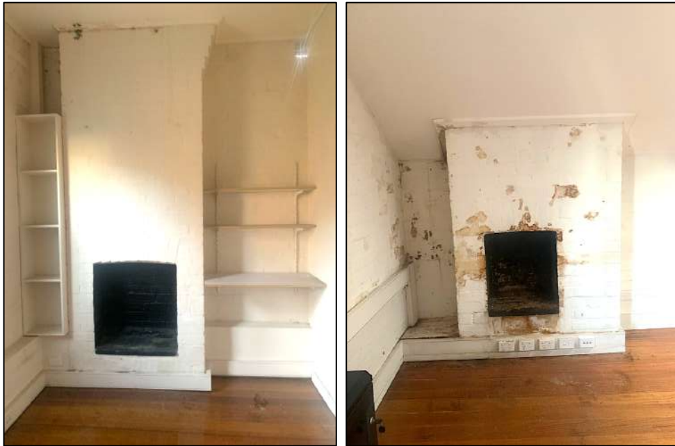
Figure 10 (left) The original brick chimney to the stable at ground level, (right) the chimney on level 1.
