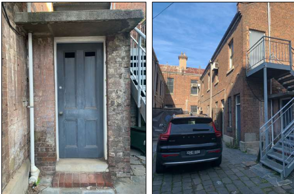
Figure 9 (left) View of the original brick outhouse building, (right) rear of the primary dwelling.
