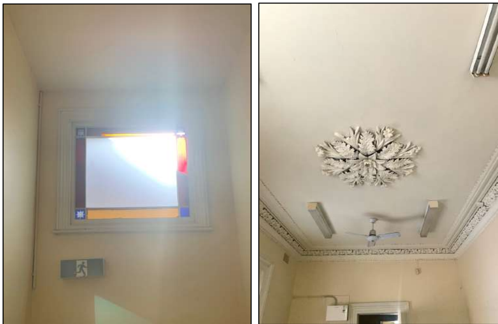
Figure 12 (left) Window with decorative stained glass border over the stairway. (right) Decorative cornices and ceiling rose featured at the ground floor rear room (room 5).
