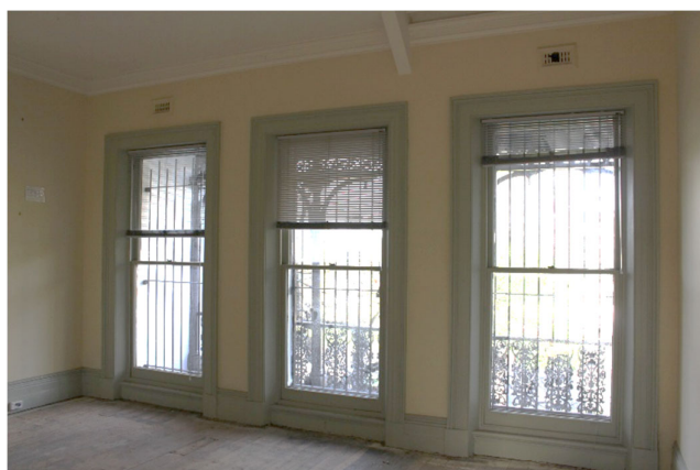
Figure 20: First floor windows with original skirtings and architraves (RBA 5 June 2026)
