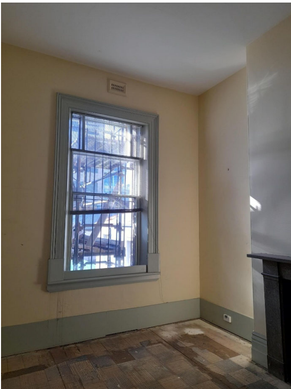
Figure 35: First floor, front wing, rear room note elaborate architrave moulding (RBA 12 May 2026)
