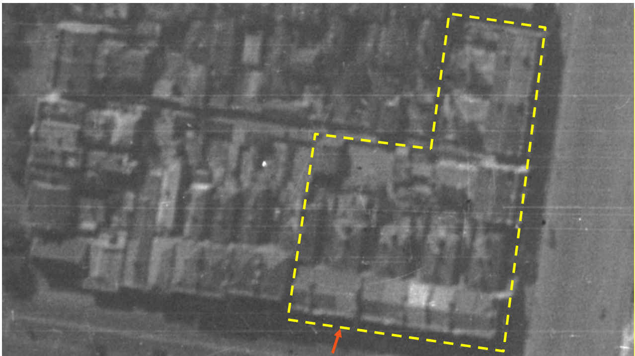
Figure 10: Detail of a 1942 aerial showing the subject site (arrow) in relation to the terrace group (dashed) (Geoscience Australia, Map 1820, run 15, frame 72333)
