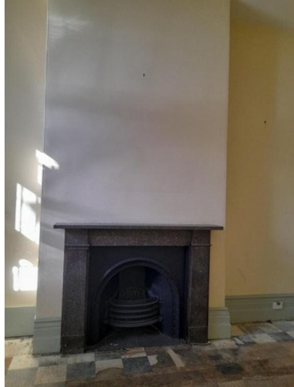
Figure 34: First floor, front wing original fireplace (RBA 12 May 2026)
