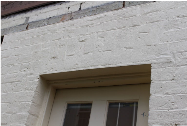
Figure 17: Overpainted brickwork with voussoir over doorway (RBA 6 August 2026)
