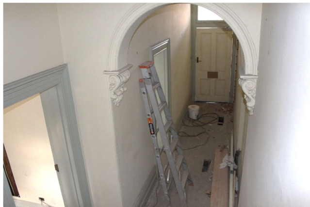
Figure 46: View of hallway looking towards front room (RBA 6 August 2026)
