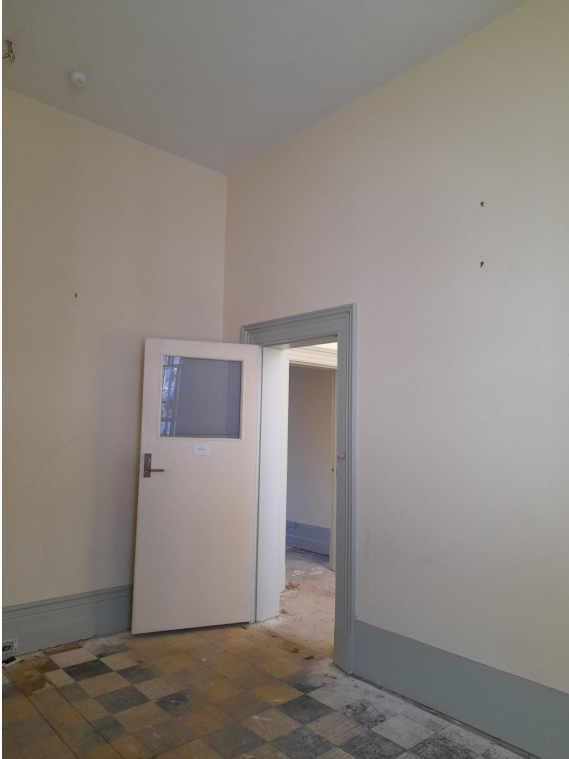
Figure 33: First floor room example of non-original door (RBA 12 May 2026)
