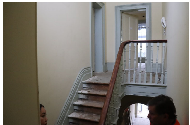
Figure 32: First floor, landing of front wing (RBA 4 June 2026)
