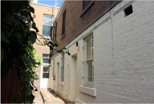
Figure 15: Side (east) elevation at rear of the property (RBA 6 August 2026)
