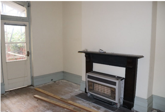
Figure 29: Ground floor, second room fireplace and non-original door (RBA 4 June 2026)
