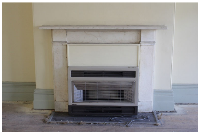
Figure 48: View of level 1 fireplace to be conserved (RBA 6 August 2026)
