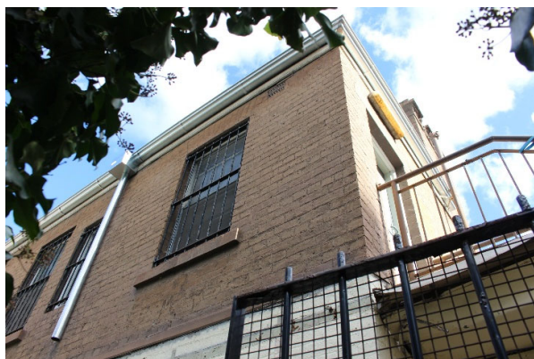
Figure 42: View of wall where one of the condenser units is proposed to be mounted (RBA 6 August 2026)
