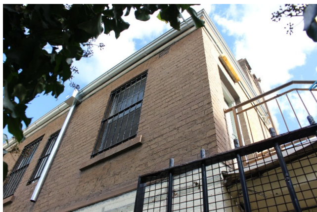
Figure 25: Rear wing, north end (RBA 6 August 2026)
