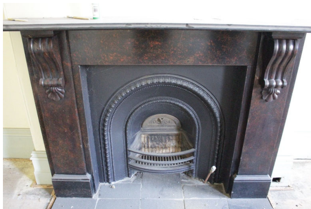
Figure 18: Marble fireplace surround ground floor (RBA 5 June 2026)
