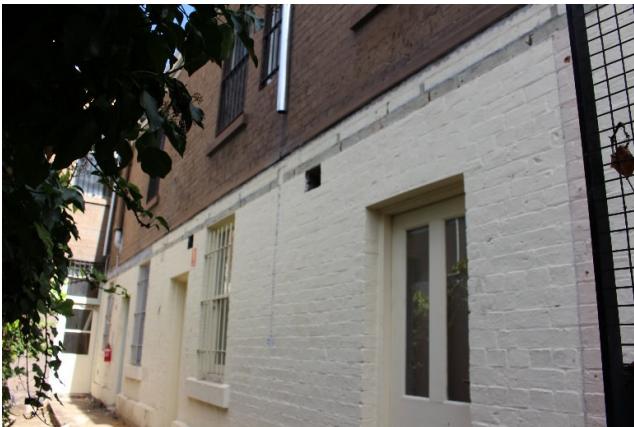
Figure 38: View of east elevation of rear of building (RBA 6 August 2026)
