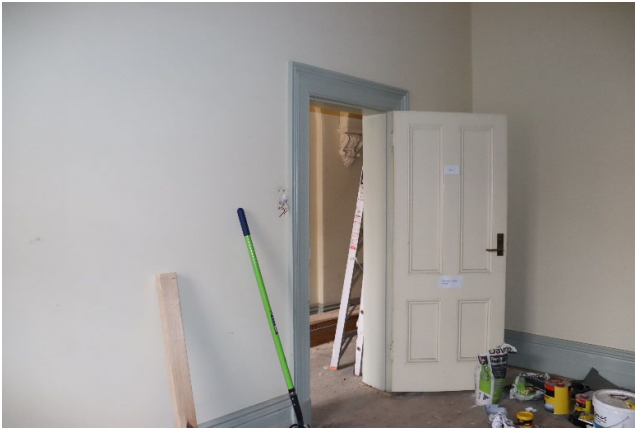
Figure 27: Ground floor, front room to hallway with original door (RBA 4 June 2026)
