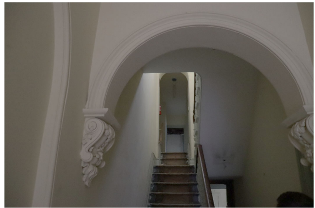
Figure 30: Stair from hallway (RBA 4 June 2026)
