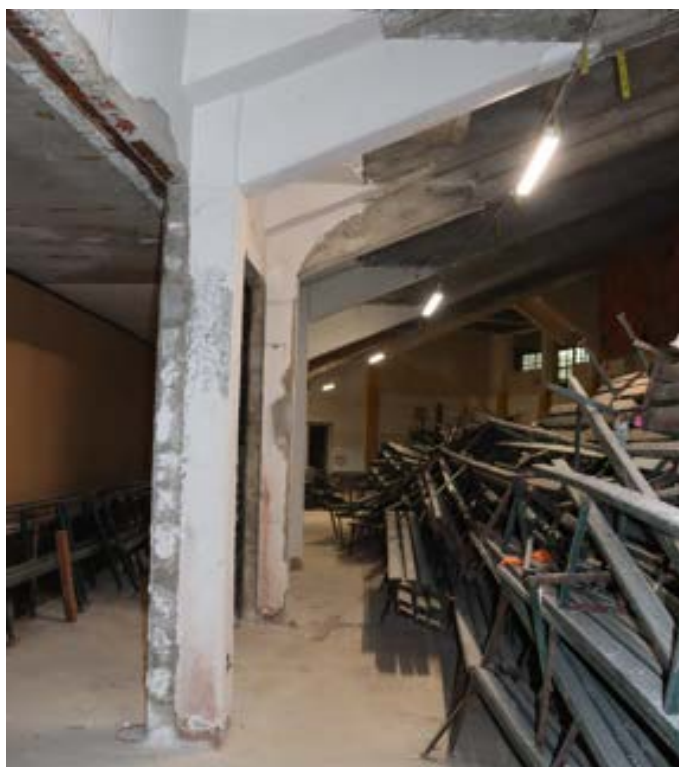
Figure 23: Undercroft interior showing the impact of structural remediation works and storage of original timber seating and balustrades
