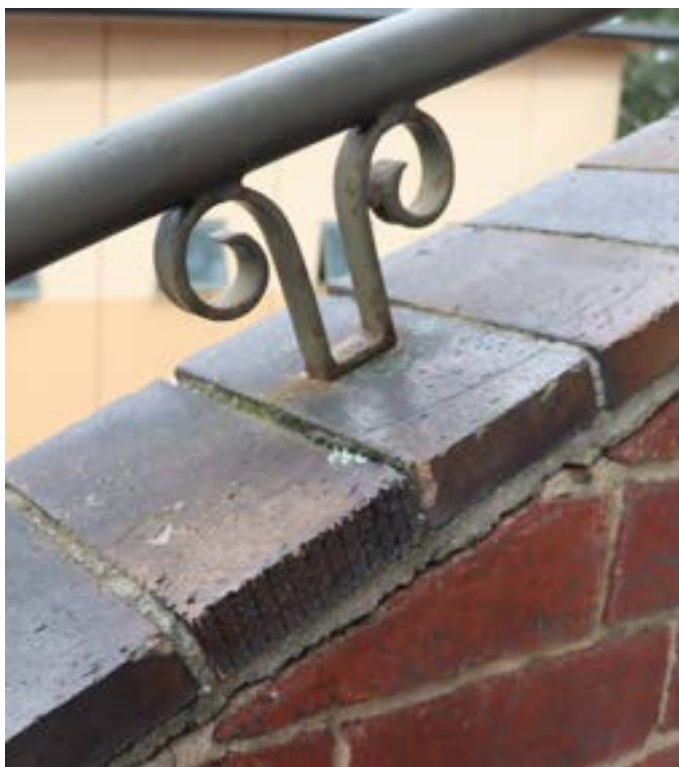
Figure 22: Balustrade at grandstand seating area showing umber slips capping brickwork and decorative curved steel bracket attached to handrail
