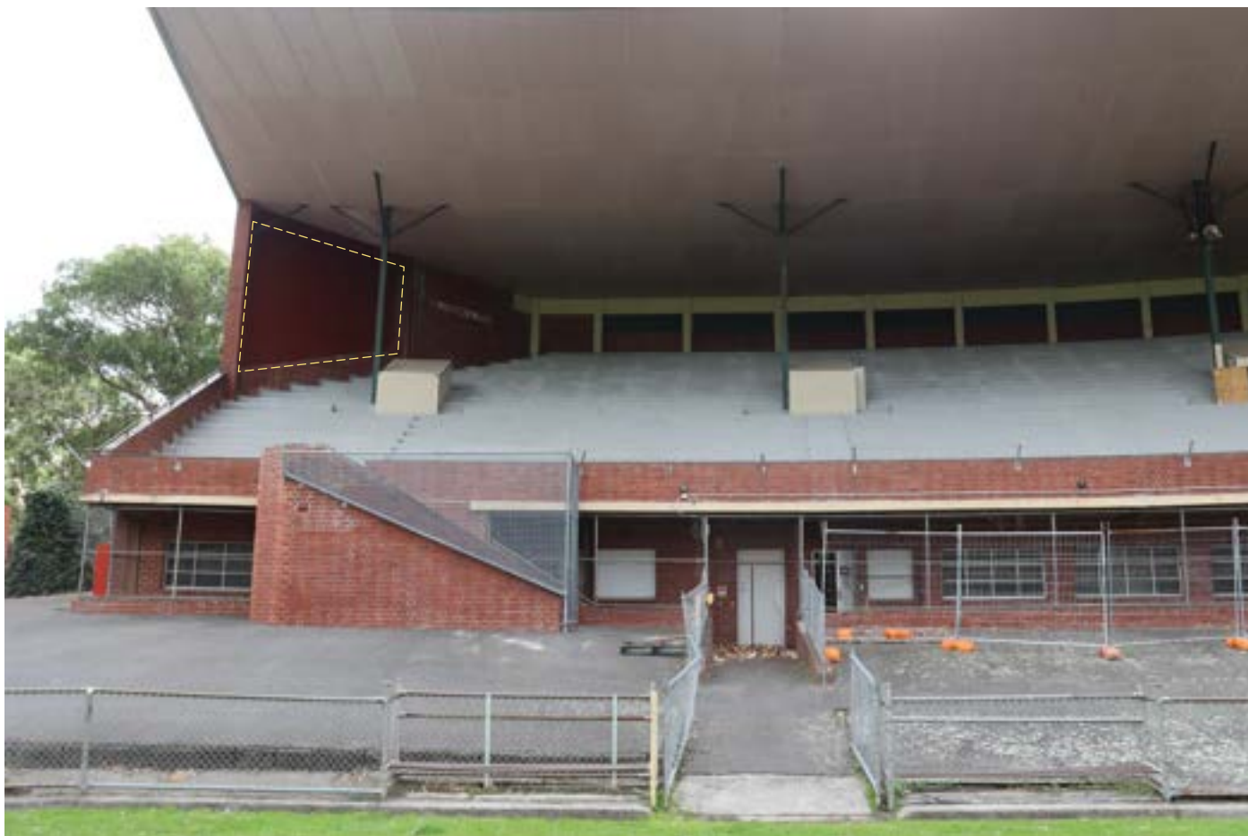
Figure 21: Front of the grandstand showing the race/run out emerging from the covered way, as well as access stairs to the south. Note the metal cladding infilling a previously open section of the southern wing wall (indicated by dash).
