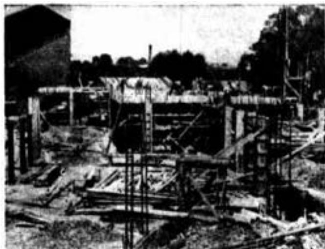
WORK IS PROGRESSING RAPIDLY on the new stand at the Glenferrie Oval. Costing £15,000, the stand will have three tiers, seat 2000 and be completed before the start of the football season.
