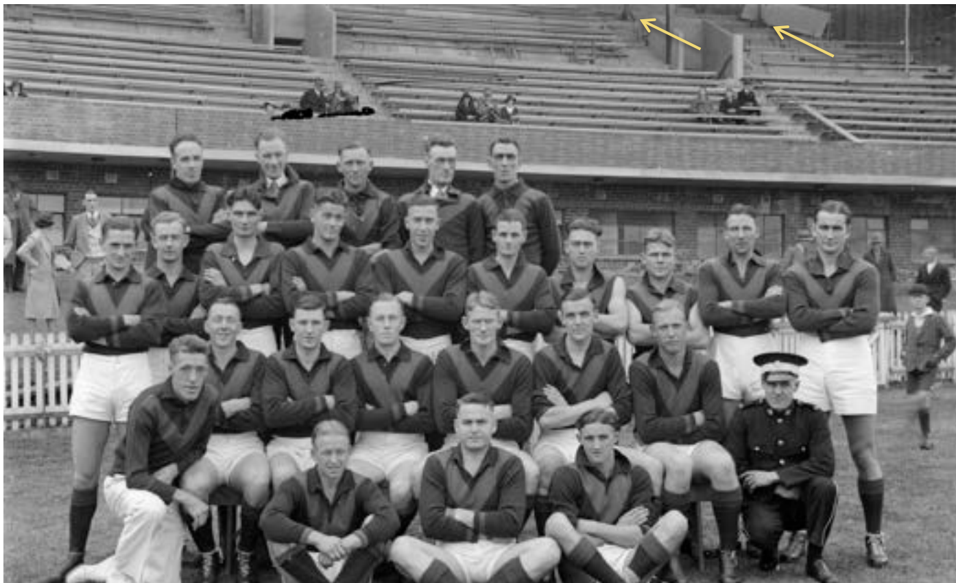
Figure 10: c1938 team photograph taken in front of the grandstand during the final stages of construction – most likely in April or early May 1938. Here, the introduction of seating is still taking place, with some vertical propping (indicated by arrow) visible within the upper levels of the grandstand. Additionally, balustrades, handrails, signage, and fencing had not yet been fully introduced when the photo was taken. (Charles Edward Boyles, SLV, H2008.122/96)
