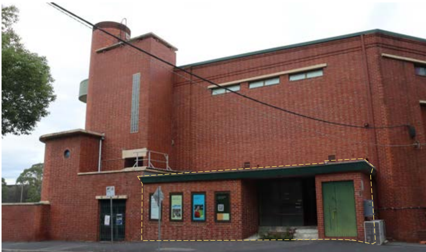
Figure 29: North elevation showing entrance foyer with tower and turret – non-original brick entrance foyer indicated by dash
