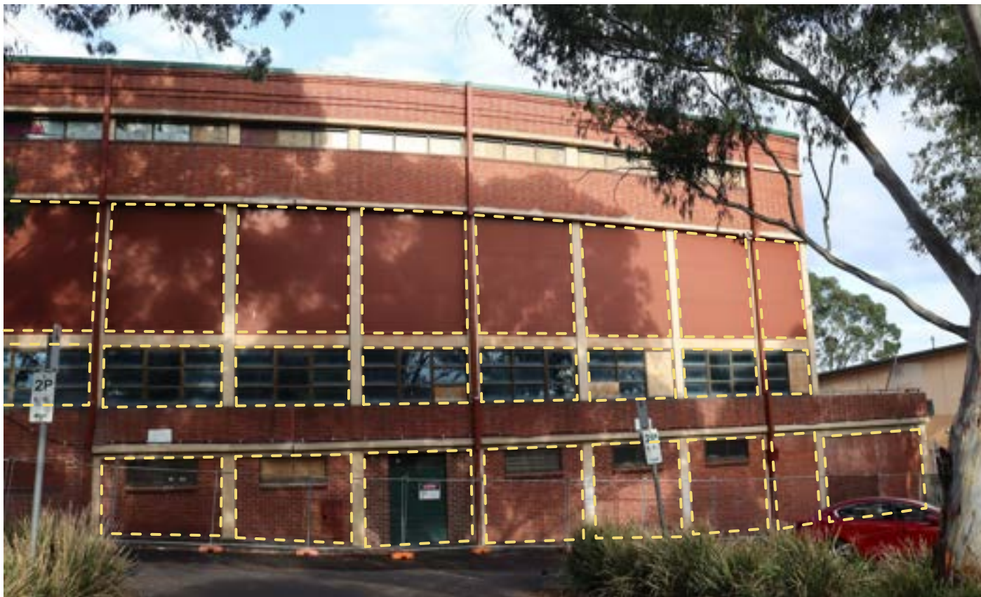
Figure 26: Rear west elevation of the grandstand with infill of previously open spans indicated by yellow dash
