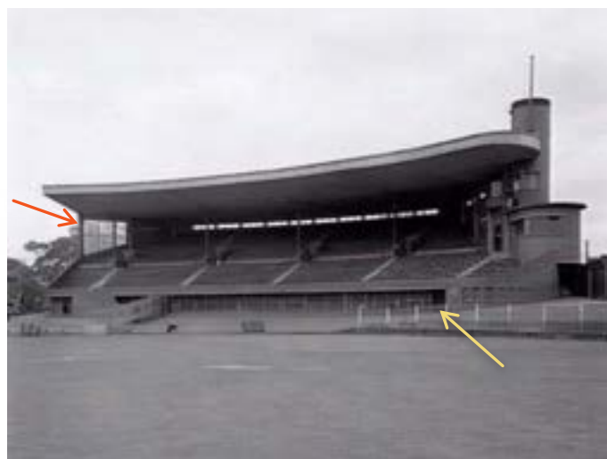
Figure 14: c1956 Grandstand from the east, showing seating area and front elevation - note the open/permeable section (orange arrow) to the south of the grandstand seating area and the northern extent of the covered way (yellow arrow) – along with the horizontal high level windows, these have been infilled (Lyle Fowler, SLV, H902.20/5896)
