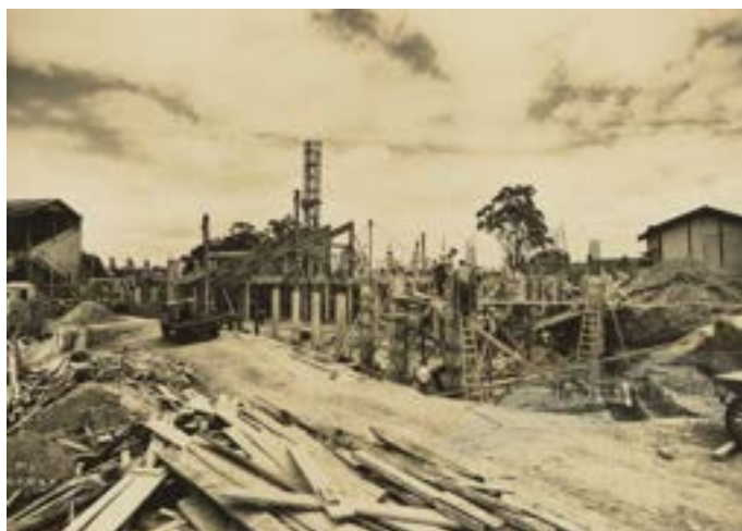
Figure 8: 12 February 1938, Construction of the grandstand at Glenferrie Oval (Edwin G Adamson, SLV, H2017.337/52)
