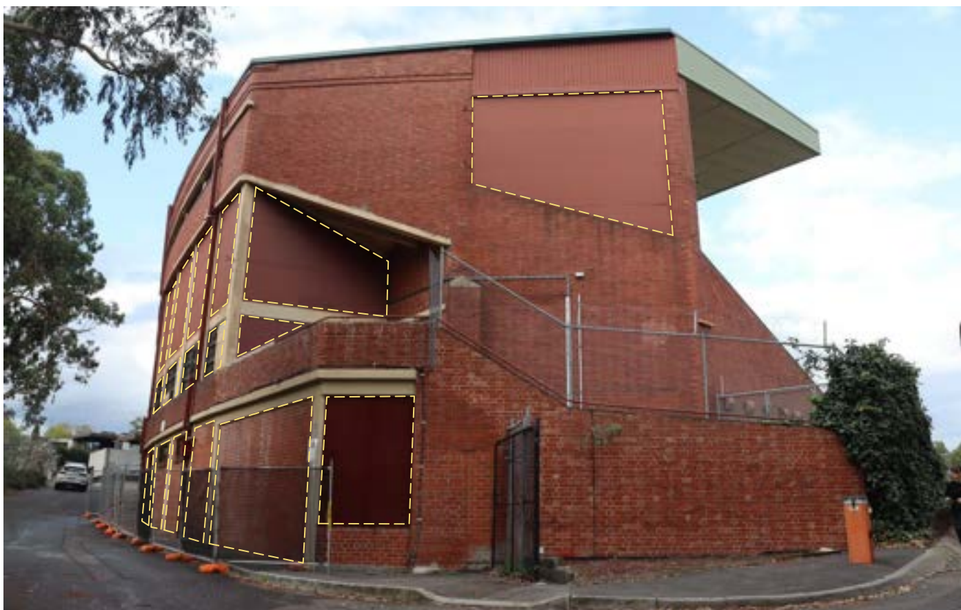
Figure 30: Southern elevation of grandstand, note the red-brown metal infill cladding (indicated by dash) at first, second, and third floor levels as well as bricks bound by yellow concrete columns and beams denoting infilled areas
