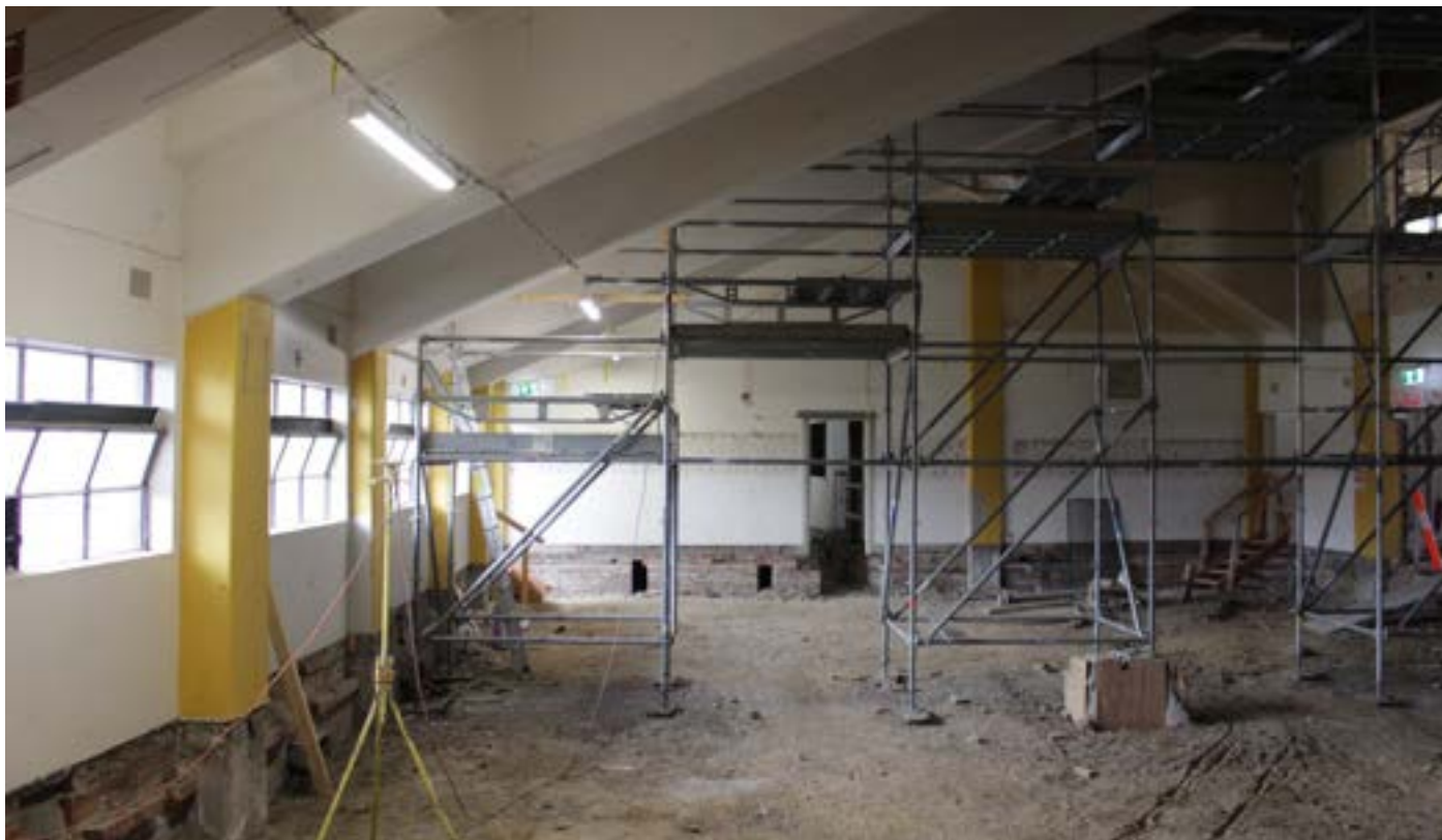
Figure 31: Undercroft interior showing impact of structural works with the removal of interior flooring
