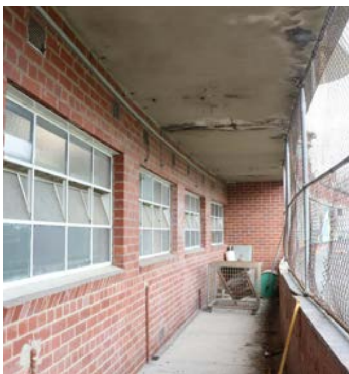
Figure 43: Steel framed multi-paned windows to the covered way
