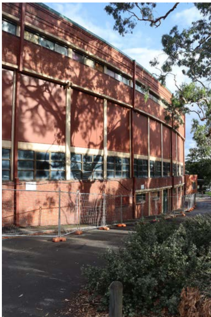
Figure 24: Rear, west elevation of the grandstand showing brickwork, decorative banding, columns and beams, openings; promenade level's former openings at double height infilled by brown metal cladding. Note the downwards slope of the ground across the building.
