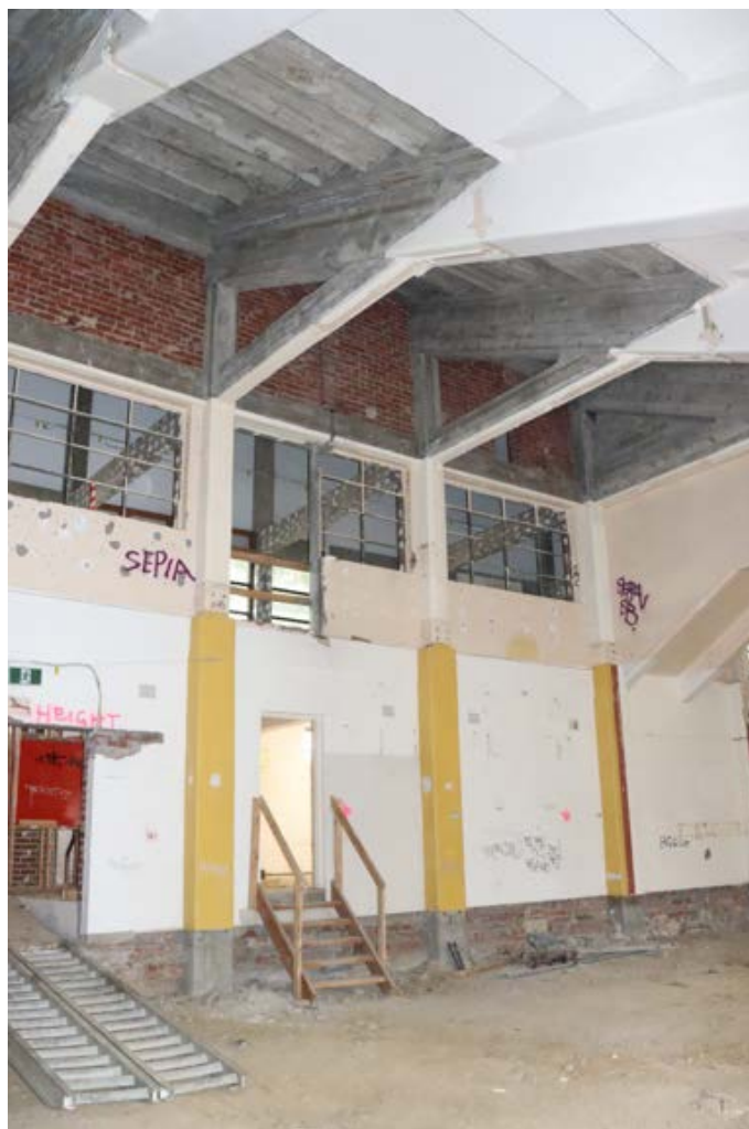
Figure 28: Double height space of the former training room (ground level) with windows to the promenade above (first floor)
