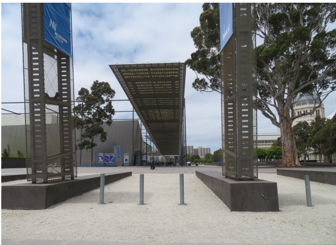
Figure 17 View of the Melbourne Museum and Museum Plaza from Rathdowne Street
