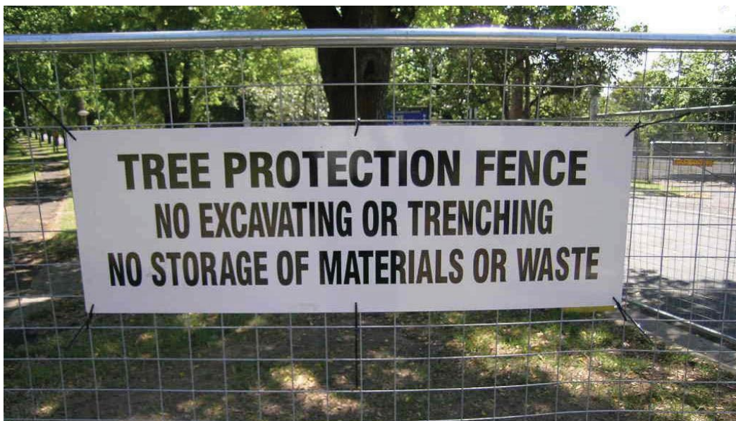
Figure 8: Example of a TPZ warning sign clearly displayed on TPZ fencing
