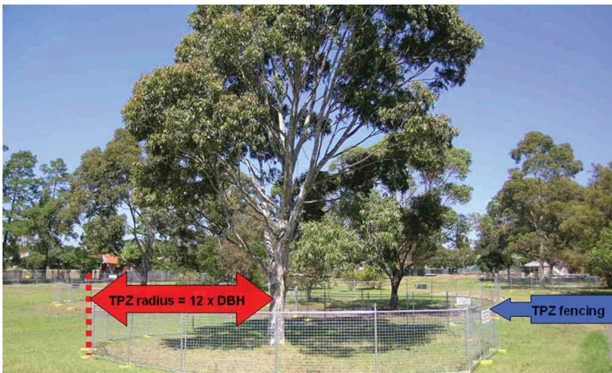
Figure 7: TPZ fencing is erected around retained trees prior to site works.
