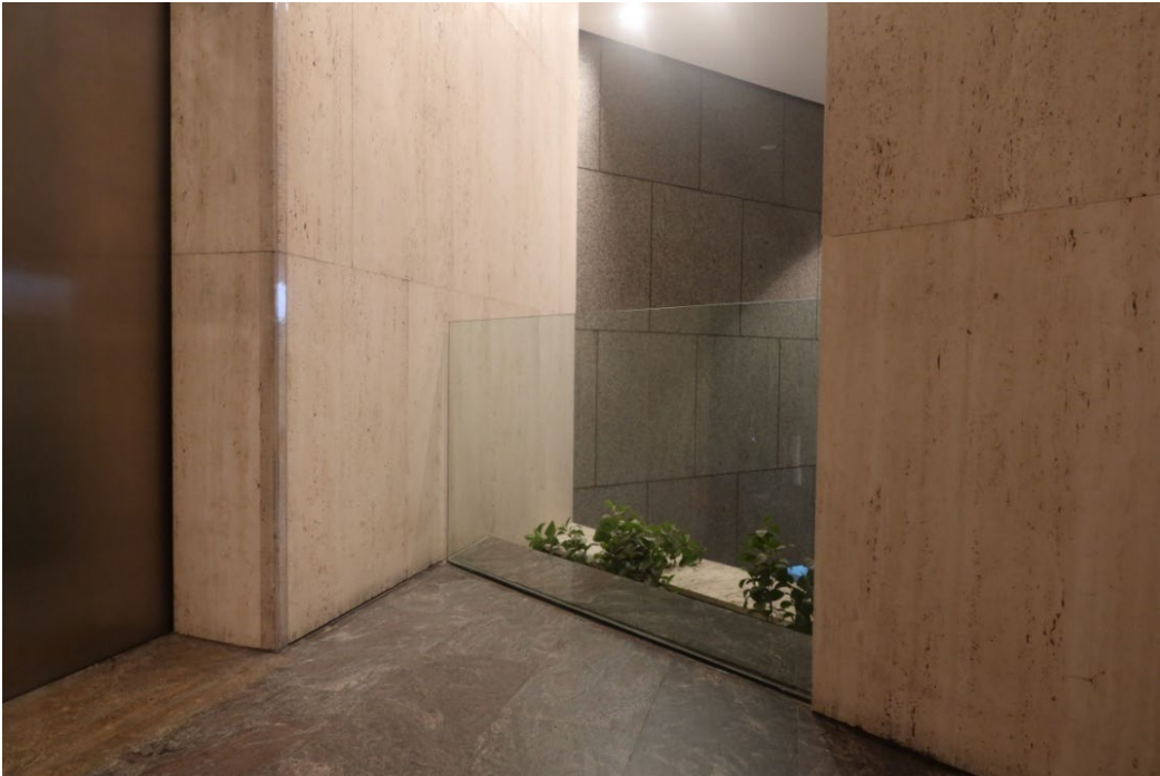
Figure 30 Planter balustrade to be removed to accommodate the new bridge
