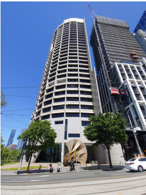
Figure 5 View of 1 Spring Street from the east in Spring Street, note the sculpture 'Shell Mace' by the American artist Charles O Perry Source: Photograph by Greg Holman
