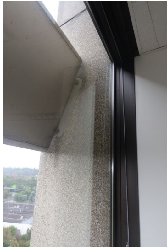
Figure 9 Detail of the position of the windows relative to the façade columns and integrated sunshades
