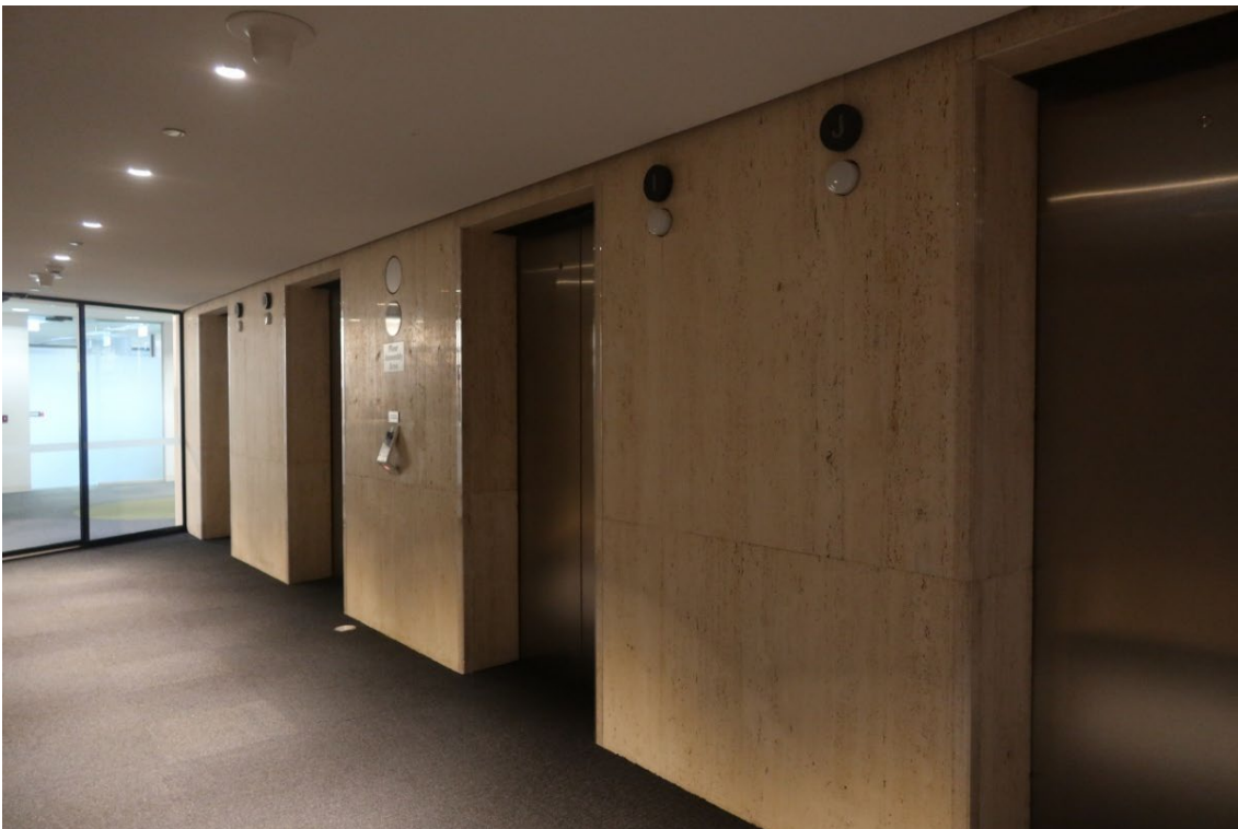
Figure 40 Travertine-clad lift lobby on Level 27, where openings to redundant lift enclosures are infilled, this would match the adjacent wall finish
