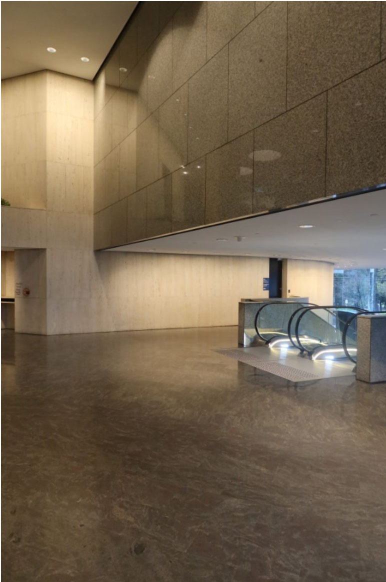
Figure 29 Another view within the void at levels 1-2 of the location of the new Level 2 bridge, escalator down to the ground floor lobby on the right
