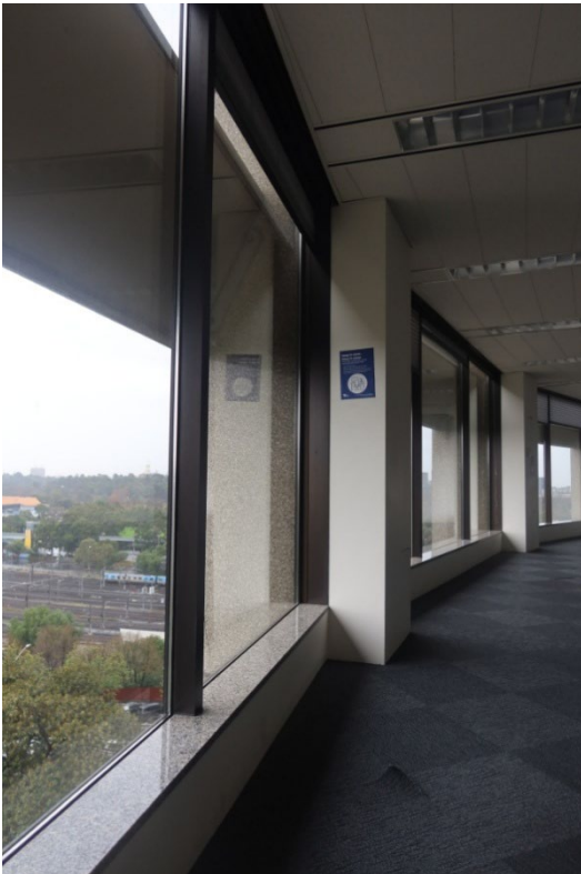
Figure 8 View of the existing fixed pane windows, note the granite-topped sills
