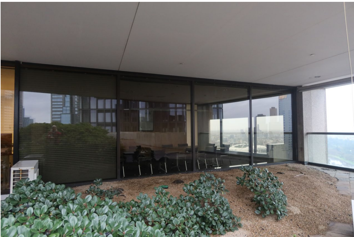
Figure 15 Existing aluminium-framed and glazed wall to the rooftop at Level 27 to be replaced
