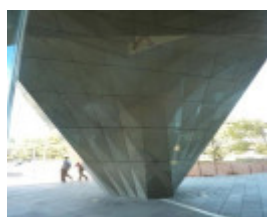
Building pier in main external plaza
