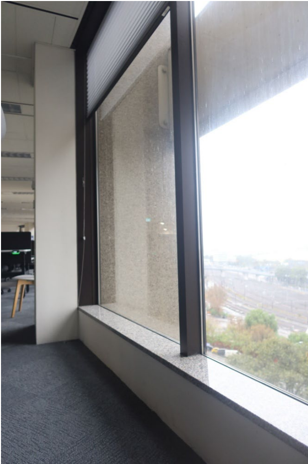
Figure 41 Existing windows and granite topped sill
