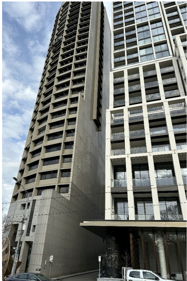
Figure 51 Recent view of the north and east elevations from Spring Street Source: Lovell Chen
