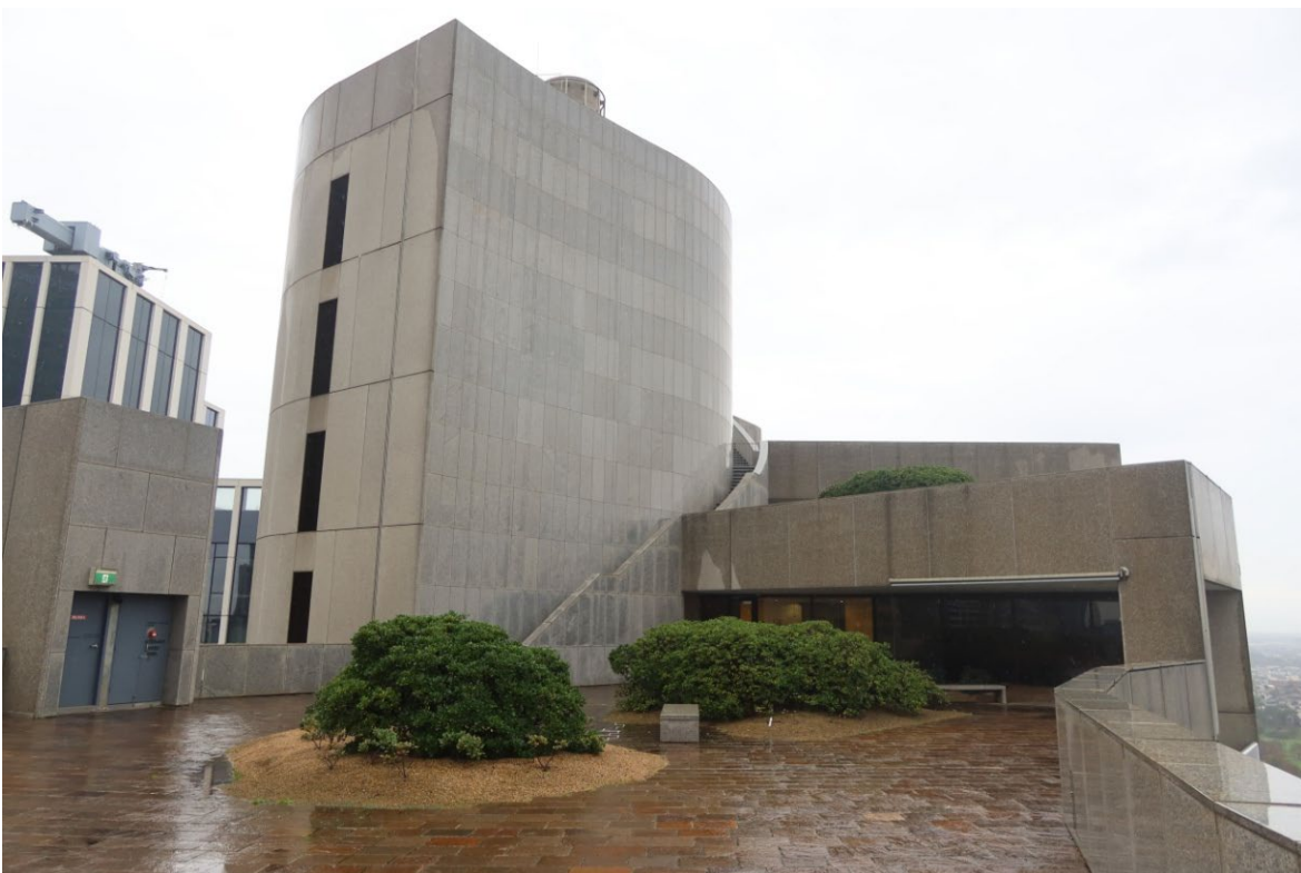
Figure 18 View on the rooftop terrace at Level 27 showing the stepped roof forms rising up (Level 28 in front and plant roofs behind), note also the recessed glazed wall to Level 27
