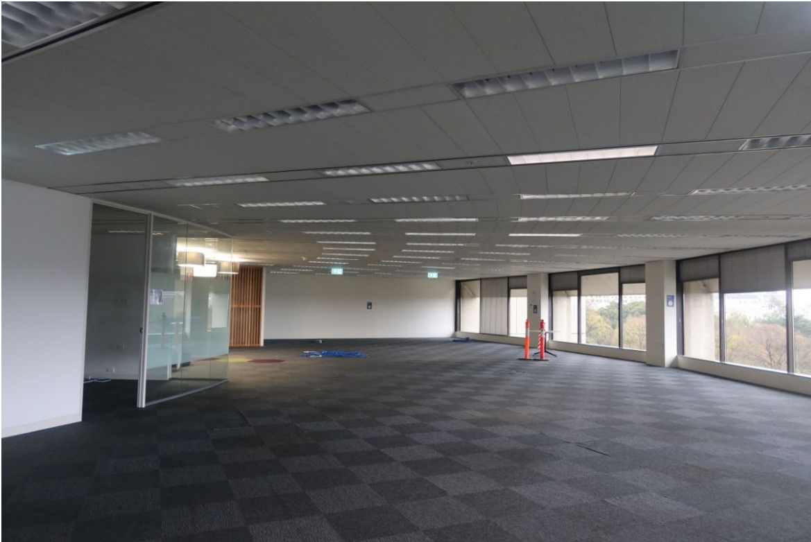
Figure 37 General view on one of the office floors (Level 6), all ceilings, flooring and partition walls and related fitout to be demolished
