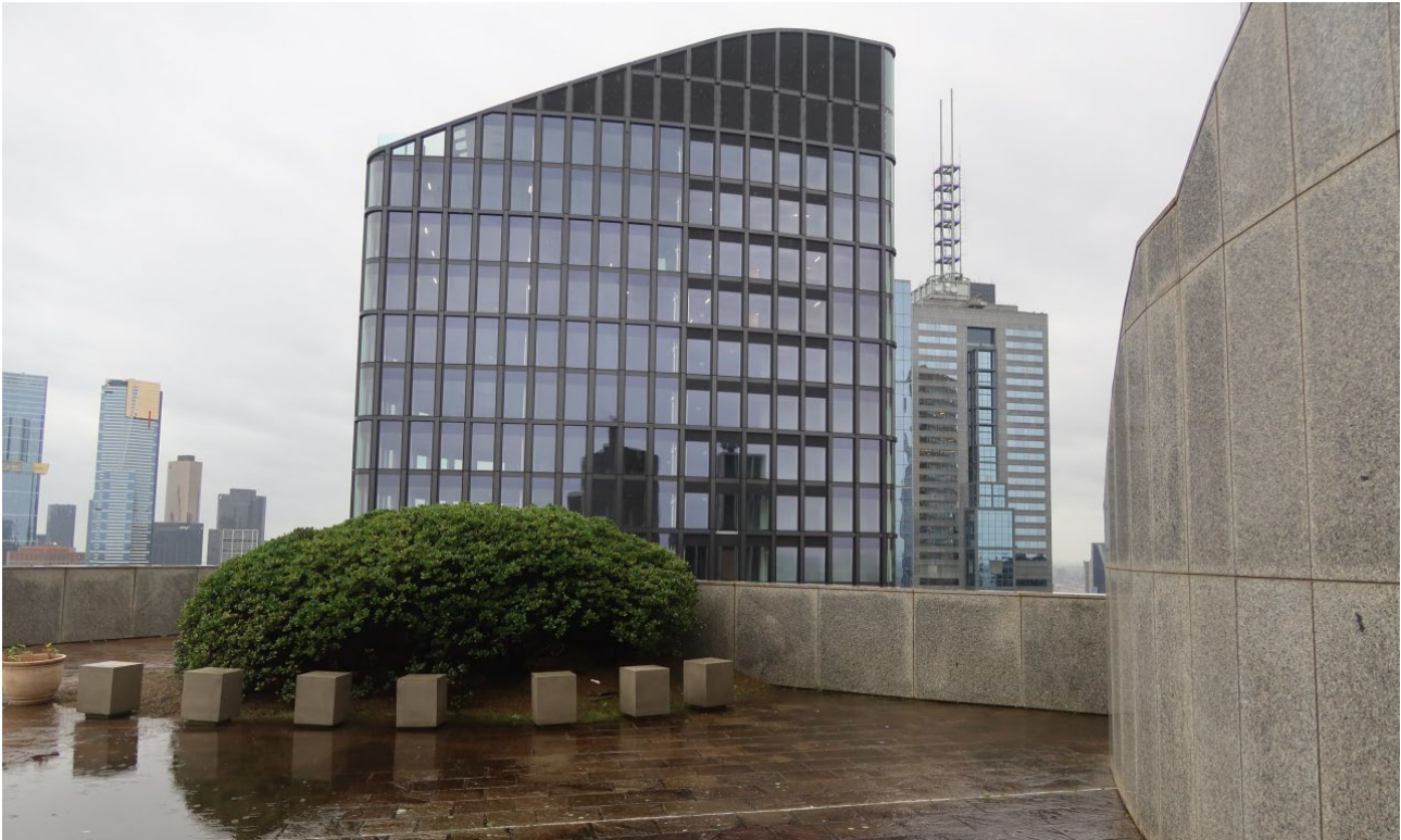
Figure 19 View of the smaller roof terrace on Level 28 looking west/north-west
