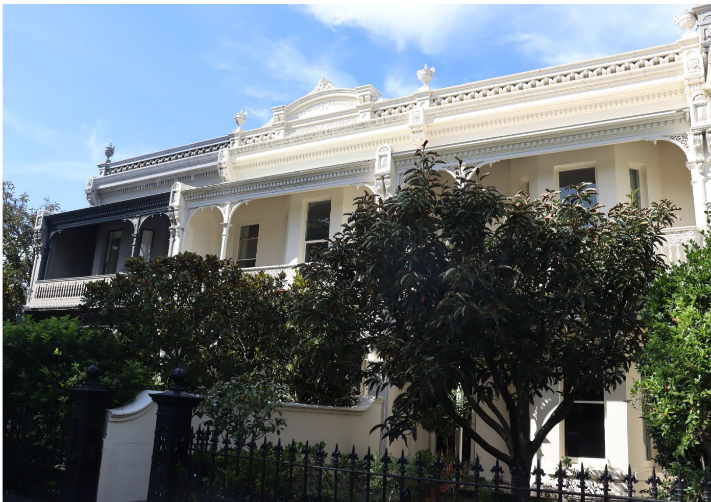
Figure 15: Belgrave Terrace showing existing façade conditions - 15 St Vincent Place (far right), and 2009 scheme applied to 11 St Vincent Place (far left)
