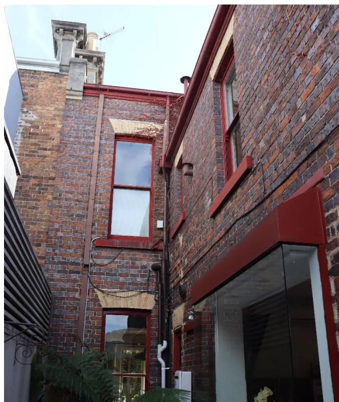
Figure 18: Configuration within light court towards original, receding form
