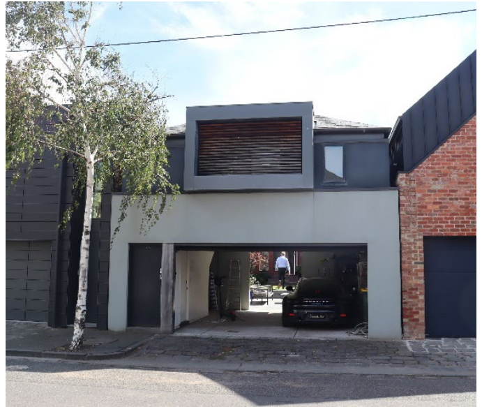
Figure 21: View from Bevan Street, looking towards the subject site (centre)
