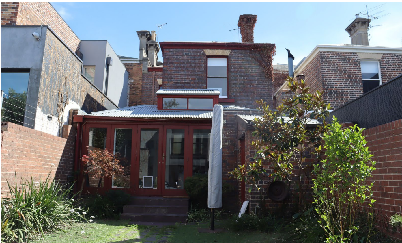
Figure 19: Main residence from the south, showing original fabric (double-storey), non-original living space addition (single-storey) and shed (to the right)
