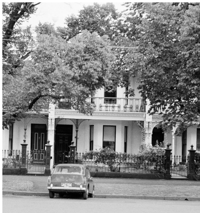
Figure 27: c1970-74, Belgrave Terrace from St Vincent Place South (no. 11 to the left, no. 13 centred, no. 15 to the right). Basalt edges to the verandah deck partially visible to residences within terrace group but obstructed at no. 15.
