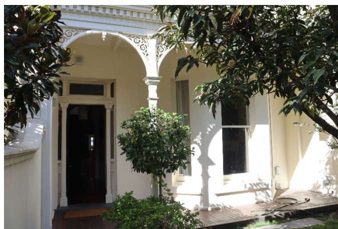
Figure 17: Entrance verandah with timber columns, decorative frieze, timber decking, and bay window.
