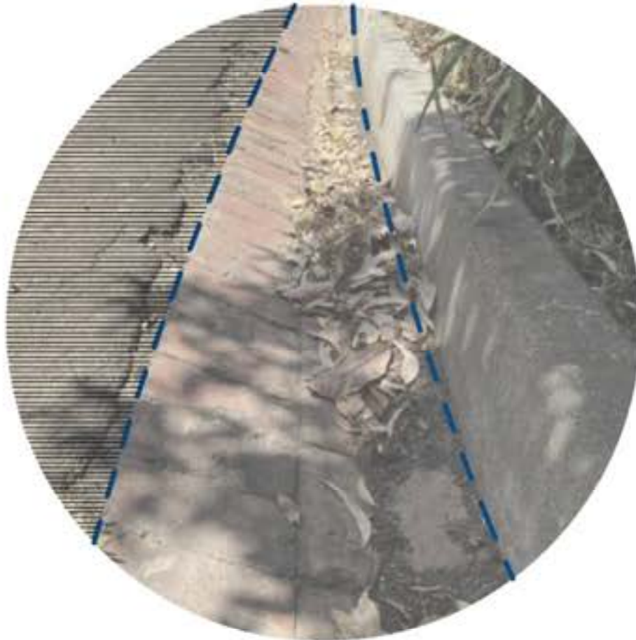
5 REMNENT BRICK SPOON DRAIN
