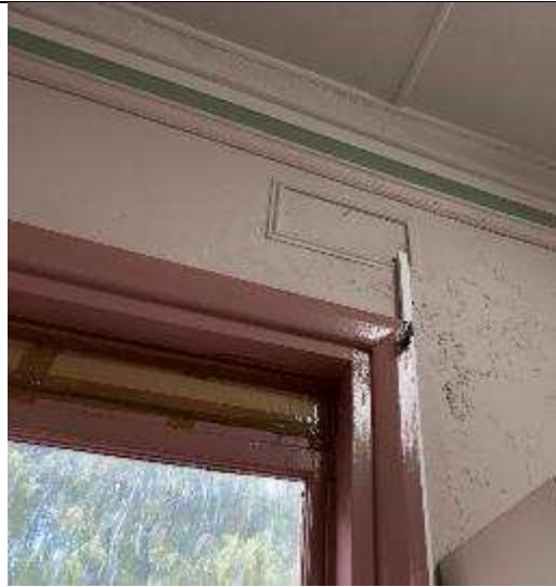
Figure 20. Apparent water damage and vent above window.
