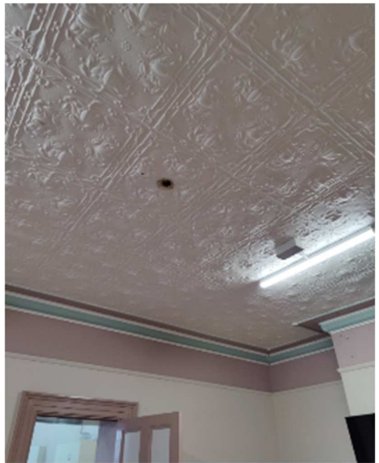
Figure 17. Detail view of the pressed metal ceiling.
