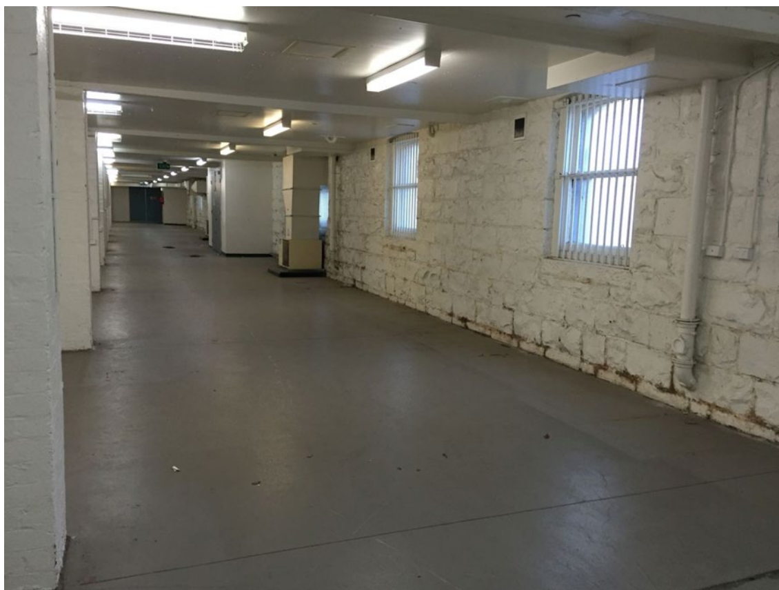
Figure 3 Interior view of basement (c. 2016) prior to recent works, note the painted interior to the bluestone basement walls and modern ceiling
