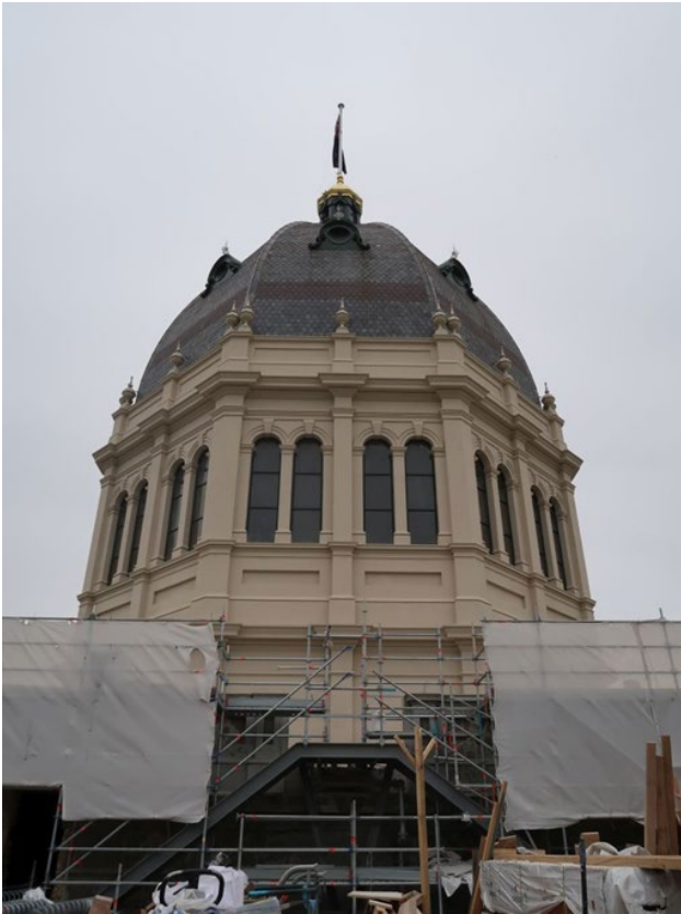
Figure 15 The dome and cupola viewed from the south at promenade level; note the dome and cupola repair works are complete and works for construction of the promenade deck are underway
