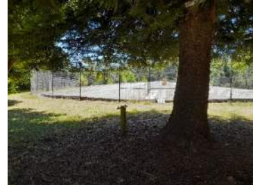
Figure 2.21 View of the reservoir behind the Day Basin (Source: GML 2022)
