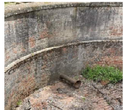
Figure 2.3 Detail view of day basin interior and pipe (GbLA, November 2023).
