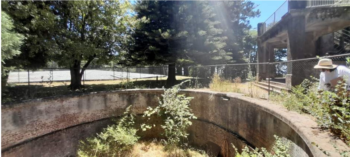
Figure 2.17 View of Day Basin fabric and bluestone capping looking north, with the oval reservoir and Pioneer Memorial Tower in the background. (Source: GML 2022)
