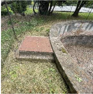
Figure 2.4 View of day basin pit cover (GbLA, November 2023).
