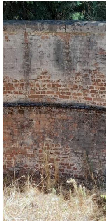
Figure 2.19 View of the Day Basin's brickwork. (Source: GML 2022)
