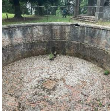
Figure 2.5 View of day basin interior and pipe (GbLA, November 2023).
