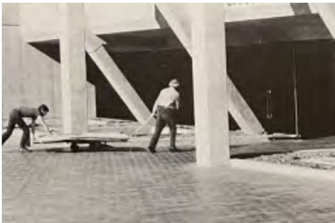
Figure 5 1980 image of the front of the building showing original (brick) paving in the forecourt along with the shallow garden beds.
