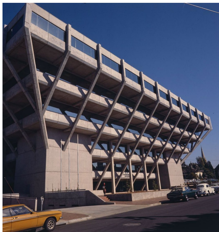
Figure 3 State Government Office, Geelong, 1979, showing original paving and early planting to northern facade. |Source: NAA.
