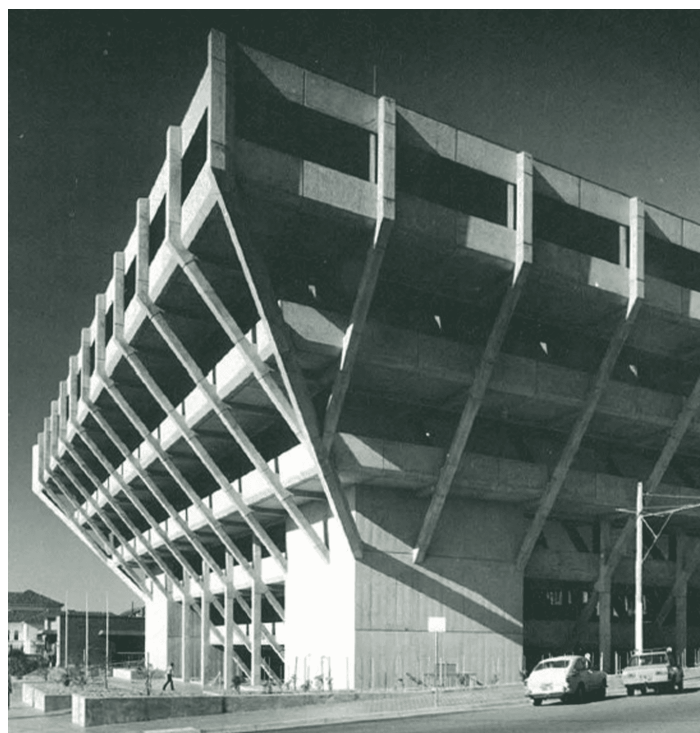
Figure 4 1979 image of the building showing early planning along Little Malop and Fenwick Streets. | Source: Buchan.
