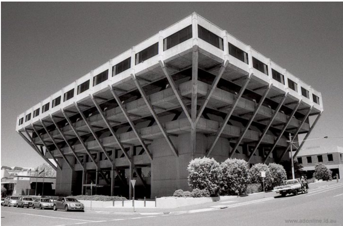
Figure 8 c.2010 view of the State Government Offices Geelong showing established trees along the western boundary of the site.
