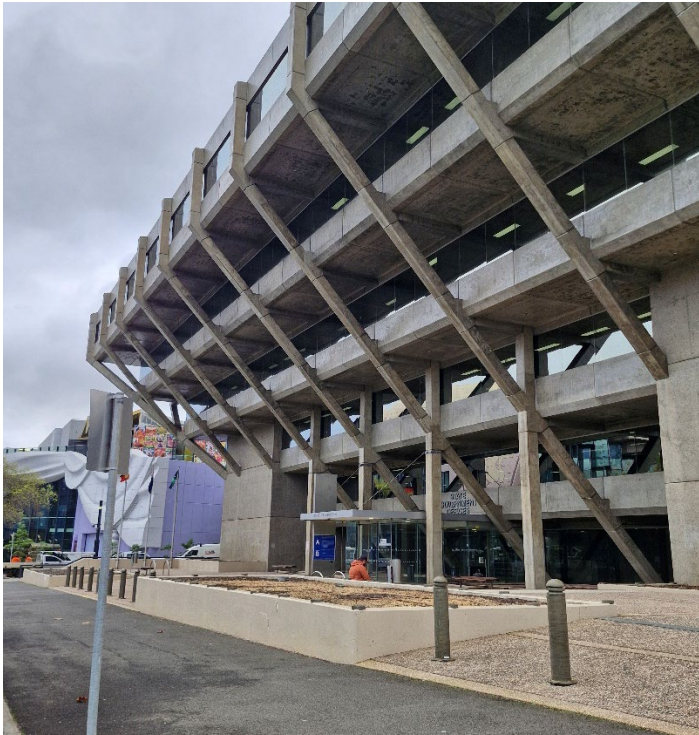
Figure 13 View of the Little Malop Street (north façade) plaza area noting large concrete planter and existing bollrds.
