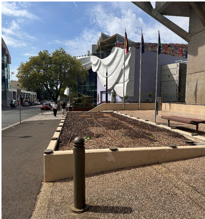
Figure 15 Detail of existing planter in Little Malop Street plaza area showing defensive protrusions to tops of planter walls.
