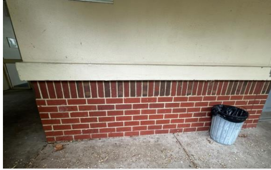
Figure 22: Detail of non-original 1990s School Building wall (eastern wall of internal courtyard). Lower portion constructed with red bricks in a stretcher bond, capped with clinker brick soldier course. Source NBRS, 2024.
