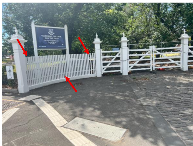
Figure 33 : Image of the angled gateway to the intersection of St Kilda Road and High Street, with the inconsistent gaps between palings indicated by an arrow. Source: NBRS 2025
