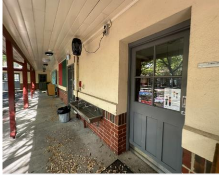
Figure 21: Detail of original 1928 School Building wall (western wall of internal courtyard). Lower portion constructed with red bricks in a Flemish bond, capped with clinker brick soldier course. Source NBRS, 2023
