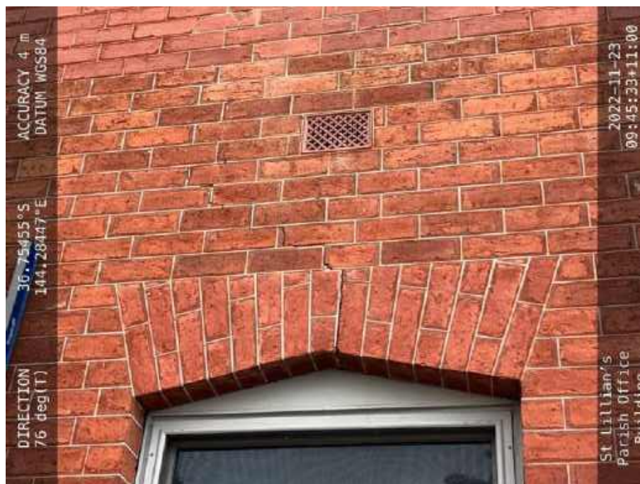
Photo 18 – Typical cracking to other walls of the subject building caused by historical foundation movements.
