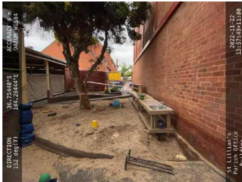
Figure 5 – Sand pit constructed against North-East wall of building allowing for rainfall to seep into soils against building.
