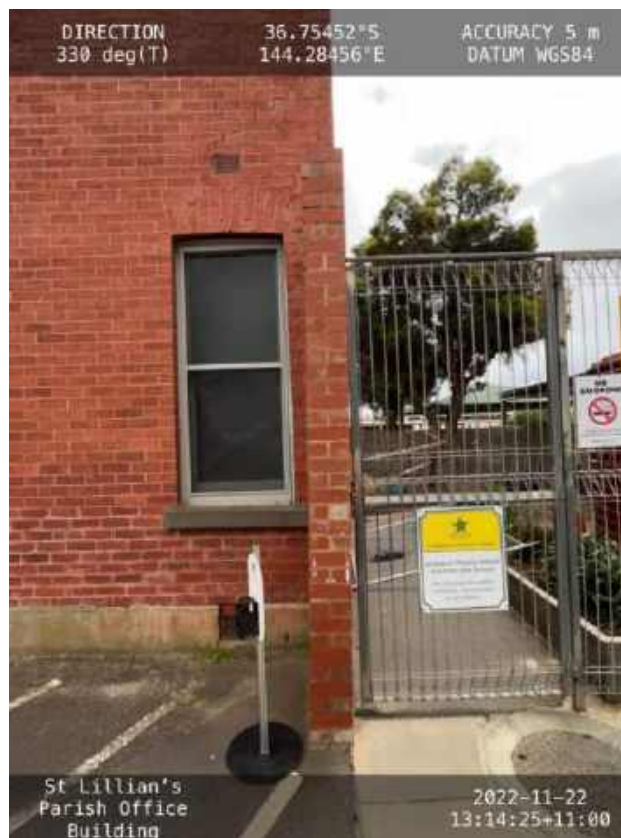
Figure 5: Blade wall significantly out-of-plumb.
