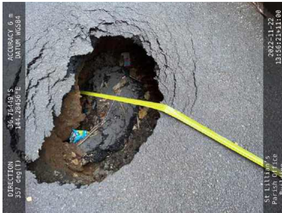
Photo 5 – Sink hole prior to excavation.
