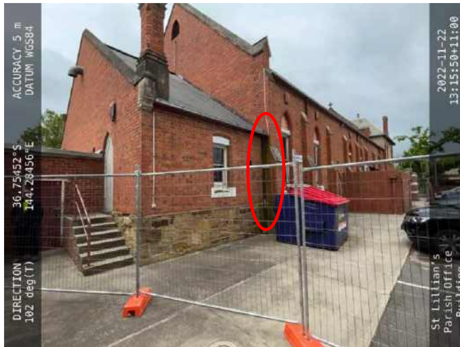
Photo 17 – Existing St Killian's Primary School, school hall building. Note possible defective down pipe noted to circled location.
