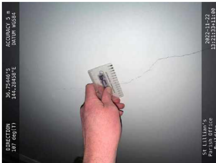
Photo 15 – Typical cracking to hard plaster to interior of White House building.
