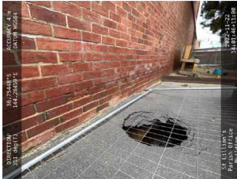
Figure 3 – Sink hole to North-East wall of building located within St Killian's Primary School site.
