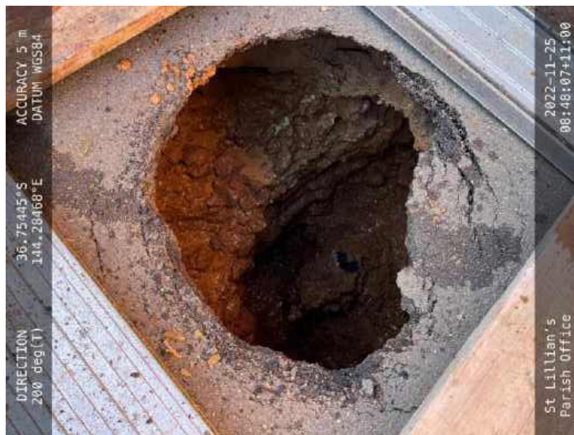
Figure 4 – Sink hole to North-East wall of building after hydro excavation.
