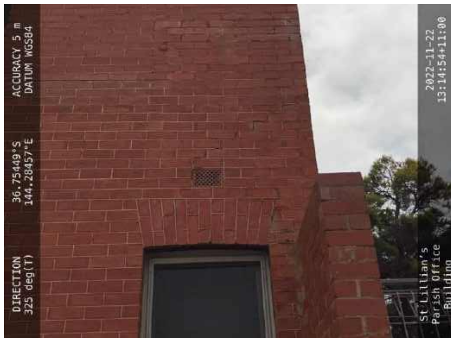
Photo 11 – Stepped cracking damage to Southern corner of White House building.
