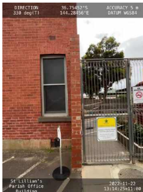
Photo 8 – Blade wall to Southern corner of building with significant out-of-plane rotations.
