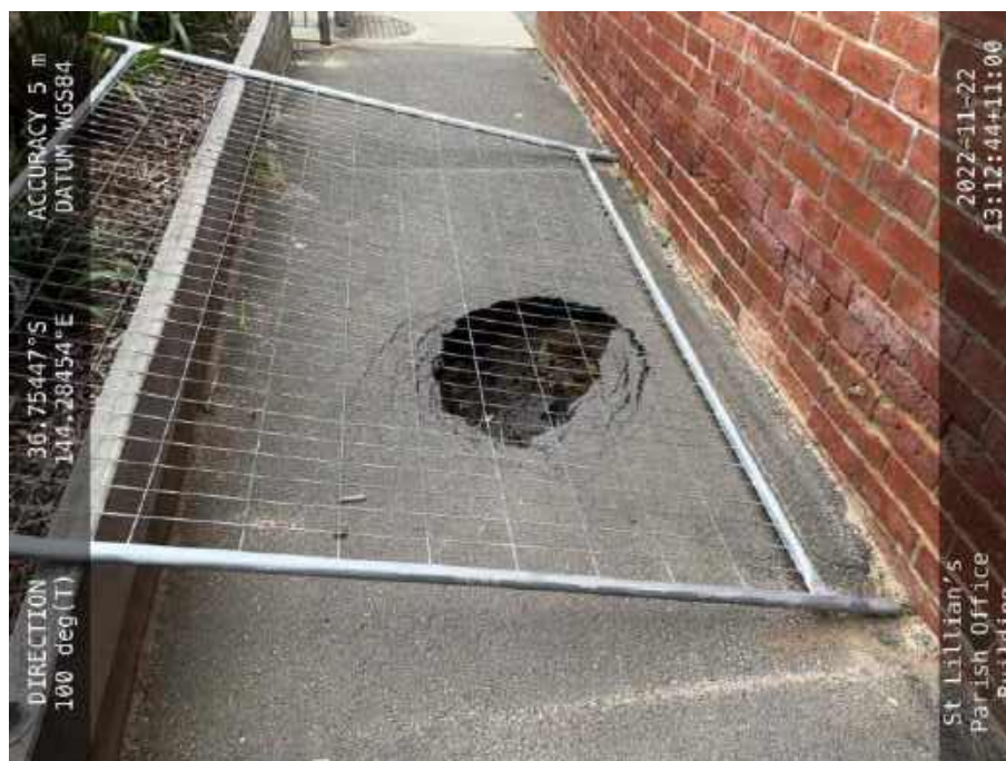
Photo 4 – Sink hole condition at first inspection.
