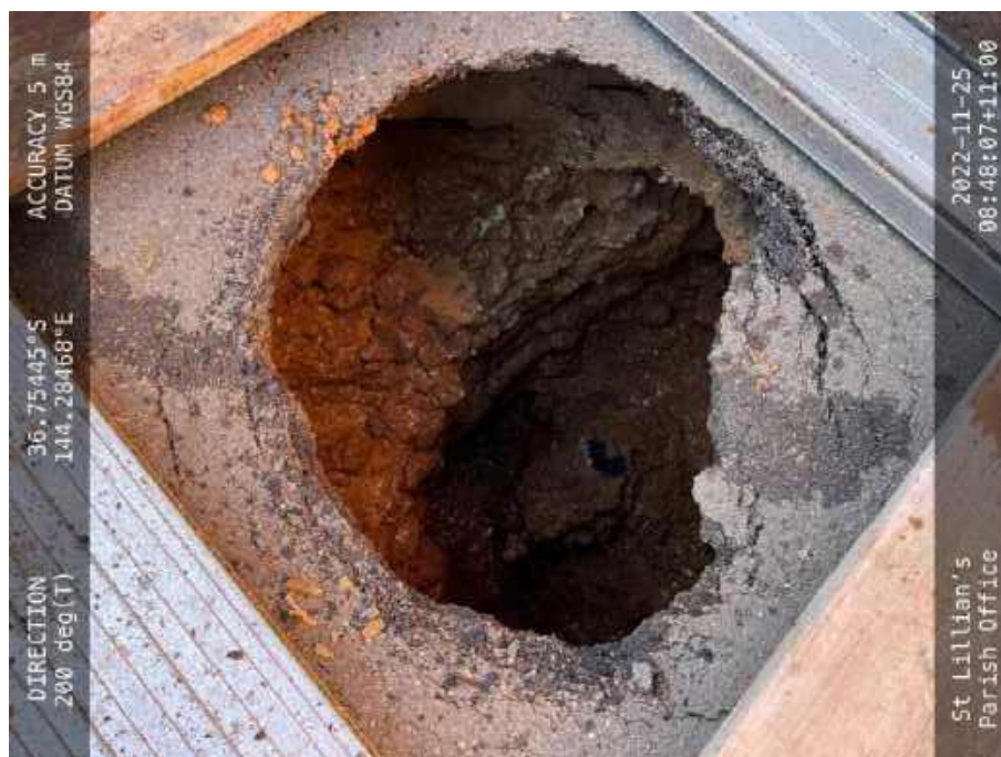
Photo 6 – Sink hole following hydro excavation.
