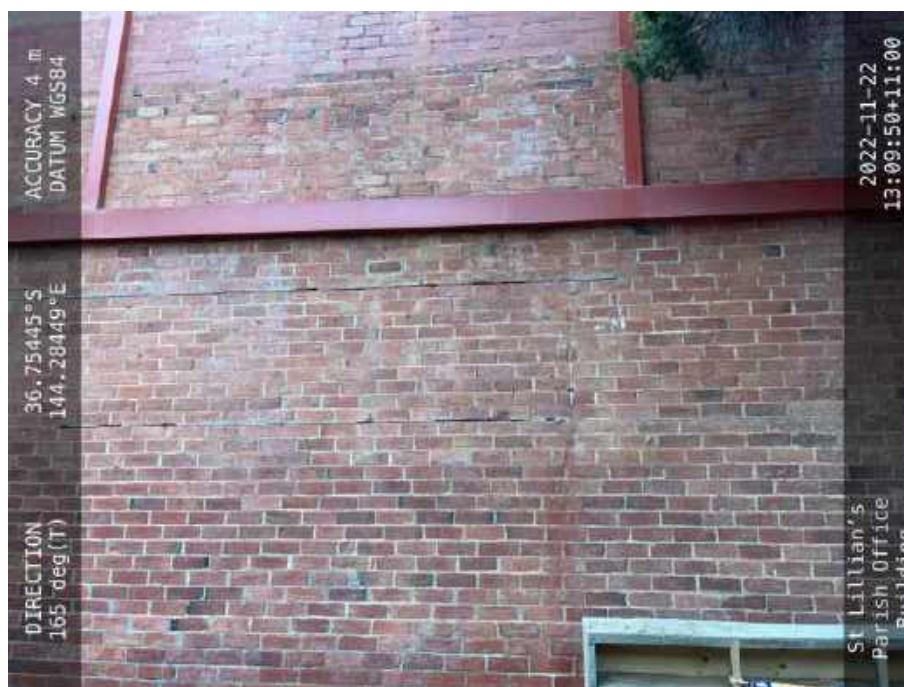
Photo 2 – Existing condition of brick wall in proximity to sink hole. Note cracking.
