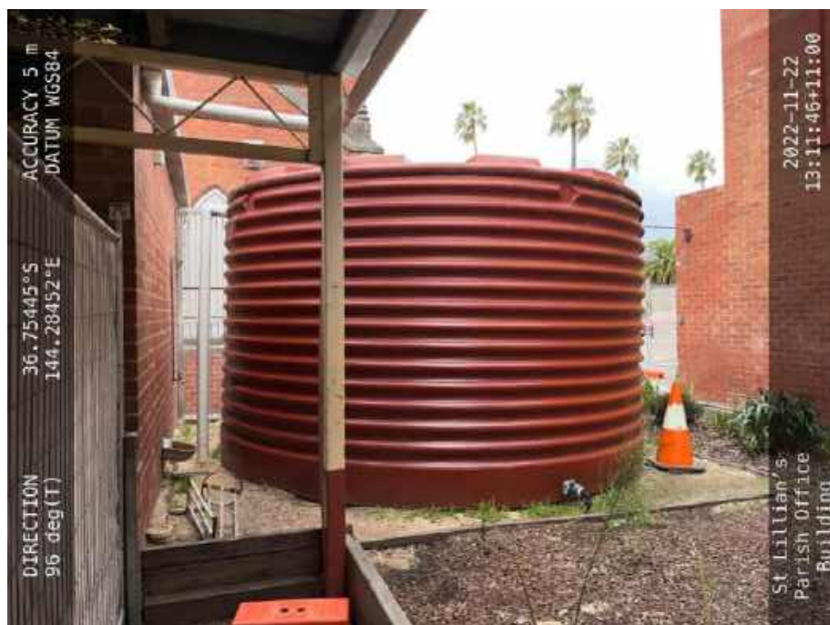
Photo 12 – Rainwater tank found not to be full at the time of inspection. Outlet valve to base of tank also found not to be fully shut.
