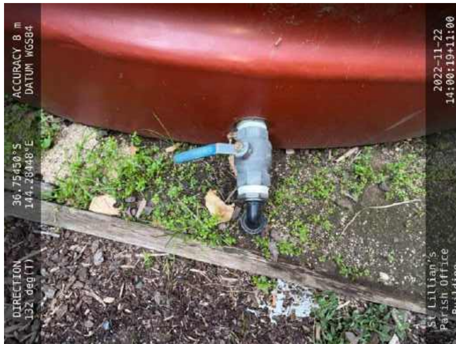
Photo 13 – Damp soil was found to the base of the tank outlet.
