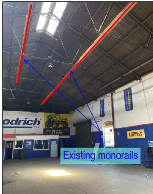
Figure 17 Monorails at the underside of roof truss bottom chords
