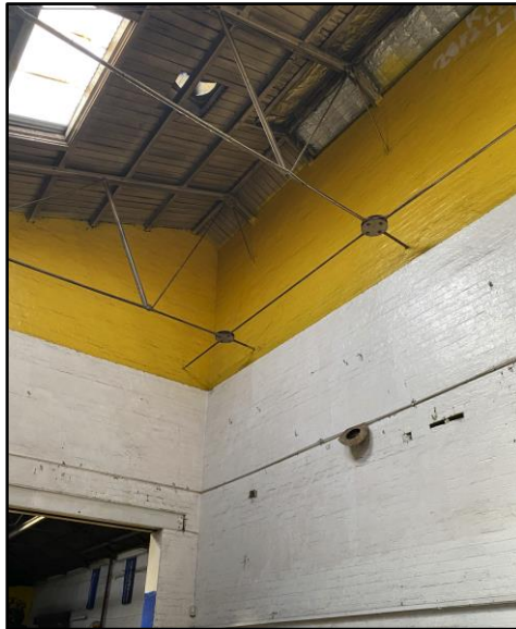
Figure 6 Roof truss bottom chord concealed inside masonry walls
