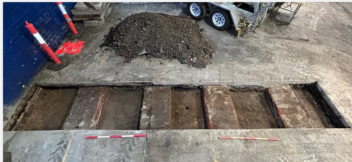
Figure 46: Overview of Trench 2 post removal of concrete and bitumen <2000> with tops of brick walls for cable pits exposed. View to the west.
