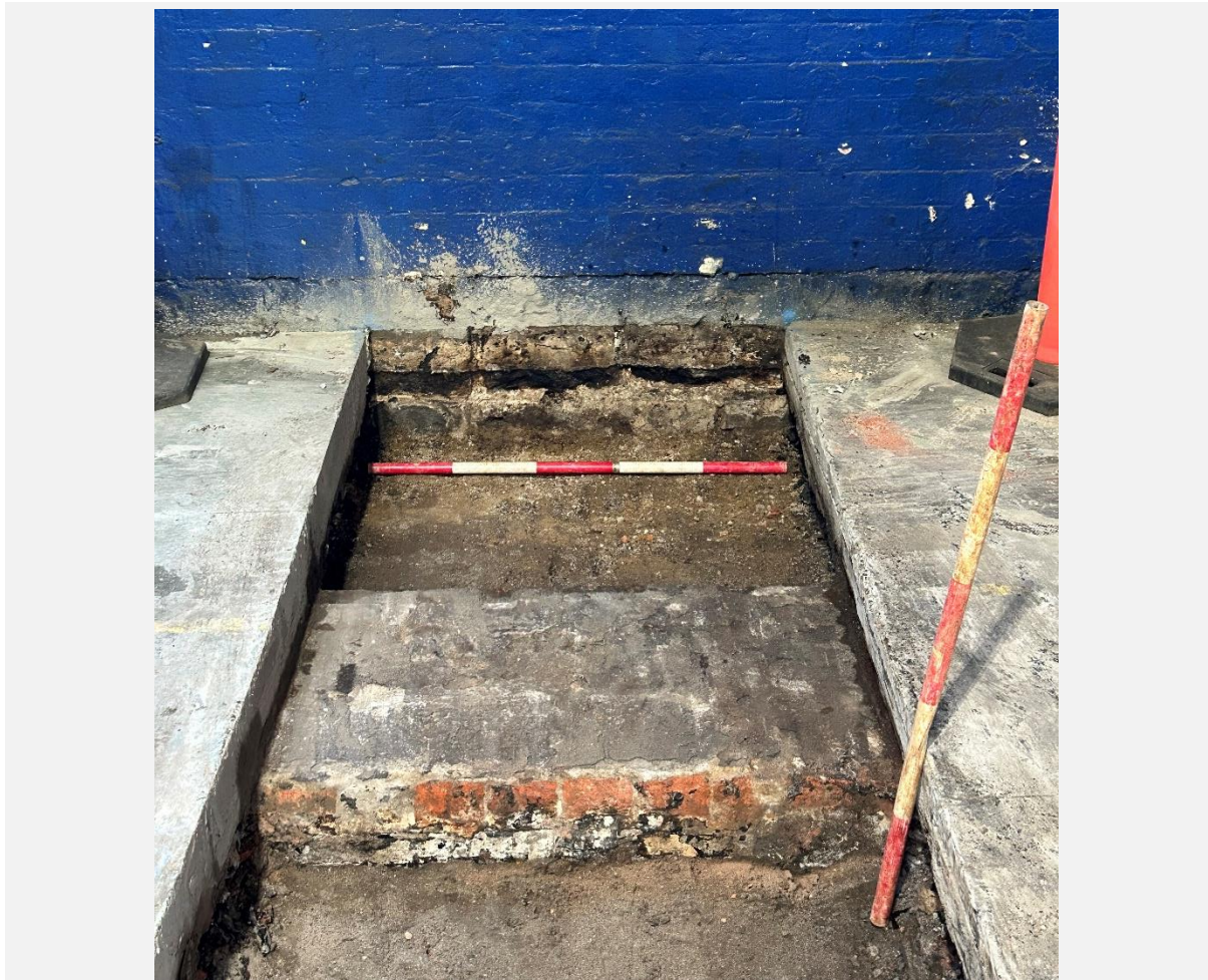
Figure 47: View of southern external wall and basal footing <2010> along with cable pit brickwork <2008>. View to the south.
