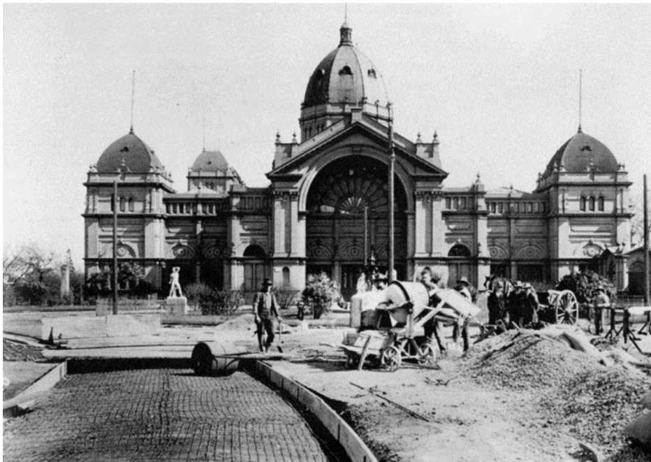
Figure 83 Pouring concrete for the Nicholson Street entrance driveway at the Exhibition Building in the 1920s. Note that the French Fountain and statuary dating from the Great Exhibitions are still clearly visible Source: Reproduced from Victorian Icon: The Royal Exhibition Building Melbourne
