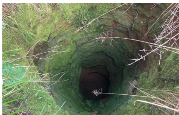
Figure 2.4.1: 10 metre deep round alluvial mining shaft, Allen's Flat, Buckland. August 2023.
