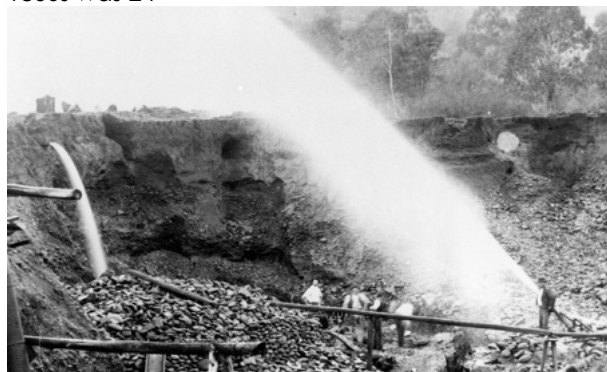
Figure A3.3: High-pressure hydraulic sluicing on the Lower Buckland. Geological Survey of Victoria.
