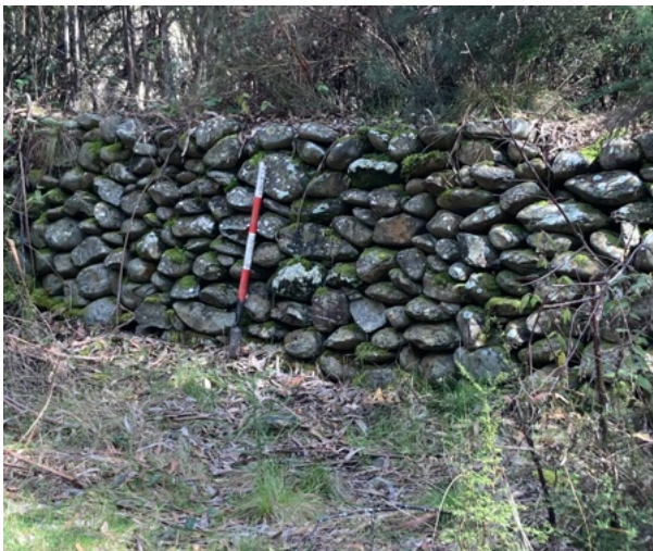
Figure 2.2.7: Cobble-stone retained elevated water race that directly fed flume over waterwheel of Paulussy's battery (200mm divisions on pole)
