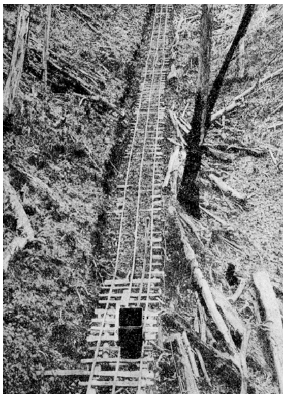
Figure 2.3.3: A typical mountain tramway, showing partially built on ground surface and partially into ground. Footprint would be similar to that of the Nelson Tramway. Big Gun incline tramway at Harrietville, c1903. Geological Survey of Victoria.
