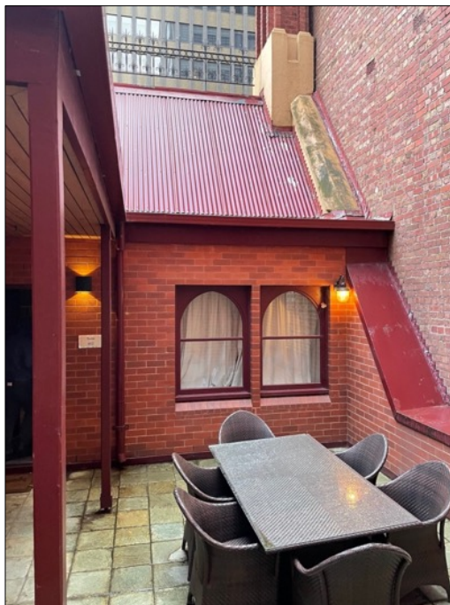
Figure 70 (left) View from roof terrace showing the rear of the attic storey roof with Colorbond cladding.
