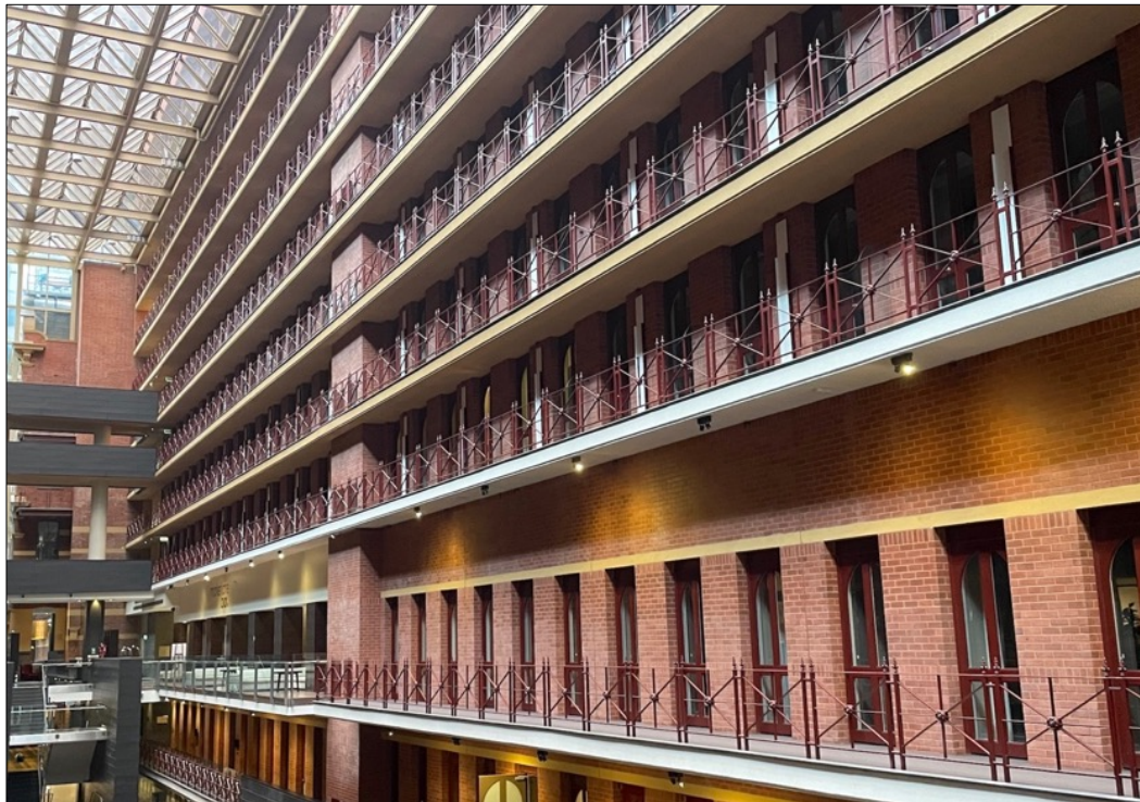
Figure 75 The west elevation of the 1980s rear wing.
