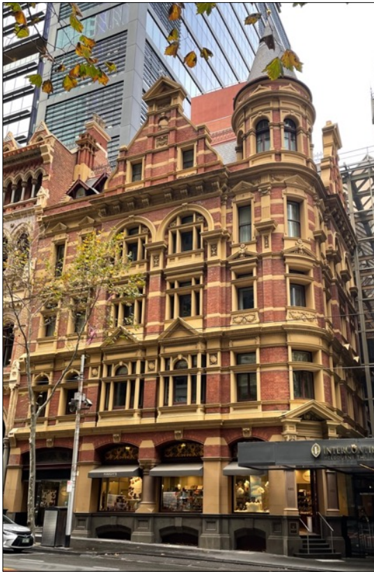
Figure 66 (left) Winfield Building Collins Street façade.
