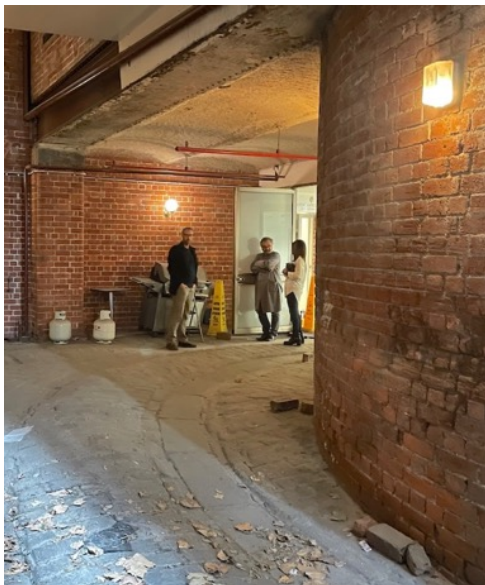
Figure 60 (left) The northern end of the subway passing under the Rialto Building. Note vaulted Traegerwellblech ceiling sprayed in vermiculite. Figure 61 (right) The curved brick wall in the subway, marking the point where the subway returned along the east elevation.
