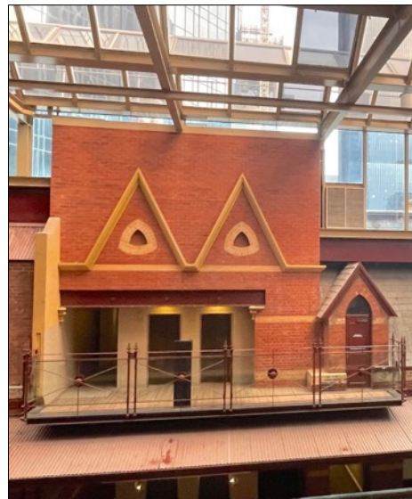
Figure 45 (right) Lift overrun, north lift shaft, with gable detailing referencing the twin gable parapets over the south lift shaft – added as part of the 1980s works.
