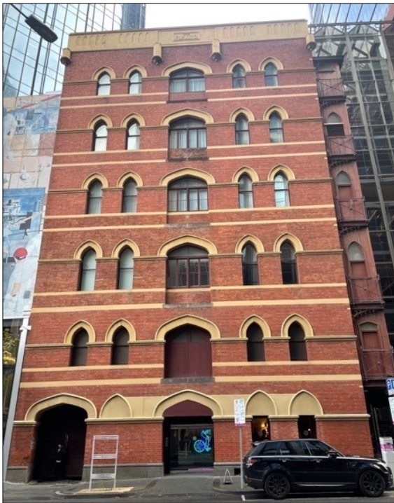
Figure 48 (left) Flinders Lane elevation. Note most of the central door openings for loading and unloading goods have been fitted with window frames.
