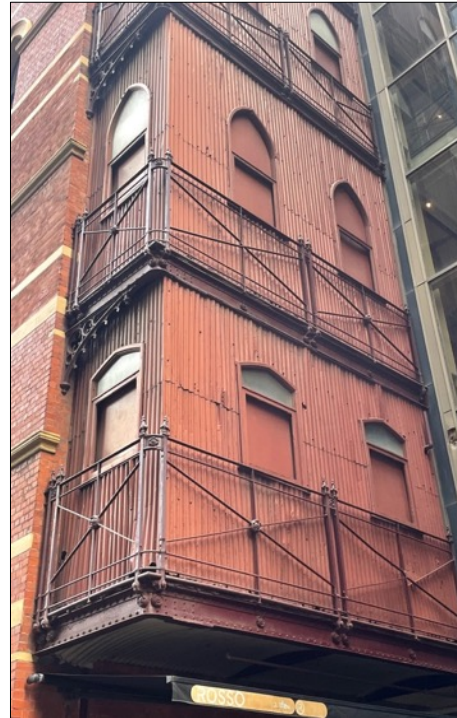
Figure 48 (left) Flinders Lane elevation. Note most of the central door openings for loading and unloading goods have been fitted with window frames.
