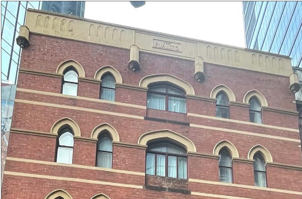
Figure 52 Current photograph with rendered parapet addition presumably dating from the 1980s works.
