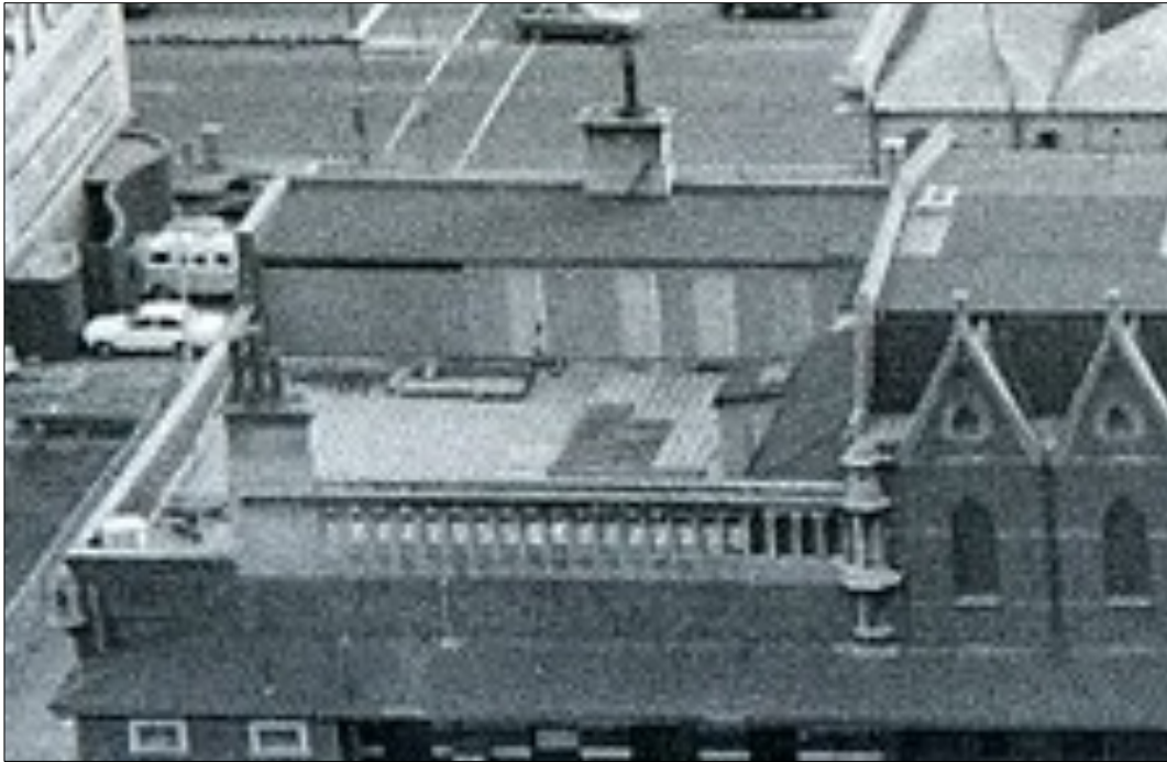
Figure 53 Detail of a c1978 photograph showing the roof at the southern end of the Rialto Building.
