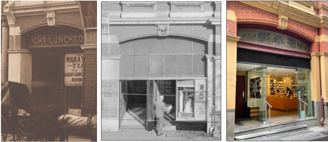
Figure 72 (left) Detail from a c1900 photograph showing shopfront at the eastern end of the ground floor façade. This is presumed to be the original shopfront configuration.
