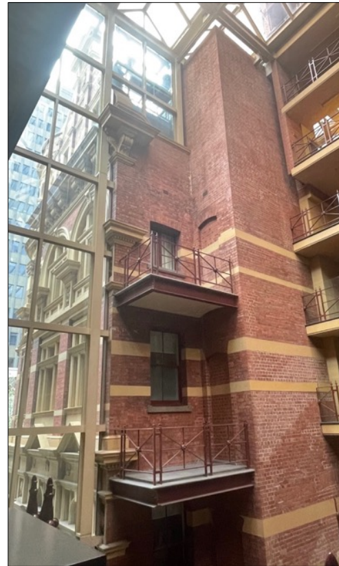
Figure 67 (right) The south-west corner of the retained heritage envelope. Note that the balconies are non-original.
