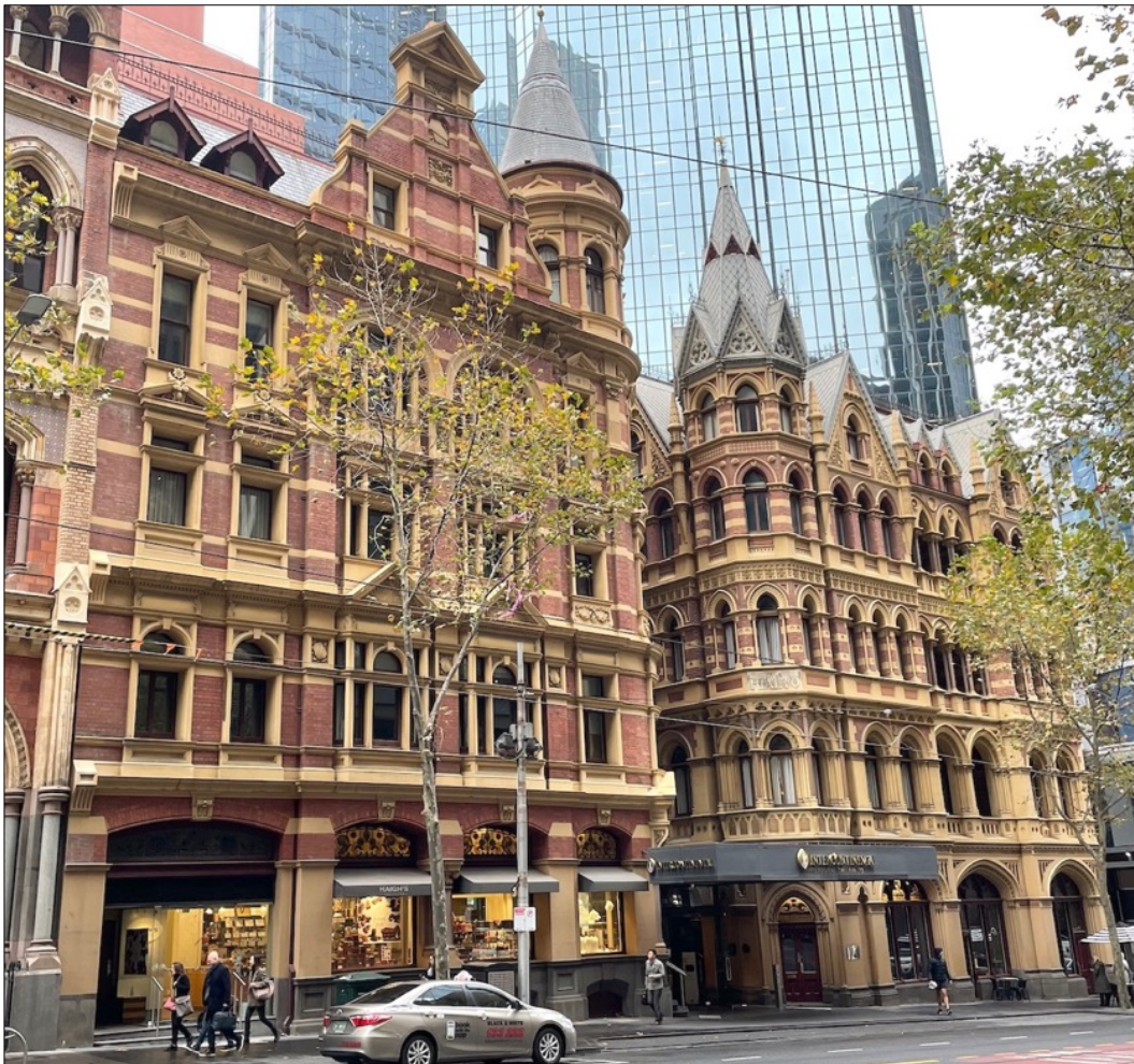
Figure 31 The Collins Street façades of the Winfield Building (left) and Rialto Building (right).
