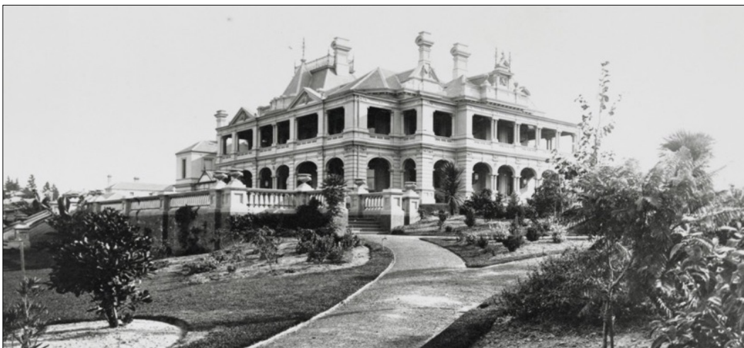
Figure 12 Stonington Mansion, c1895. Architect Charles D'Ebro. Source: State Library of Victoria.
