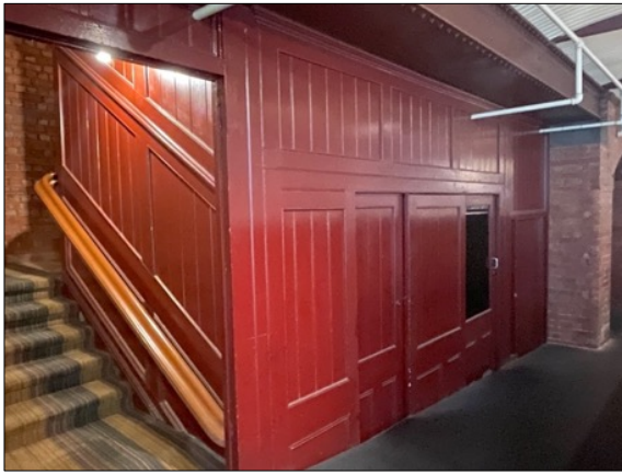
Figure 46 (left) Panelled timber lift enclosure, south lift shaft.
