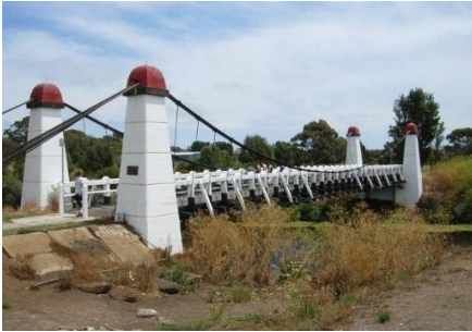
Wollaston Bridge, Warrnambool City Council
