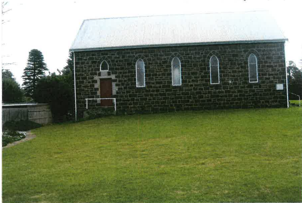
S1. e). CS east elevation - taken from east-west approx. midpoint of the land
