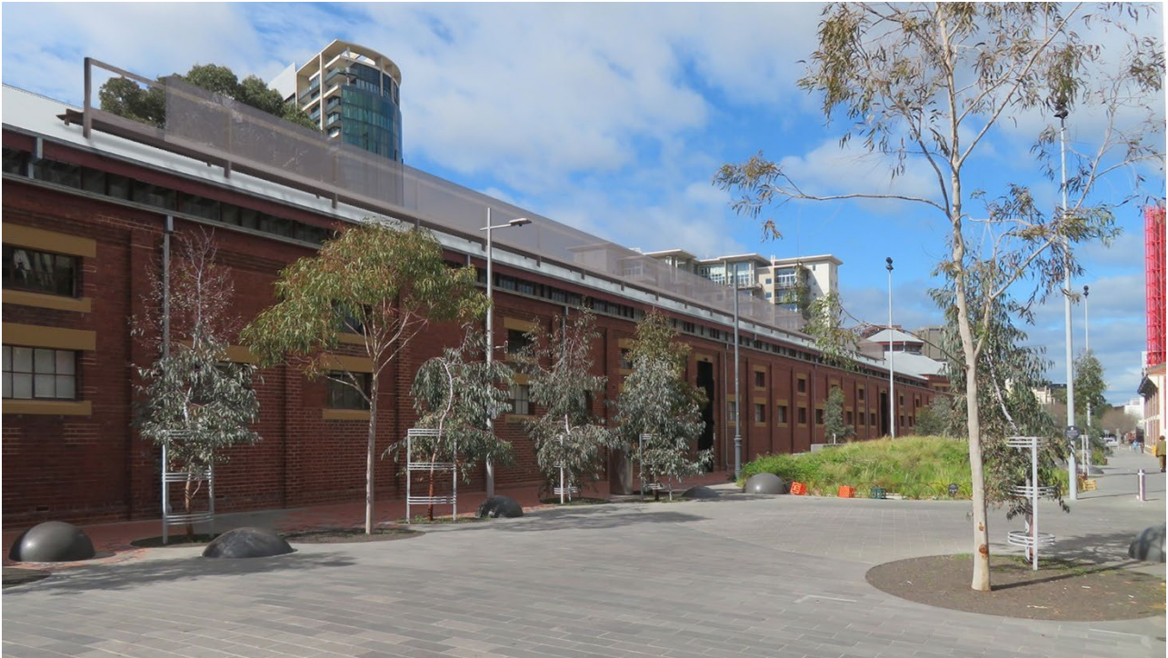
Figure 13 View of the stables with the location and outline of Artwork K and its supporting frame (specific details and transparency not shown), looking to west elevation of the stables wing from the north-west Source: Lovell Chen, September 2025
