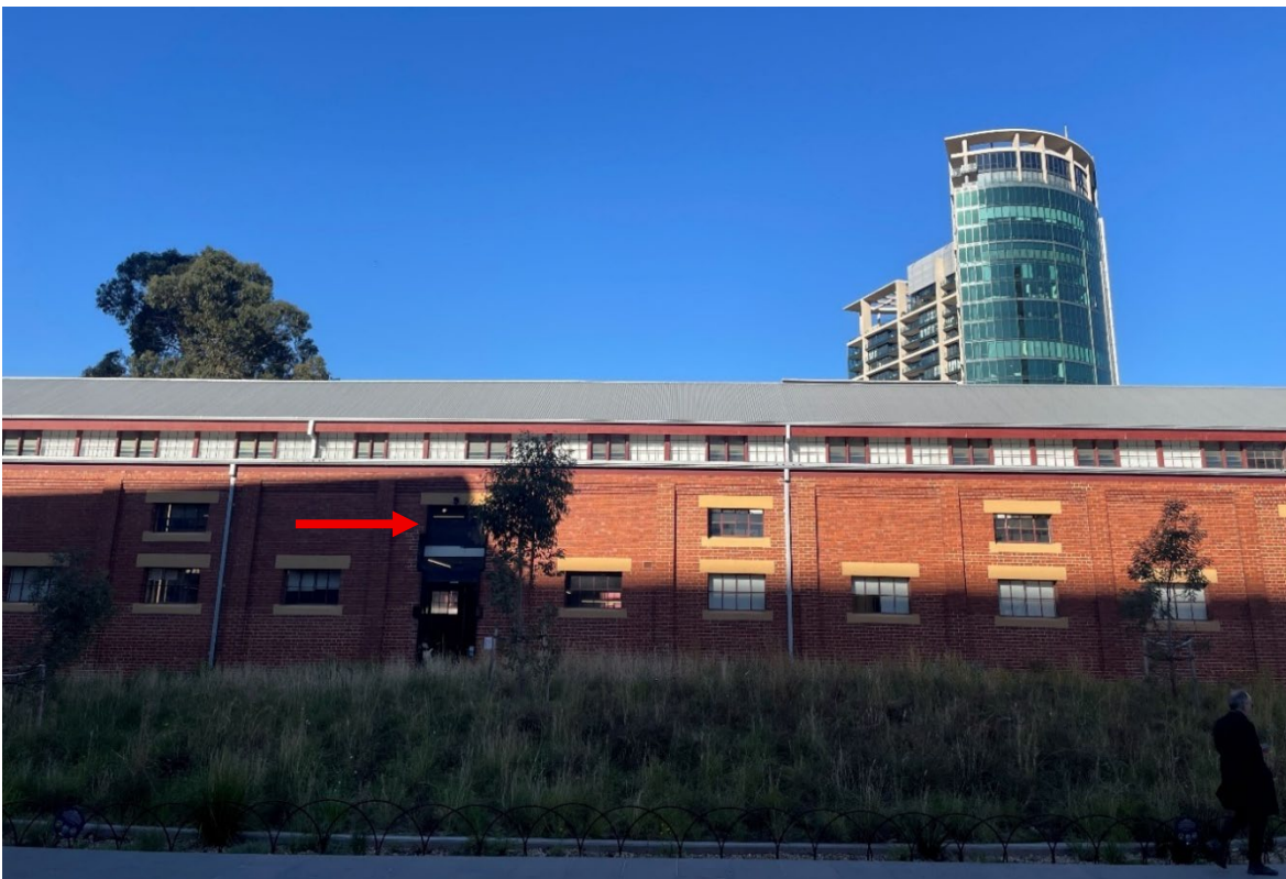
Figure 10 Part west elevation of the stables wing, showing the new galvanised roof to the lantern (clerestory) and introduced entry (indicated)
