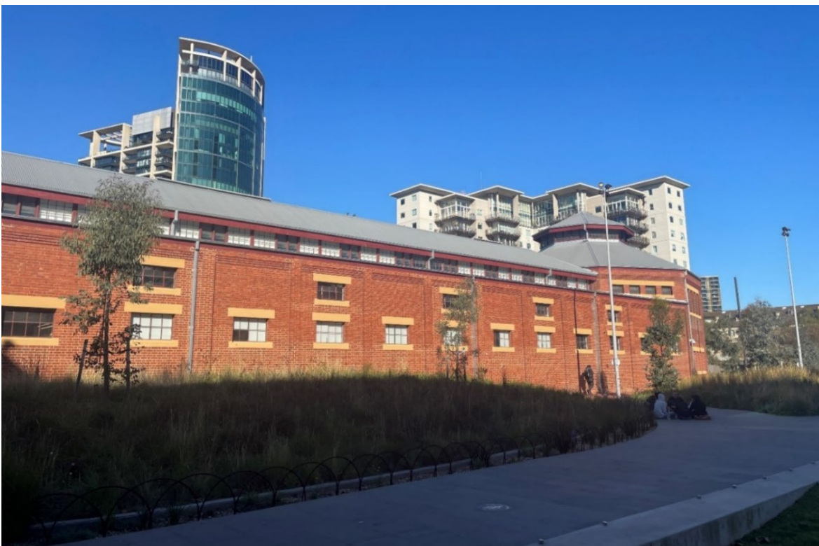
Figure 8 View of the south end of the stables wing (west elevation), with Dodds Street Linear Park in foreground; the octagon is at right
