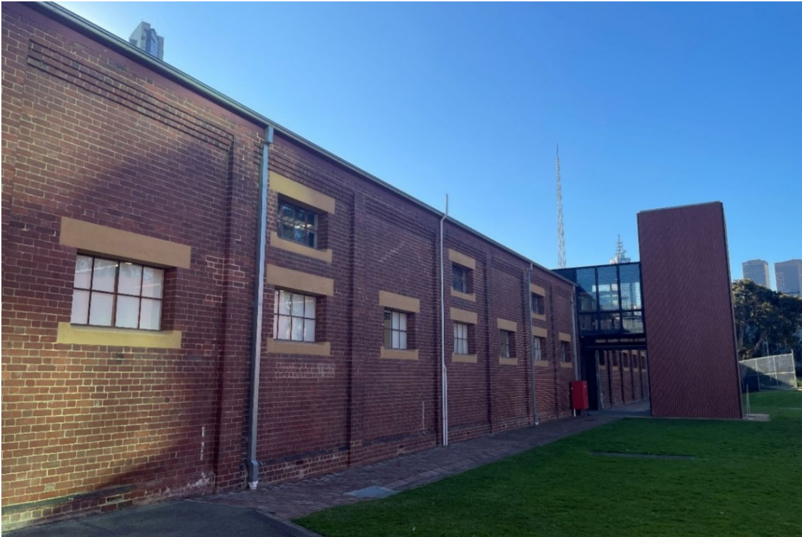
Figure 9 The stables wing (east elevation), with freestanding lift shaft and glazed bridge at right
