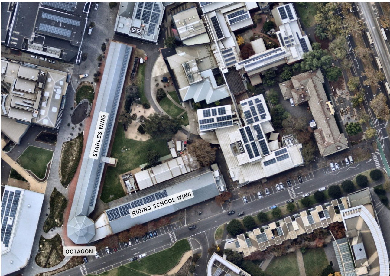
Figure 5 Aerial photograph showing elements of the stables complex Source: Nearmap, 26 May 2025
