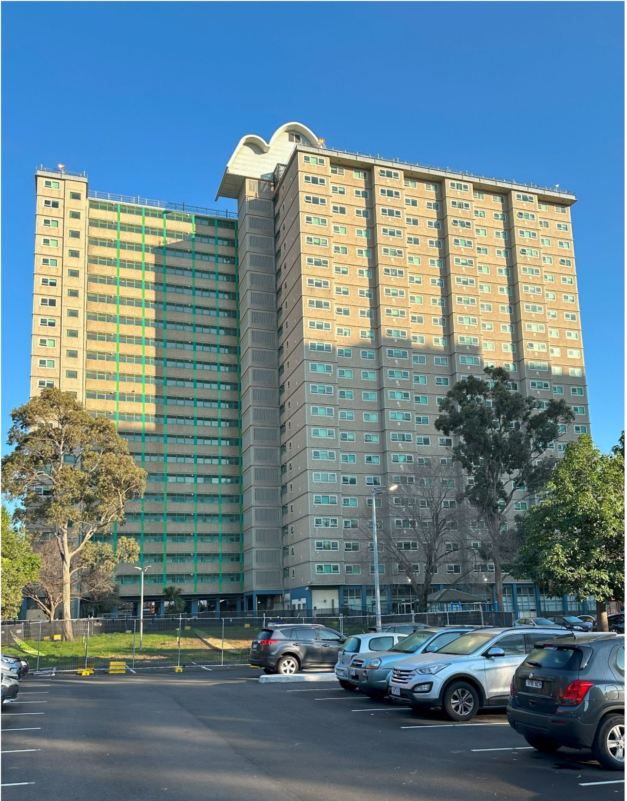
Figure 1 East elevation of 12 Holland Court: the cloud-like addition encloses a lift overrun, part of a programme of works designed by ARM in 1995
