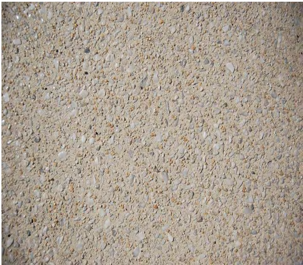
CN01 – CONCRETE PARAPET SNOWSTONE EXPOSED AGGREGATE CONCRETE
