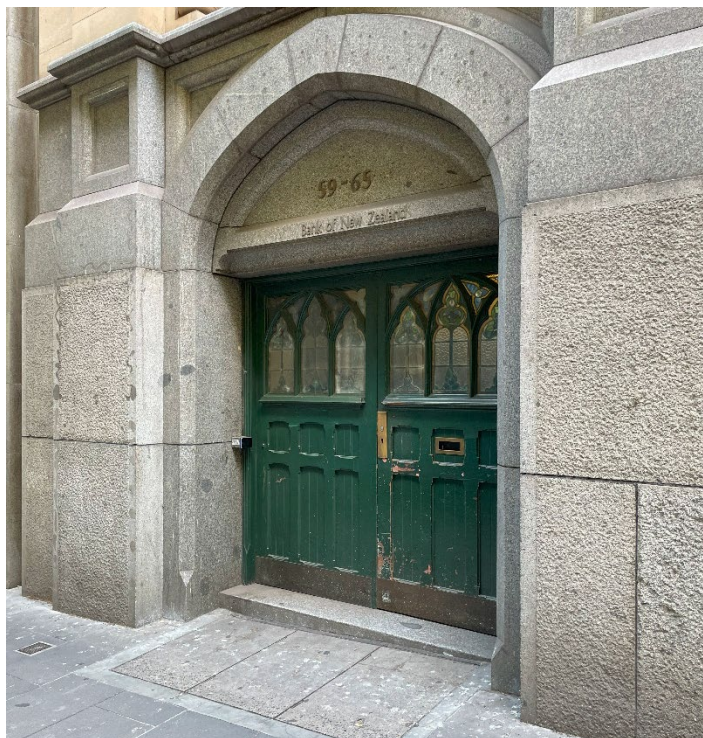
Figure 16 Queen Street entrance, requiring threshold ramp and alteration of swinging doors.
