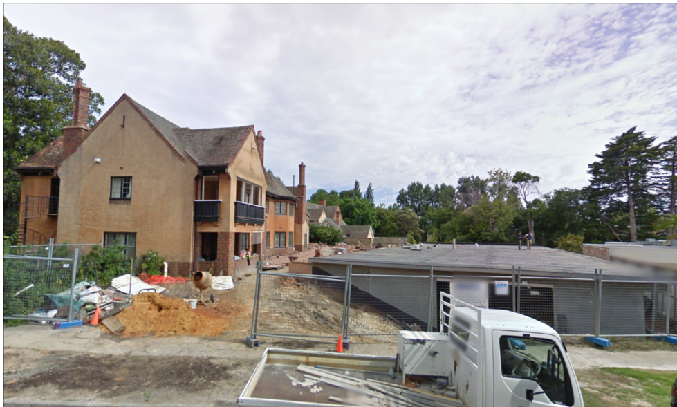
Figure 12 The below ground garage under construction, 2009. Source: Google Street View.
