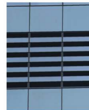
GLA04 - Glass - Tower - Clear Glazing with Louvres/Openings
