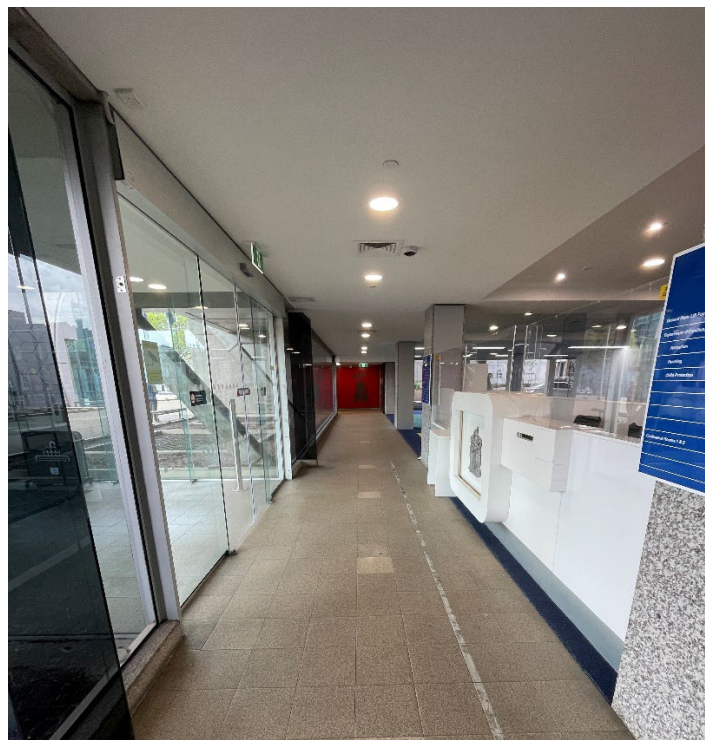
Figure 5 View of the space between the external glass sliding doors and the security desk. Circulation to Lift A in distance.
