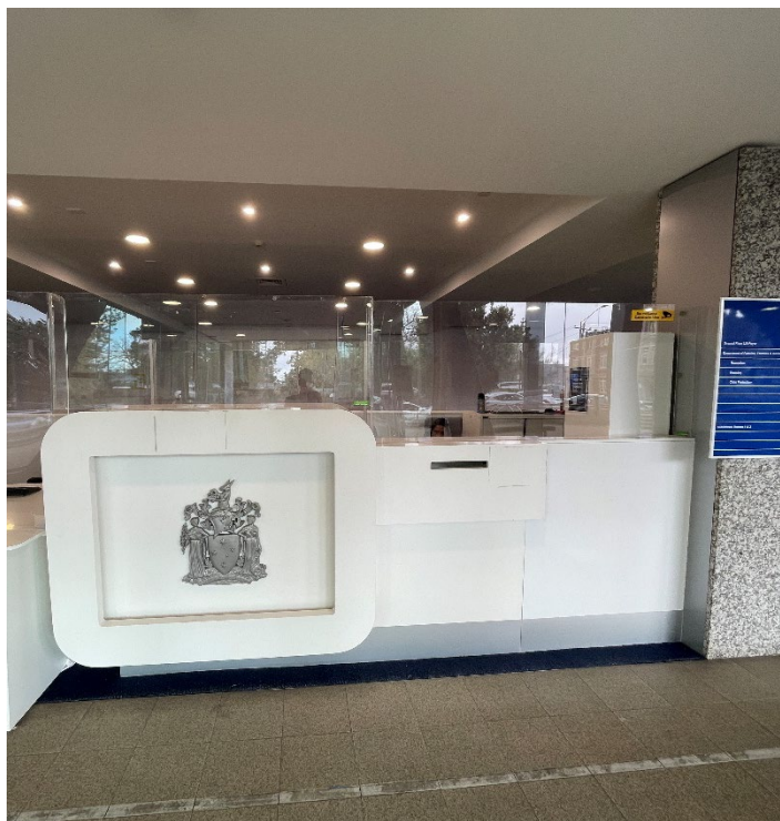
Figure 4 View of the existing security desk from the front entrance.
