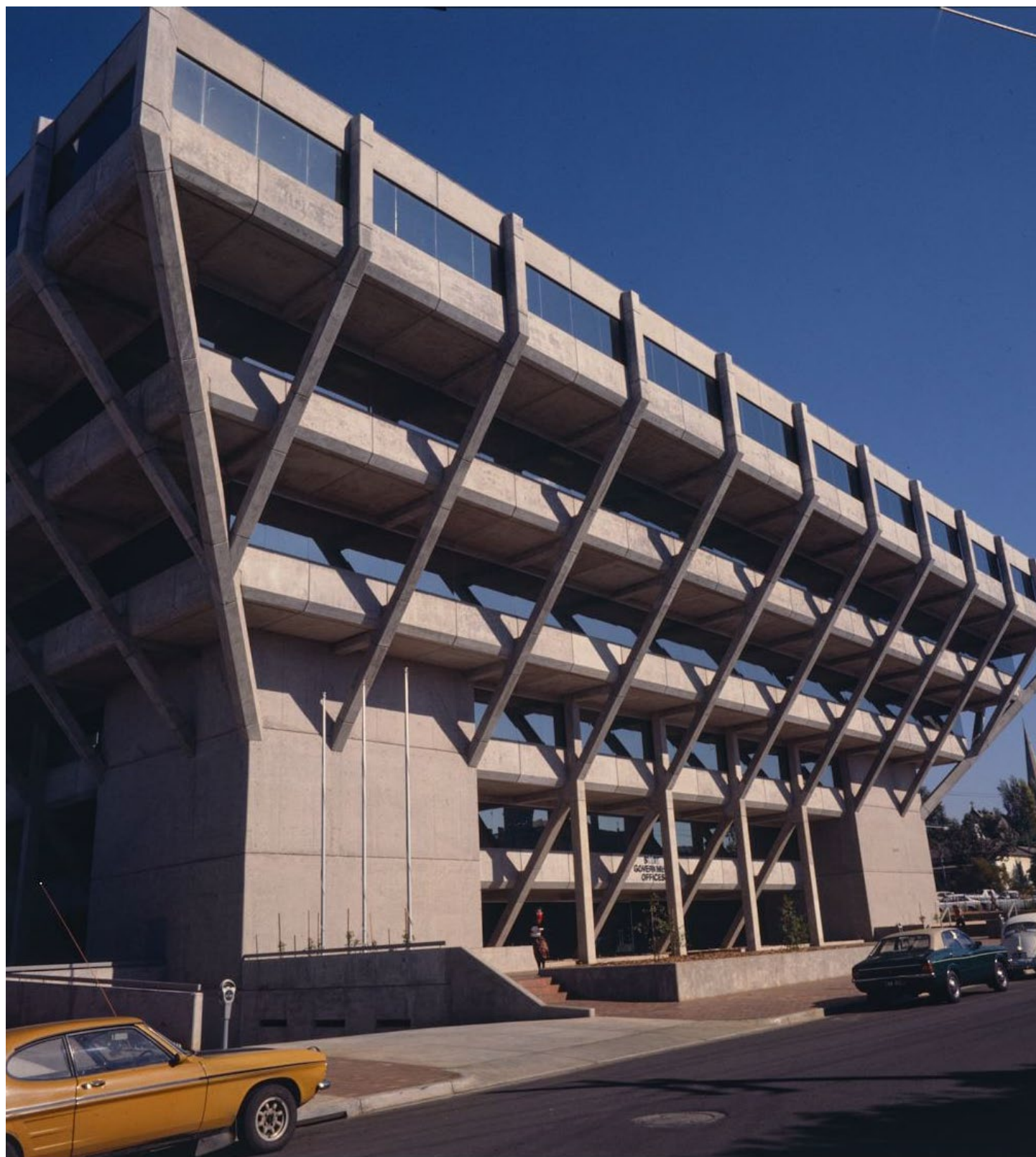
Figure 2 State Government Offices, Geelong, 1979. [Source: National Archives of Australia (NAA: A6135, K11/9/79/5).]
