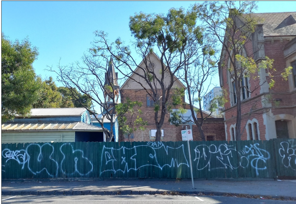
Figure 10 The rear of the church viewed from David Street. The former Model School is partially visible to the right.
