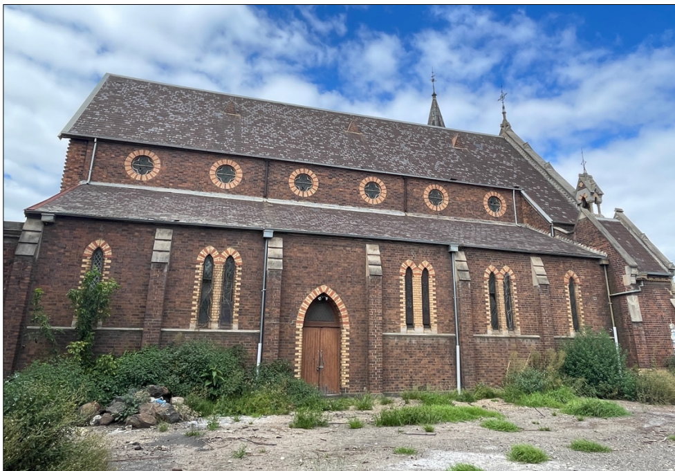
Figure 6 The north elevation.
